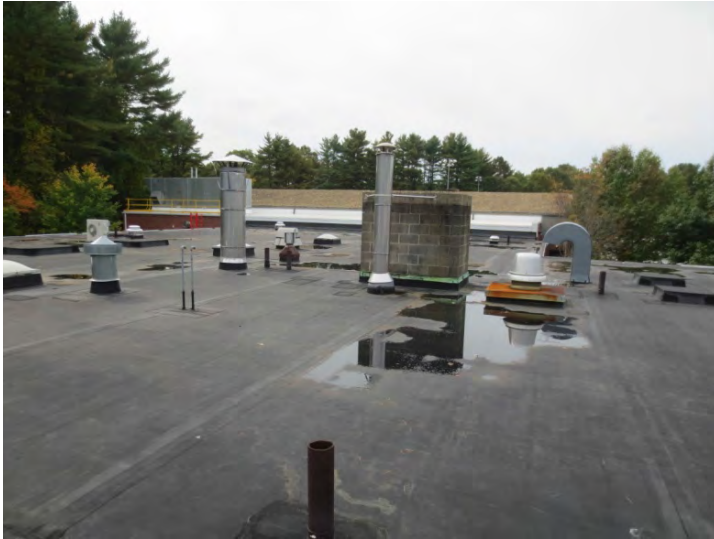
Confirmed Roofing Deficiencies
