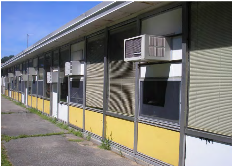
Failed Window Wall of Original School
