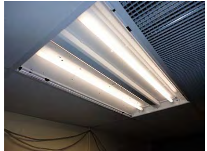
Inefficient Lighting- Lack of Lighting Controls
