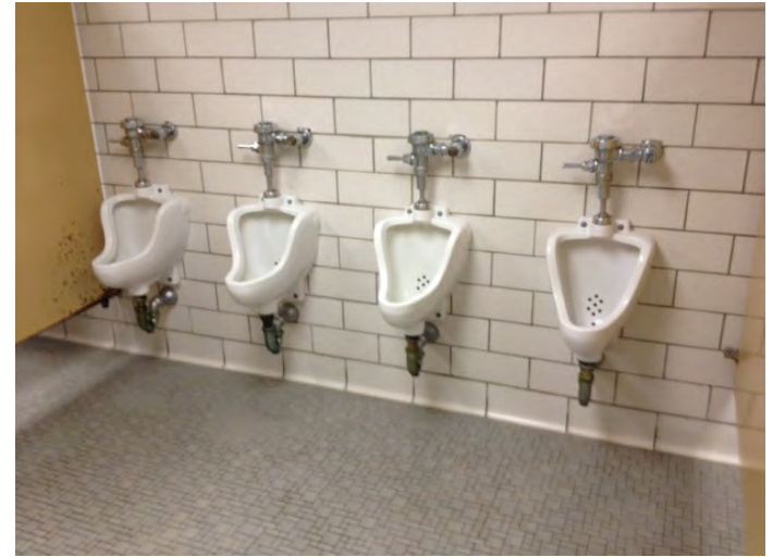
Original 1959 Plumbing Fixtures
