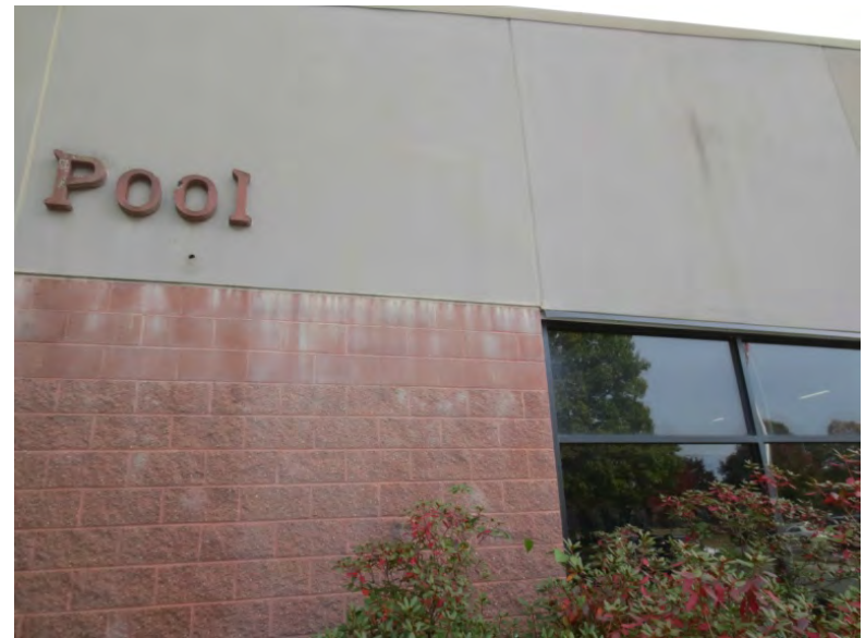
Moisture Issues at Pool Wing
