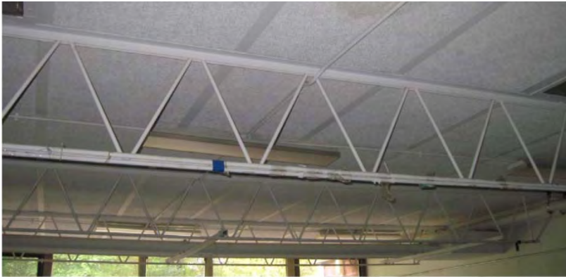
Figure 4-Typical Classroom Framing
