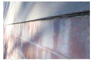
Photo 8 - Failed sealant joint at EIFS panel to veneer CMU below
