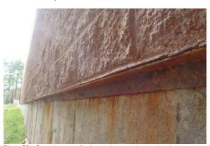
Photo 23 - Corrosion on relieving angle at southeast elevation
