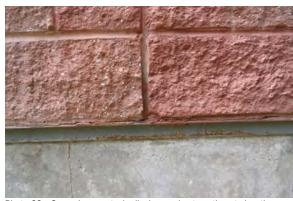
Photo 22 - Corrosion on steel relieving angle at southeast elevation
