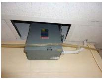
Figure 32 - TV Room Disconnect at Ceiling
