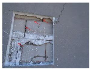
Photo 16 - Cracked CMU joints generally align with crack in EIFS
