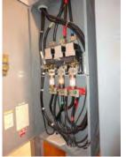
Figure 19 - Disconnect 400 Amp showing burn marks on fuse
