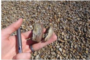
Photo 28 - Degraded roof ballast with sharp edges
