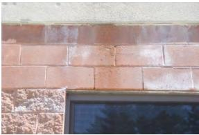
Photo 24 - Scoured CMU below gutter seam
