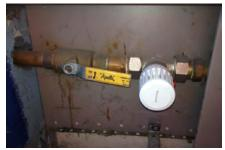
Figure 6 - Replaced Heating Valve
