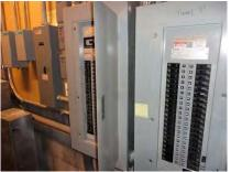
Figure 26 - Branch Panel in Main Electrical Room
