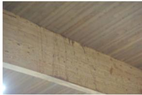
Photo 3 - Staining on the interior laminated wood beams
