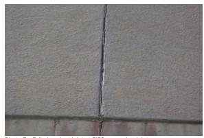
Photo 7 - Failed sealant joint at EIFS expansion joint
