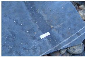
Photo 26 - Water test paper indicating condensation (pink color) on the underside of the EPDM membrane
