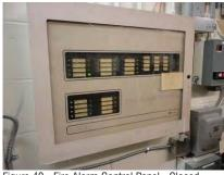
Figure 40 - Fire Alarm Control Panel - Closed
