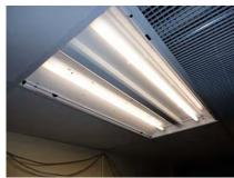
Figure 34 - Troffer with Missing Lens
