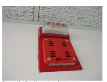
Figure 42 - Fire Alarm Horn Strobe
