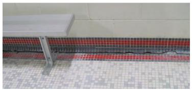
Figure 9 - Slab Settlement Near Diving Pool
