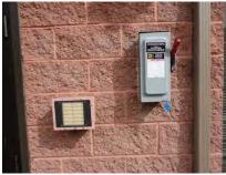
Figure 25 - PV System Utility Disconnect and Fire Alarm Remote Annunciator
