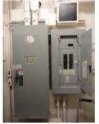
Figure 22 - Automatic Transfer Switch and Emergency Panel
