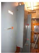
Figure 18 - Main Switchgear (two disconnects and one main breaker)
