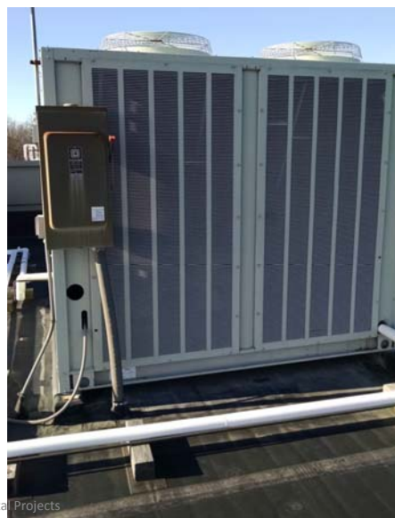
Existing R22 Refrigerant AC Condensing Unit Typical for Curtis and Loring
