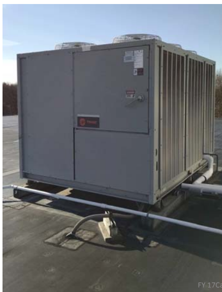
Existing R22 Refrigerant AC Condensing Unit Typical for Curtis and Loring
