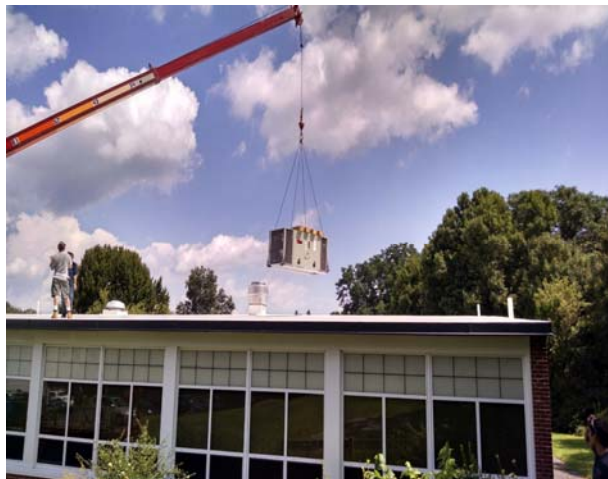
This is the Noyes rooftop unit replaced in 2015
