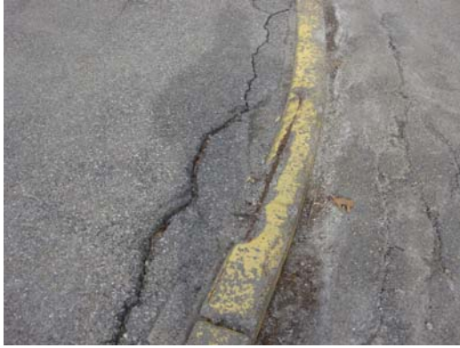
Rebar is exposed in concrete curbs
