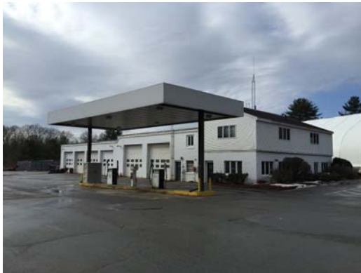
DPW fuel filling station
