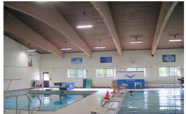
Figure 10 - Typical Roof Framing at Atkinson Pool
