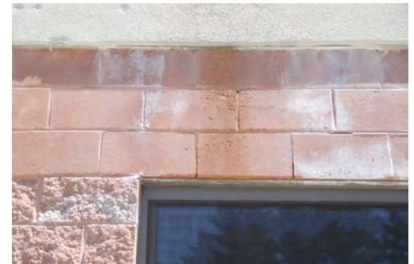
Photo 24 - Scoured CMU below gutter seam
