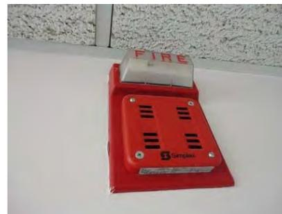
Figure 42 - Fire Alarm Horn Strobe
