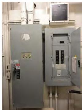
Figure 22 - Automatic Transfer Switch and Emergency Panel
