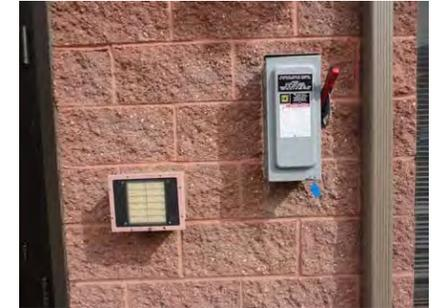
Figure 25 - PV System Utility Disconnect and Fire Alarm Remote Annunciator
