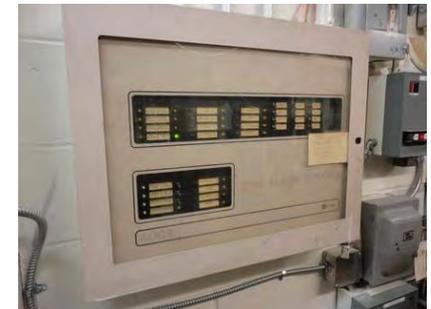
Figure 40 - Fire Alarm Control Panel - Closed
