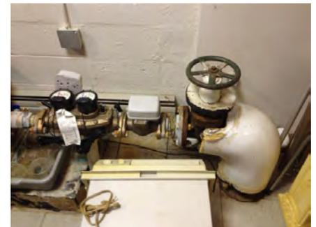
Figure 11 - Water Service Leak
