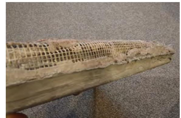
Photo 12 - EIFS base coat does not wrap around the board edges at the base of the system
