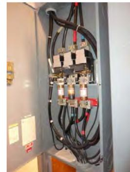
Figure 19 - Disconnect 400 Amp showing burn marks on fuse
