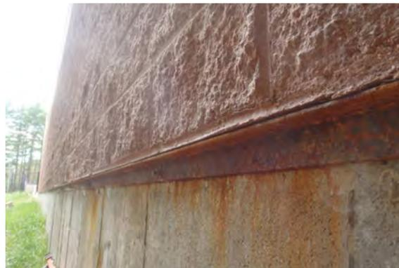
Photo 23 - Corrosion on relieving angle at southeast elevation
