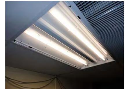
Figure 34 - Troffer with Missing Lens
