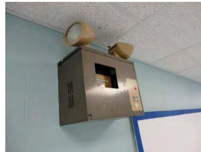
Figure 39 - Emergency Lighting Unit in Corridor
