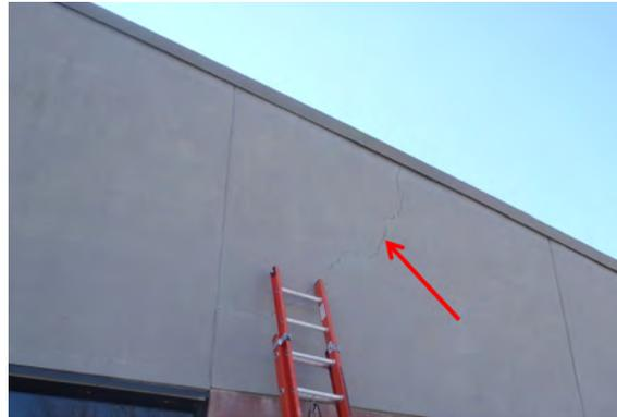
Photo 4 - Crack at the northwest elevation
