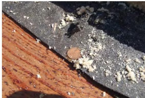
Photo 27 - Surface corrosion on fastener securing asphalt-impregnated felt to wood deck
