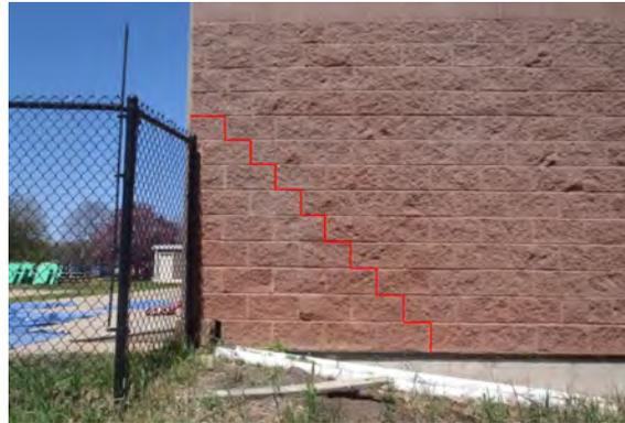
Photo 19 - Cracking at the south corner of the building
