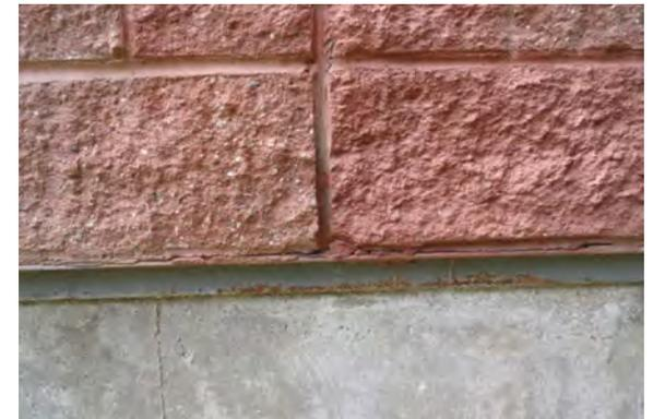
Photo 22 - Corrosion on steel relieving angle at southeast elevation
