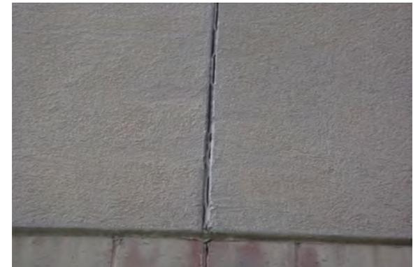
Photo 7 - Failed sealant joint at EIFS expansion joint
