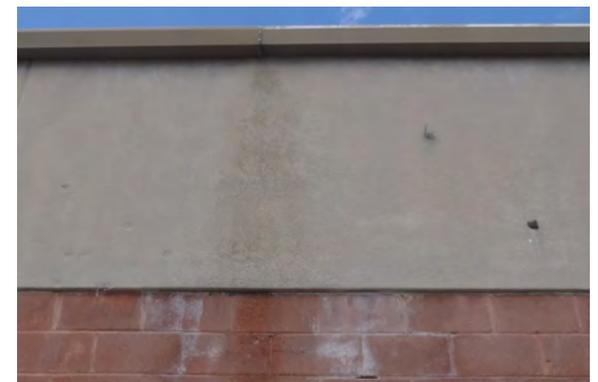
Photo 9 - Scoured EIFS and CMU below leaking gutter joint
