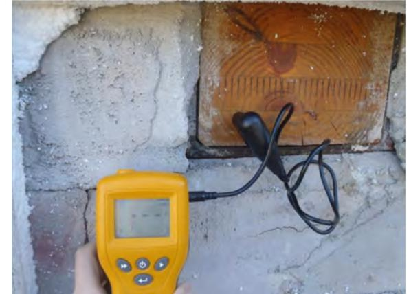
Photo 15 - Wood beam exposed behind EIFS
