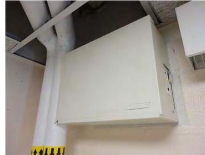
Figure 37 - Emergency Lighting Battery / Inverter
