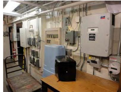
Figure 24 - PV System Inverter
