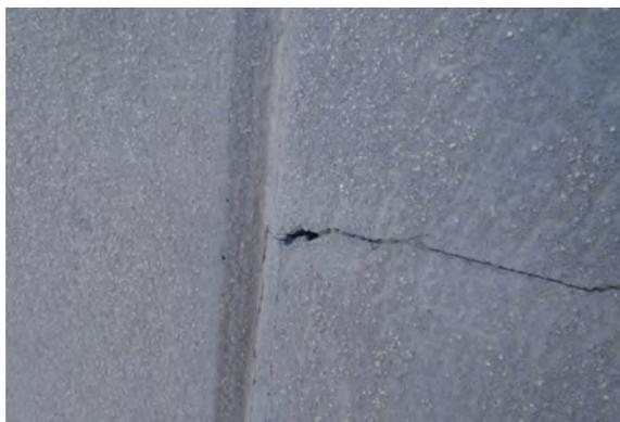
Photo 10 - Reveal in EIFS system cracked at the northwest elevation
