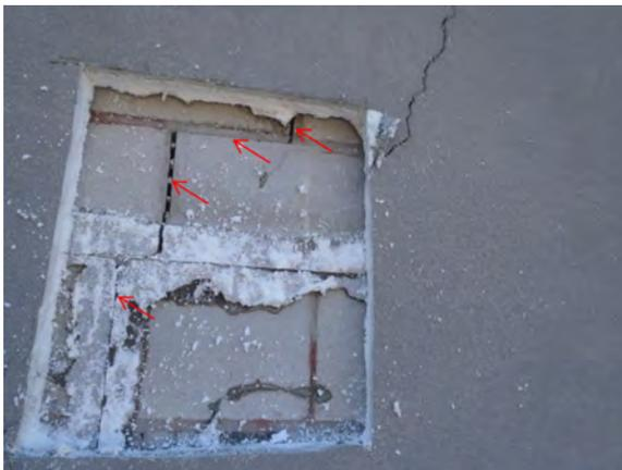
Photo 16 - Cracked CMU joints generally align with crack in EIFS
