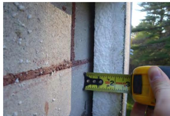
Photo 11 - EIFS insulation board spaced approx. 1/2 in off CMU backup
