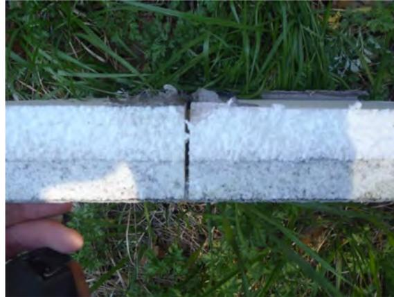
Photo 14 - Insulation Boards are spaced approximately 1/8 in.
