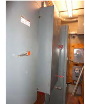
Figure 18 - Main Switchgear (two disconnects and one main breaker)
