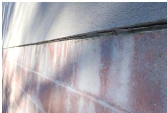
Photo 8 - Failed sealant joint at EIFS panel to veneer CMU below
