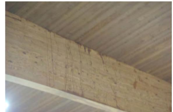
Photo 3 - Staining on the interior laminated wood beams
