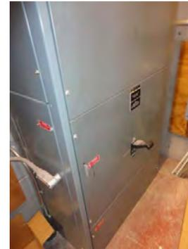
Figure 16 - 800 Amp Main Breaker Switchgear
