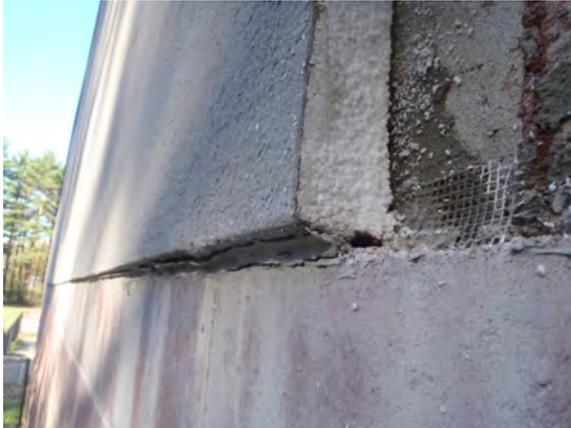
Photo 13 - Failed sealant at the EIFS to CMU veneer joint
