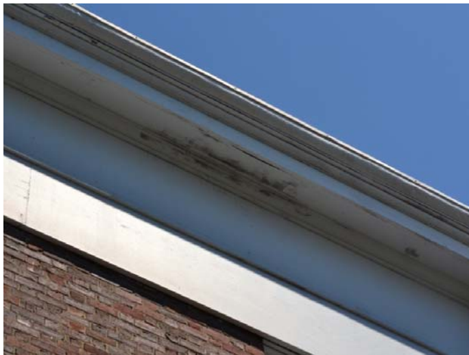
Deteriorating wood soffit
