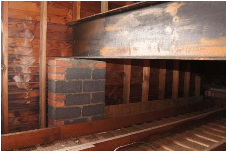
Steel beam in attic supported on brick and cinder block pier.
