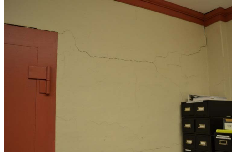
Plaster cracking at first floor vault wall.
