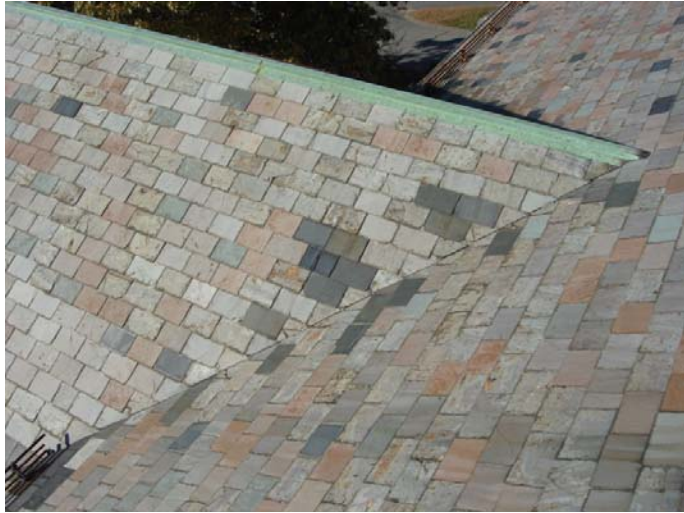
Slate, flashings and snow guards in fair to poor condition
