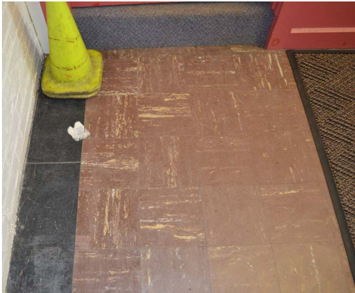
Possible asbestos tile in Town Clerk lobby and north and south wing stair halls
