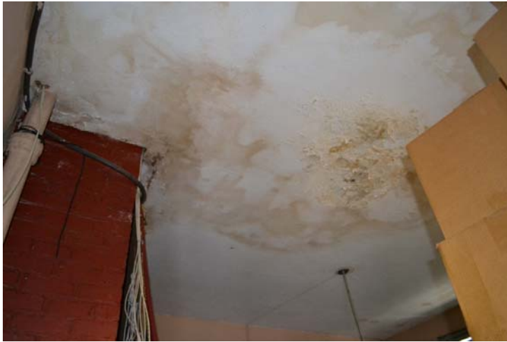
Water damage at ceiling on stage level.
