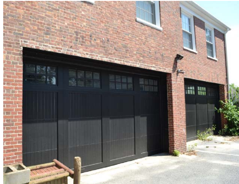
Failing masonry opening at Fire Station doors
