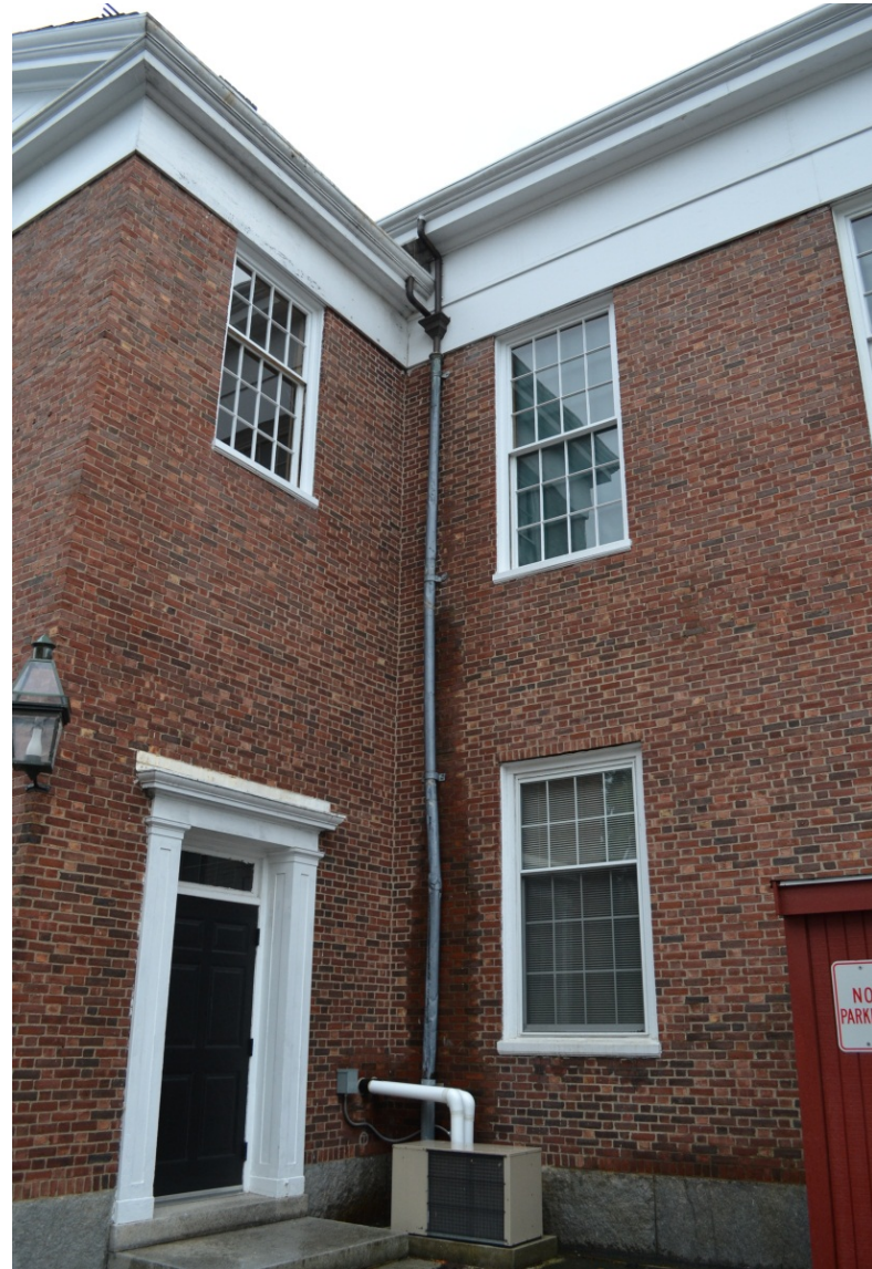
Leaking gutters and rain leaders
