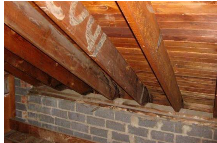
Rafters not tied to masonry walls
