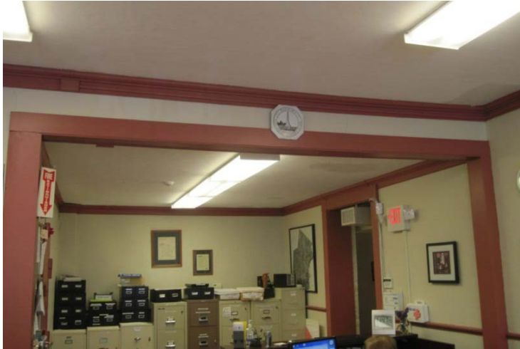
The support beam at the Town Clerk ceiling is sagging.
