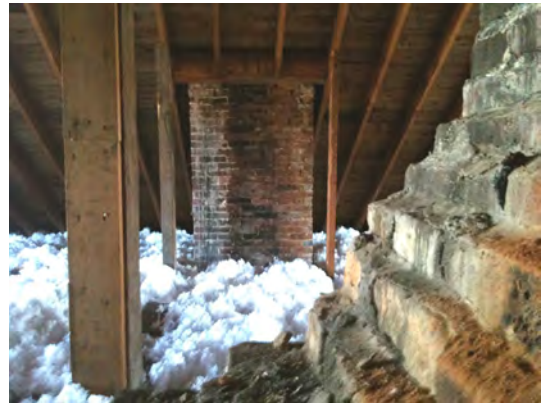
Loose fill insulation between ceiling joists.
