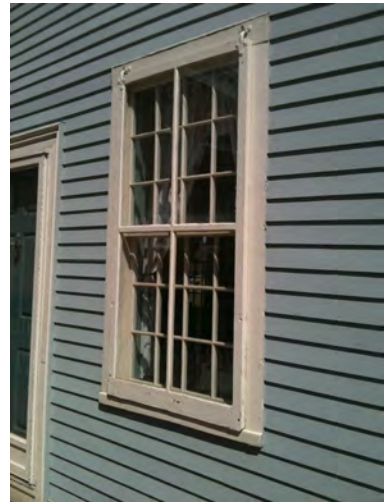
2-over-2 storm window in place over 12-over-12 window.
