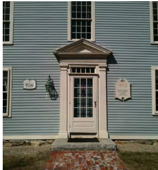
Pedimented door surround with pilasters, transom, and dentilled cornice and entablature.
