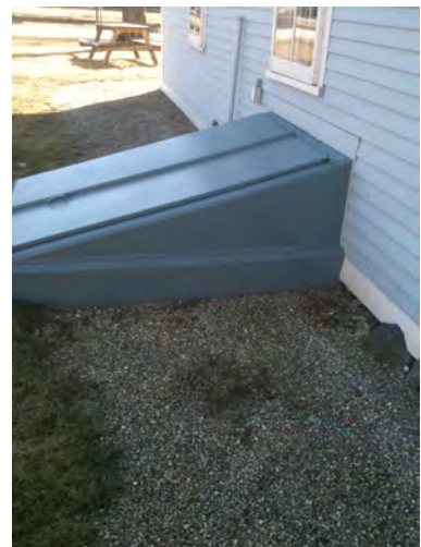
Bulkhead at north elevation.
