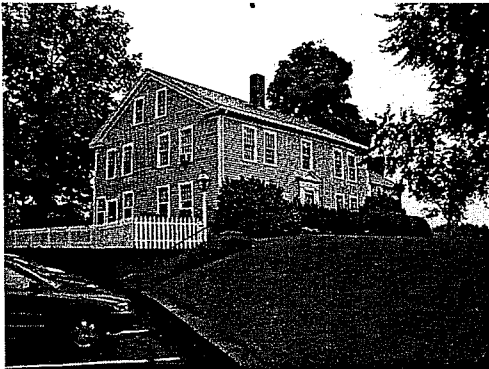
Parking lot for the Parsonage. Note stairs to reach main entry.
