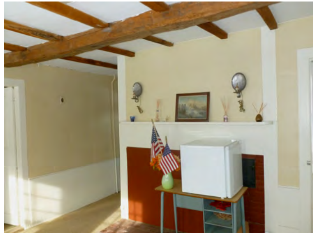
Wainscot of wide horizontal boards. Framing elements at ceiling.
