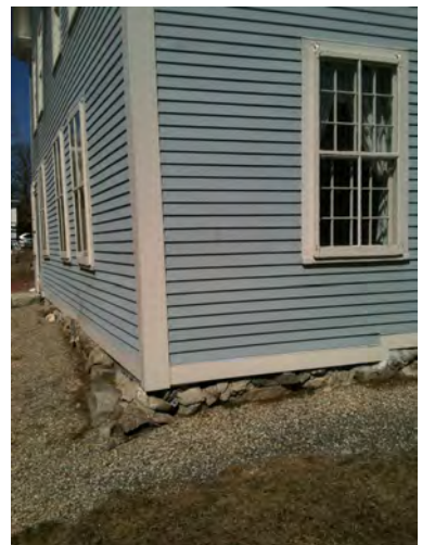
Note wood storms on the windows and rubble stone foundation.
