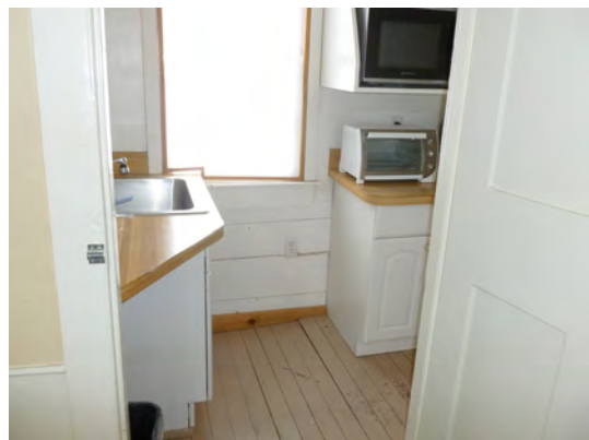
Narrow strip floor in the kitchen. Note horizontal plank dado.
