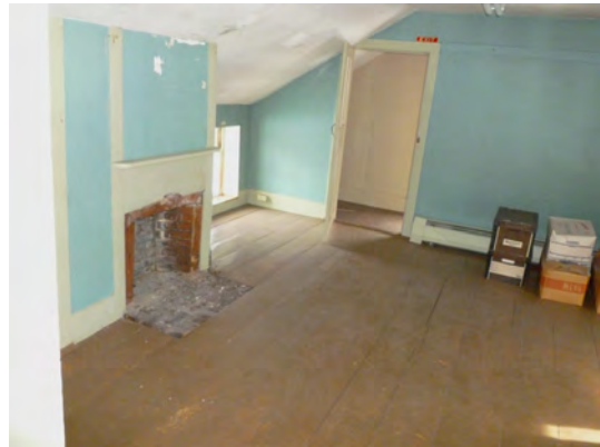
Wide plank flooring and open fireplace in ell storage room.
