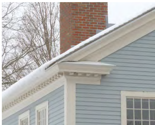
Greek Revival cornice return at gable end. Note dentils.
