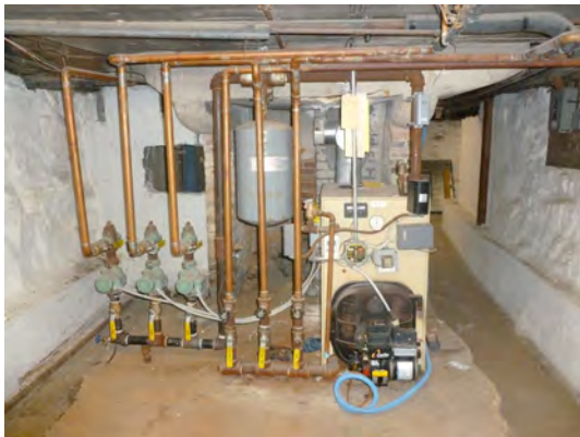
Note concrete haunch at the foot of the whitewashed rubble walls.
