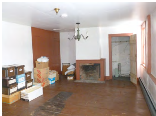
Wide plank flooring and open fireplace in northeast room.
