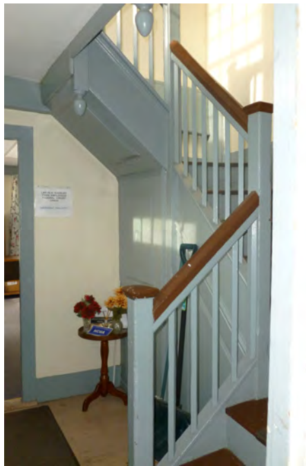
Stair hall. Note pendant details.
