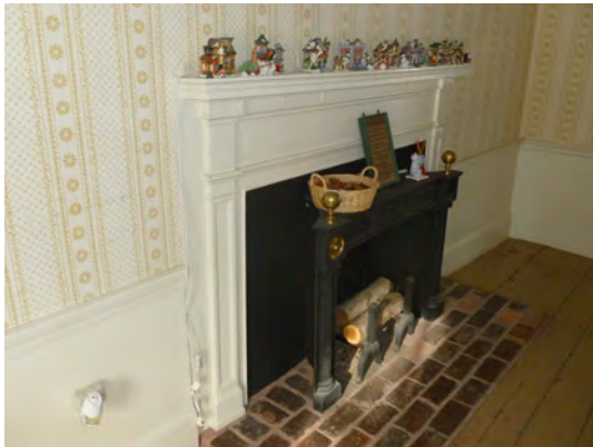
The plaster walls in the parlor have been papered. Note the Federal era fireplace insert.
