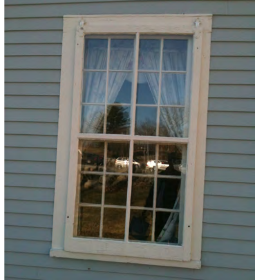
12-over-12 light sash with 2-over-2 wood storm window.
