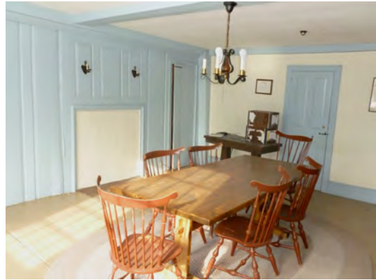
Paneled wall, boxed framing and wide plank flooring in southeast room. Fireplace has been closed in.
