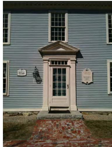
Main entry with pedimented surround.
