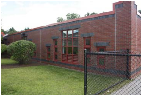
Fig. 2-39 TYPICAL MASONRY CONTROL JOINT & WINDOW OPENINGS AT 1990 & 1994
