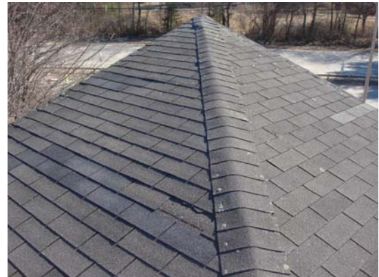
Fig. 2-09 SLOPED CENTER RIDGE WITH AREA OF PREVIOUS SHINGLE REPAIR
