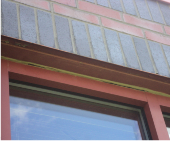
Fig. 2-45 LINTEL ABOVE WINDOW OPENINGS AT 1990 CONSTRUCTION, PEELING PAINT AND SEPARATED CAULKING ARE EVIDENT
