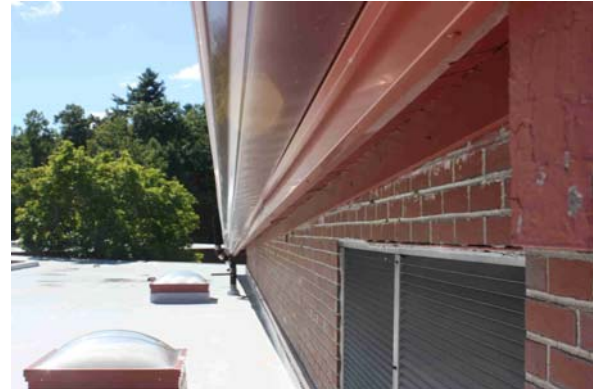
Fig. 2-46 LOUVER AT THE BACKSIDE OF THE CAFETORIUM – PERIMETER CAULKING TO BE ABATED & REPLACED
