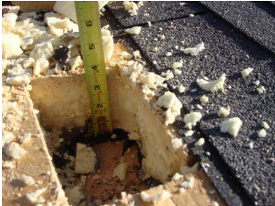
Fig. 2-07 ROOF CUT SHOWING TOP OF WOOD DECK, VAPOR BARRIER, INSULATION, NAILER BOARD, UNDERLAYMENT & SHINGLES
