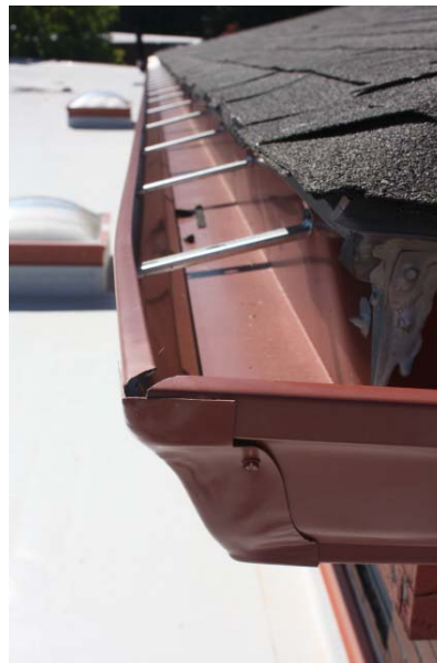
Fig. 2-14 TYPICAL GUTTER AT SLOPED SHINGLE ROOF
