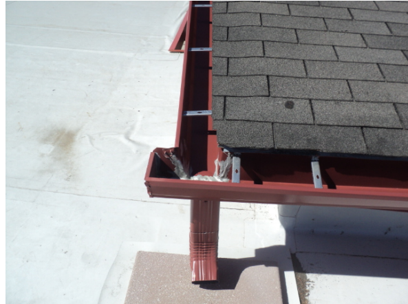
Fig. 2-13 DOWNSPOUT TO SPLASHBLOCK ON FLAT ROOF- NORTHEAST CORNER
