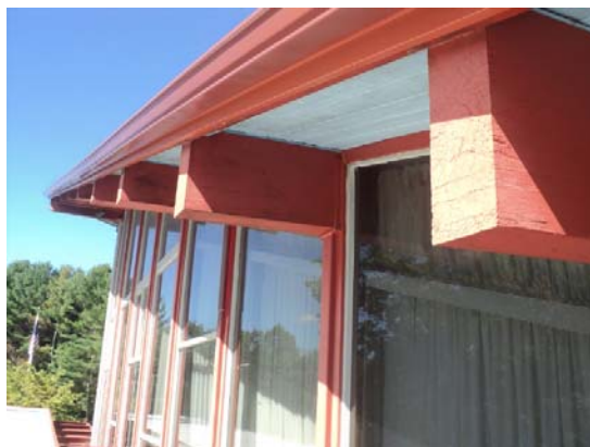
Fig. 2-06 CAFETORIUM OVERHANGING SOFFIT WITH EXPOSED WOOD DECK AND GLU-LAM BEAMS
