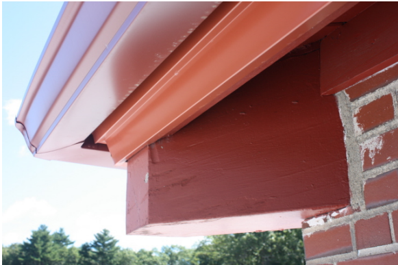
Fig. 2-11 TYPICAL GUTTER, FASCIA & MAIN GIRDER – NORTHEAST CORNER
