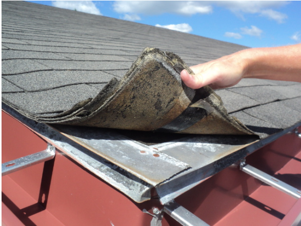
Fig. 2-10 DRIP EDGE CONDITION
