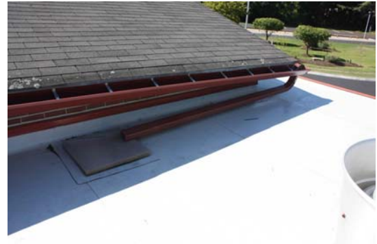
Fig. 2-15 DOWNSPOUT TO SPLASHBLOCK SET ON FLAT ROOF- NORTHWEST CORNER
