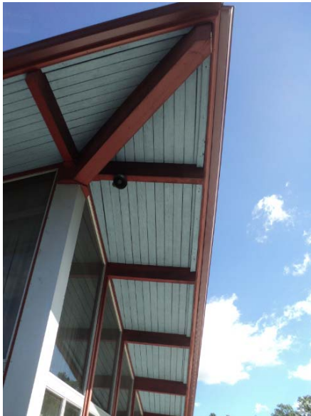
Fig. 2-16 CAFETORIUM SOFFIT WITH EXPOSED WOOD DECK AND GLU-LAM BEAMS AT SOUTHWEST CORNER
