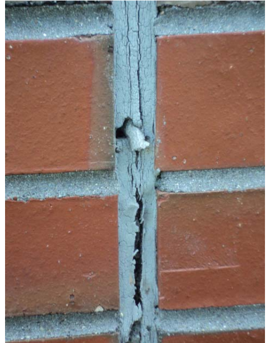
Fig. 2-40 MASONRY CONTROL JOINT, 1990 CONSTRUCTION
