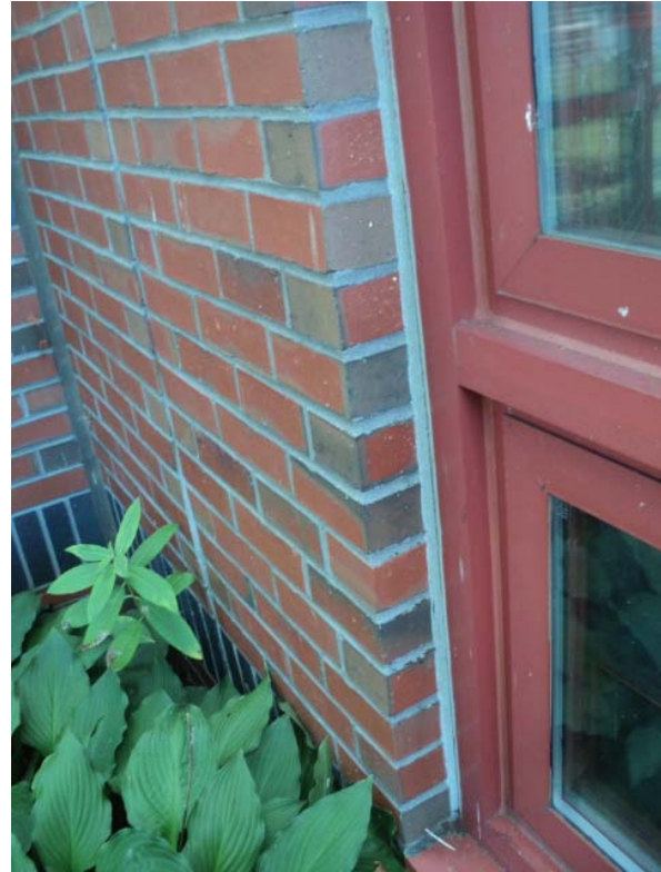
Fig. 2-44 WINDOW PERIMETER JOINT & METAL-TO-METAL JOINT OPERABLE SASH TO FRAME, 1990 BUILDING
