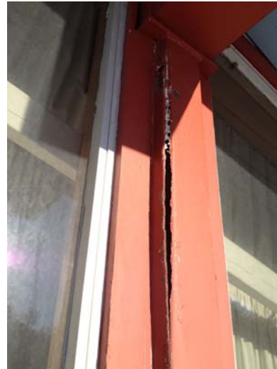
Fig. 2-22 DAMAGED COLUMN PRIOR TO REPAIR
