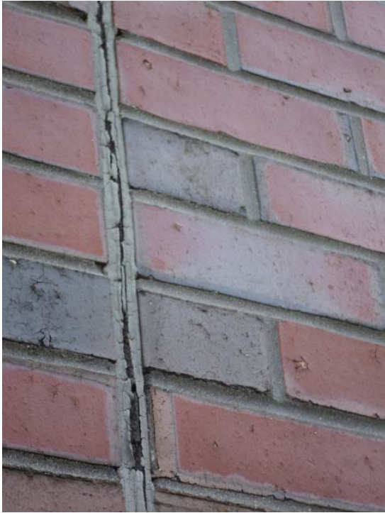
Fig. 2-42 MASONRY CONTROL JOINT, 1990 CONSTRUCTION
