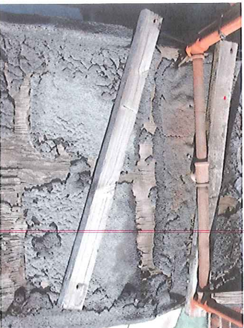
ROTTED DECKING & ROOF OF PLATFORM @ RIGE
