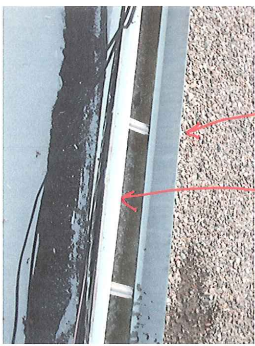
EDGE FLASH & GUTTER @ REAR ENTRY
