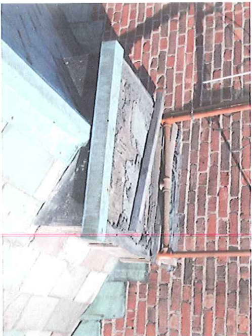
ROTTED DECKING & ROOF OF PLATFORM @ RIGE
