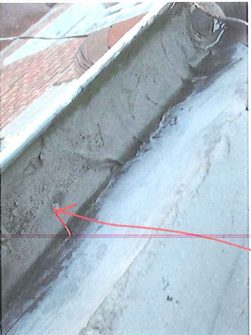
COPPER GUTTER LINED W/ TAR
