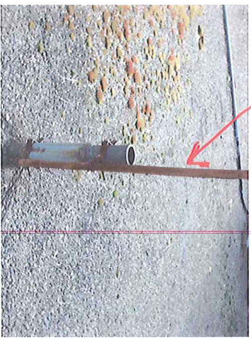
COPPER FLASHED SOIL PIPE W/ANTENNA POLE
