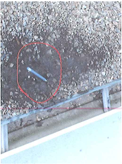
COPPER FLASHED SOIL PIPE W/ANTENNA POLE
