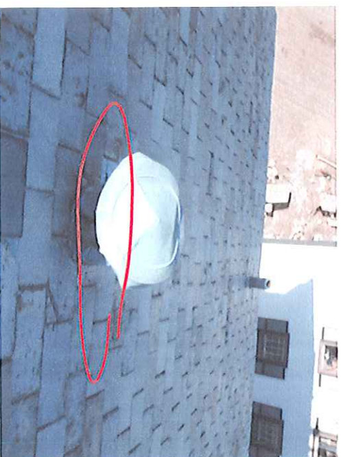
10" STACK DAMAGED
