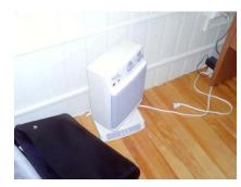
Some of the office workers are uncomfortably cold in the winter. In order to maintain comfort, they use electric space heaters. Electric heat is expensive. It would be more cost effective to use the central hot water loop to provide additional heating to cold spaces in the building.
