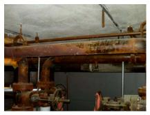
Hot water piping in the area around the boiler was observed to be missing insulation. These pipes are in semi-unconditioned spaces. Most of the heat that is dissipated through these uninsulated pipes will not contribute to building heat.
