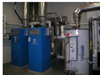
Fig. 6-1 A new boiler plant was installed in 2003.
