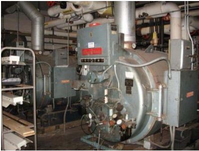
Existing Cleaver-Brooks Boilers
