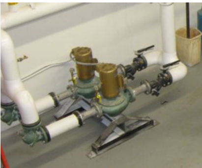
Hot Water Circulating Pumps
