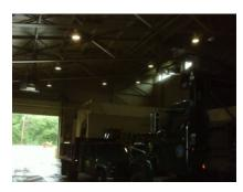
The metal equipment storage high bay space attached to the DPW Office Building is currently lit with twenty-four (24) 400-watt metal halide units. We estimate that the lights are on at least 2,500-hours per year.
