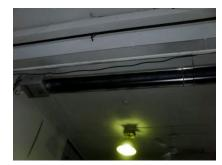
One maintenance bay is currently lit with six (24) 400-watt metal halide units. We estimate that the lights are on at least 2,500-hours per year.
