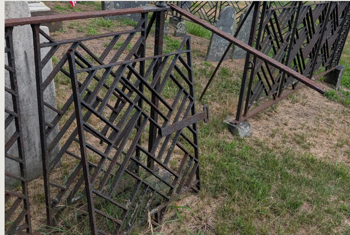
Plympton plot — enclosure off its posts and leaning on the stones
