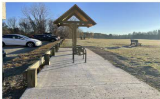
Photo 3: Field entrance area.
