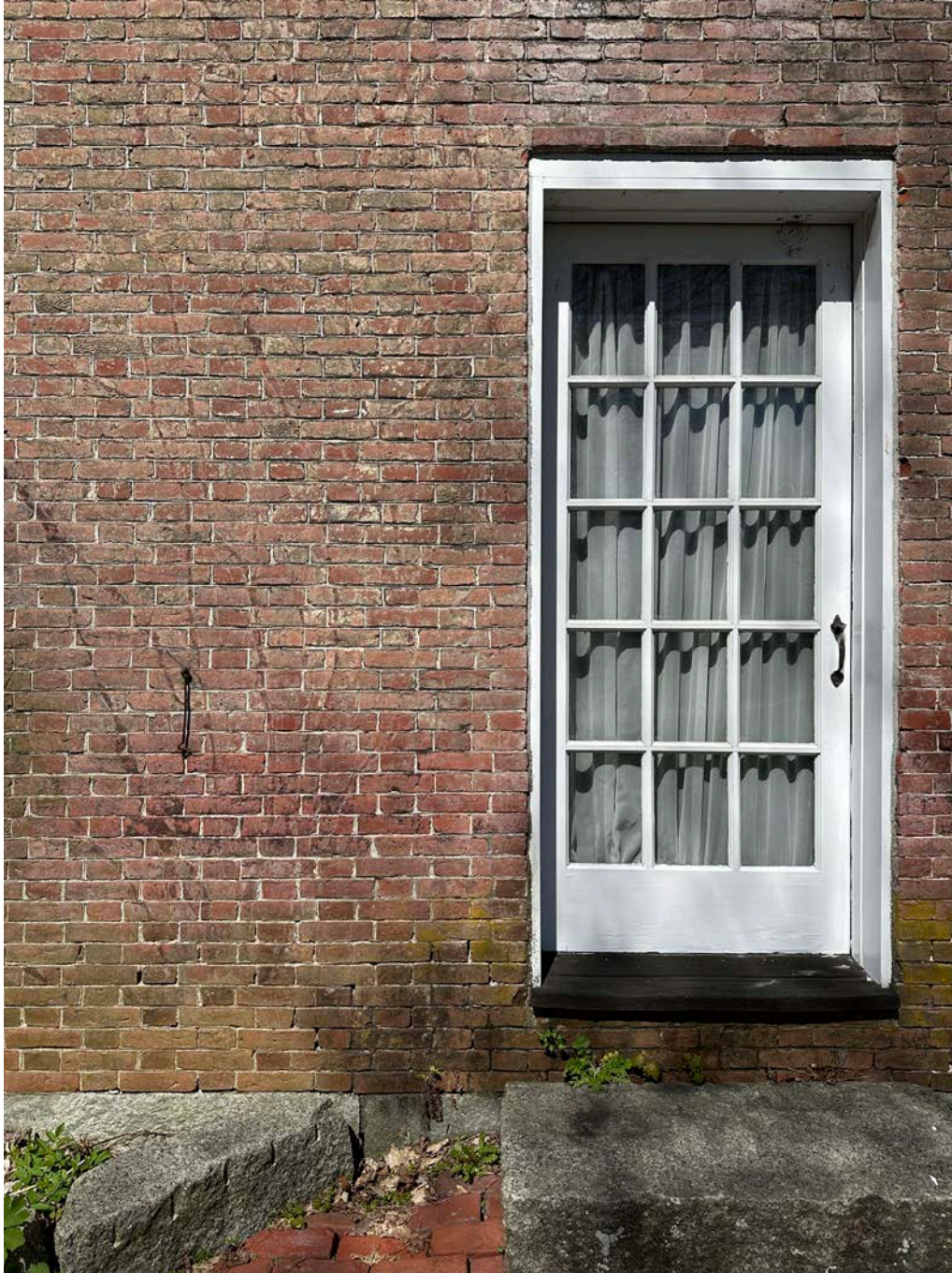
Figure 4.4-5 D-06 is a new tempered glass door.
