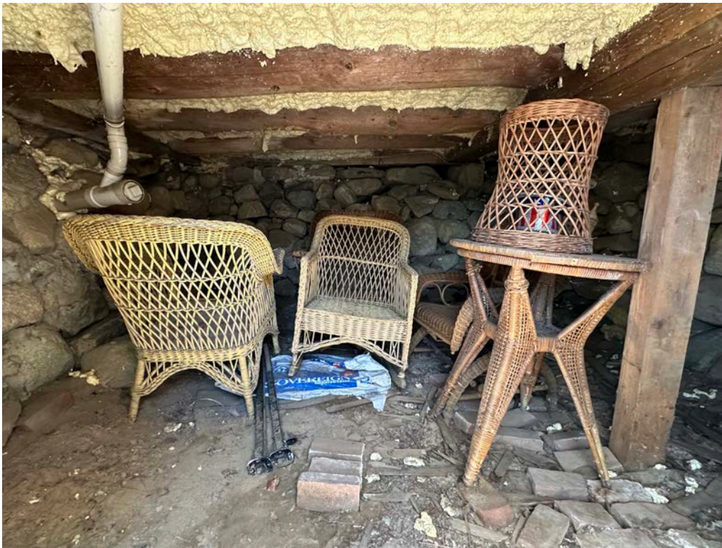
Figure 4.3-10 There is one crawl space (room B-02) directly below room F-05, which is accessed from outside with no access to the basement, and is also constructed of both ashlar and loose laid stone masonry.
