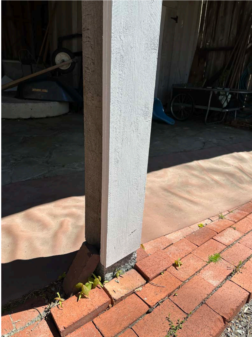
Figure 4.1-9 Refaced and re finished carriage house column.
