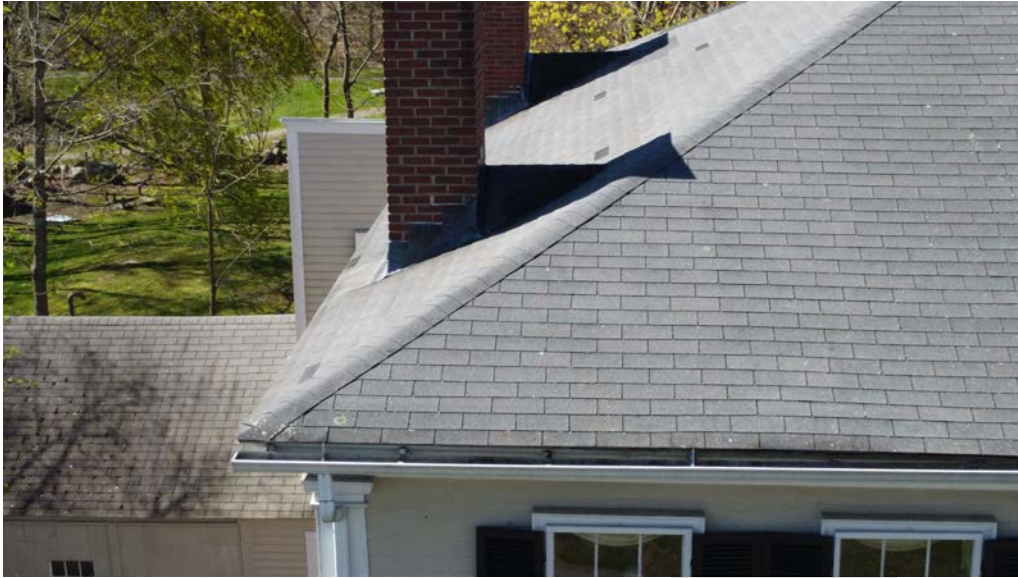
Figure 4.8-4 It seems that to avoid fastening the gutter to the detailed fascia, small blocks cut to match the profile of the fascia were installed at evenly spaced intervals and protrude out just past the roof edge.
