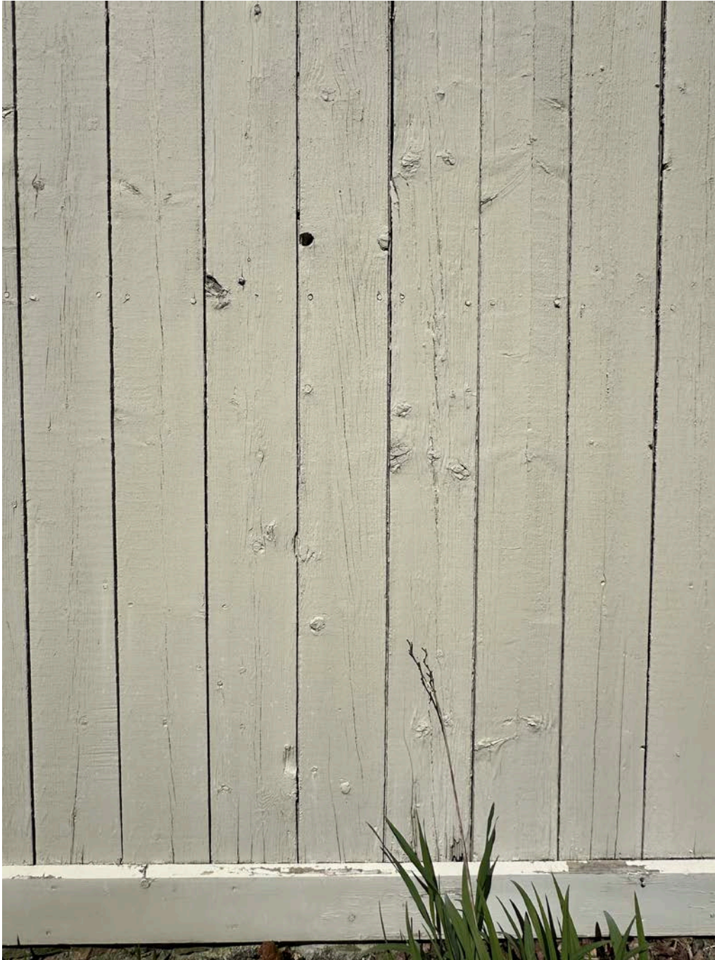
Figure 4.1-7 Vertical planks of carriage house with an average exposure of 6-1/2 inches.
