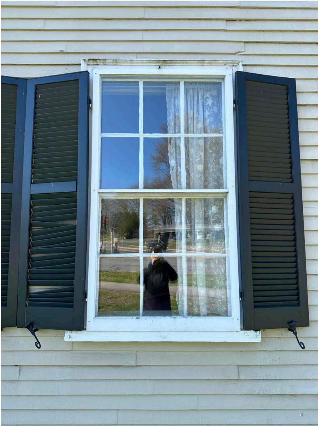
Figure 4.4-1 Double-hung six-over-six lite window configuration found typically on the main house.
