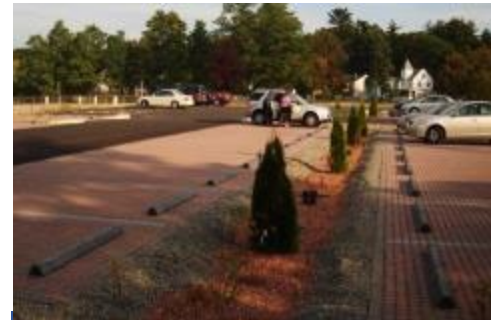
Silver Lake (Wilmington, Massachusetts) LID Demonstration Project
