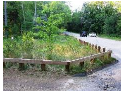
Bioretention cell constructed as part of watershed-based plan BMP recommendations.
