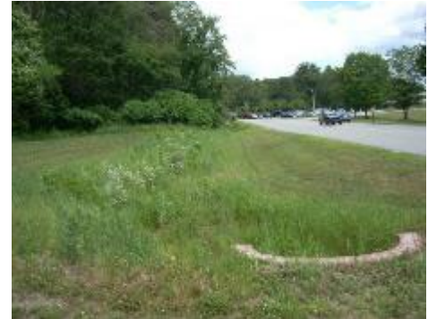
Bioretention cell installed as part of a grant implementation project.
