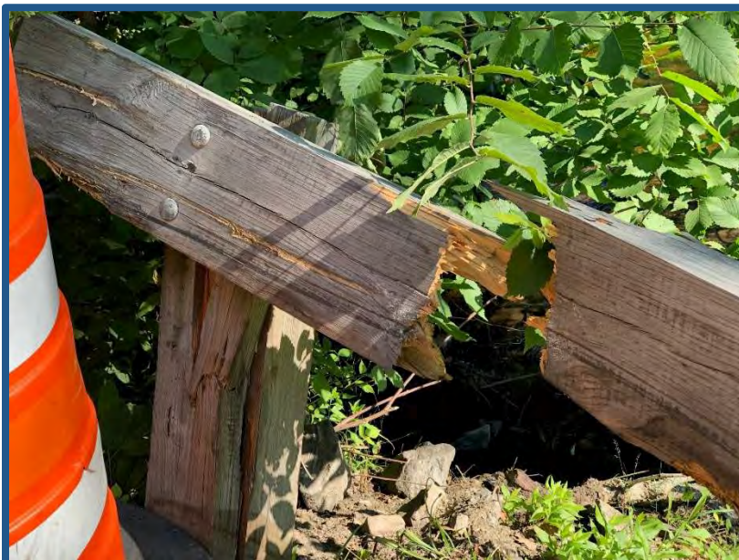
Broken sections of wood guardrail
