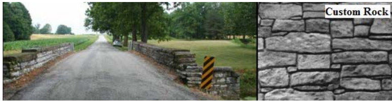
(a) Railing Detail (b) Formliner: "New England Drystack" Figure 4.14 – Stone 2 railing
