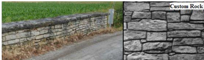
(a) Railing Detail (b) Formliner: "New England Drystack" Figure 4.15 – Stone 3 railing
