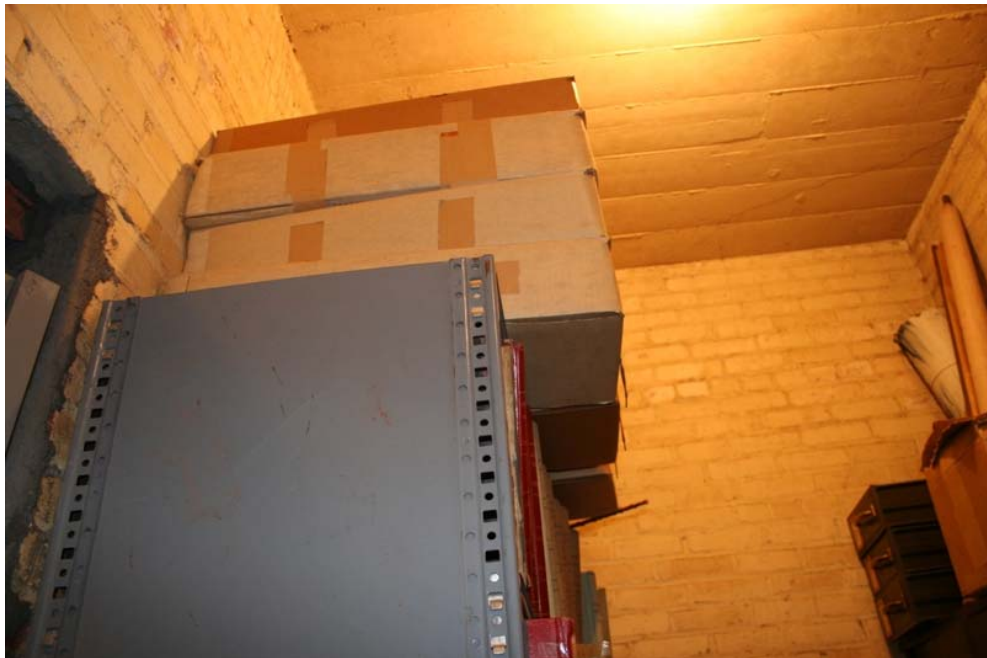
Figure 4. Boxes are stacked on top of a shelving unit in the basement vault for lack of anywhere else to put them. They are very difficult to access and could easily topple if the stack were to become unbalanced.
