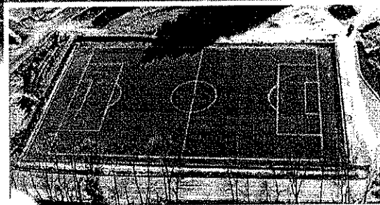
Cutting Field during construction - 2005
