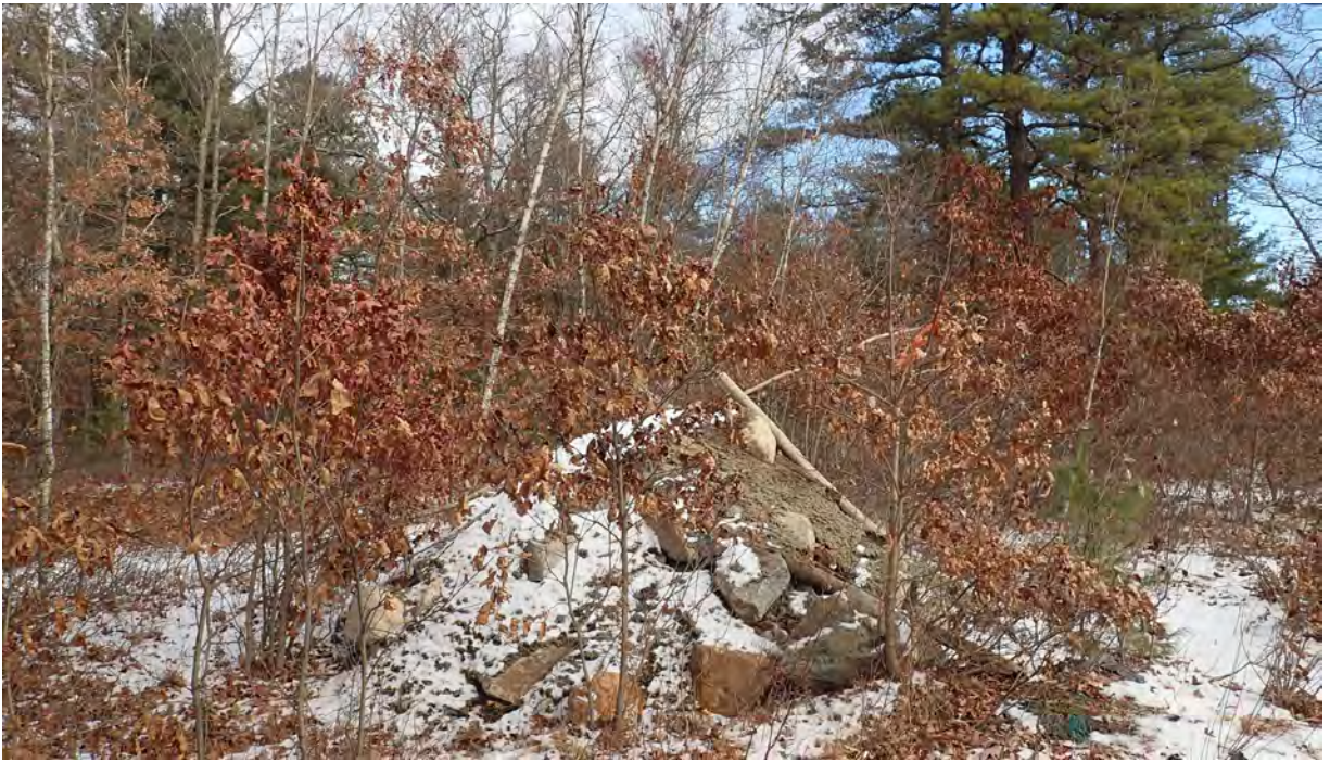
Photo #1: View of installed rock pile in Segment 7 by the Sudbury Town line. Facing east.
