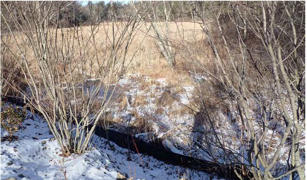
Photo #2: View of installed fallen tree near Bridge 127 in Segment 8. Facing northwest.
