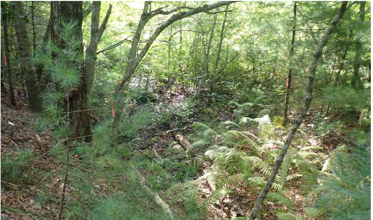
Photo #2: View of installed downed trees in Segment 8. No sediment or construction debris observed within the resource area or beyond the silt fencing. Facing east.
