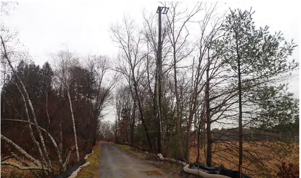
Photo #10: View of installed osprey nest on the east side of Bridge 127 in Segment 14. Facing east.
