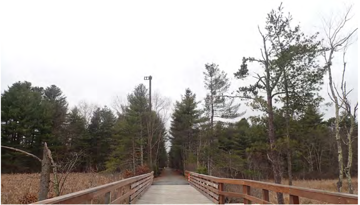
Photo #3: View of installed osprey nest by Bridge 128 in Segment 7. Facing west.
