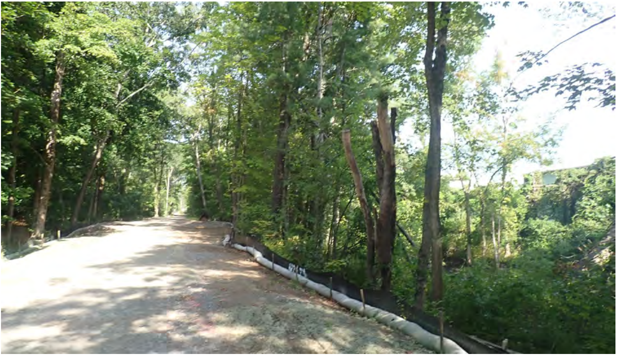
Photo #3: View of installed snag in Segment 13. Snag appears to stable. Silt fencing is in good condition. No sediment or debris observed in the resource area or associated buffer zones. Facing west.
