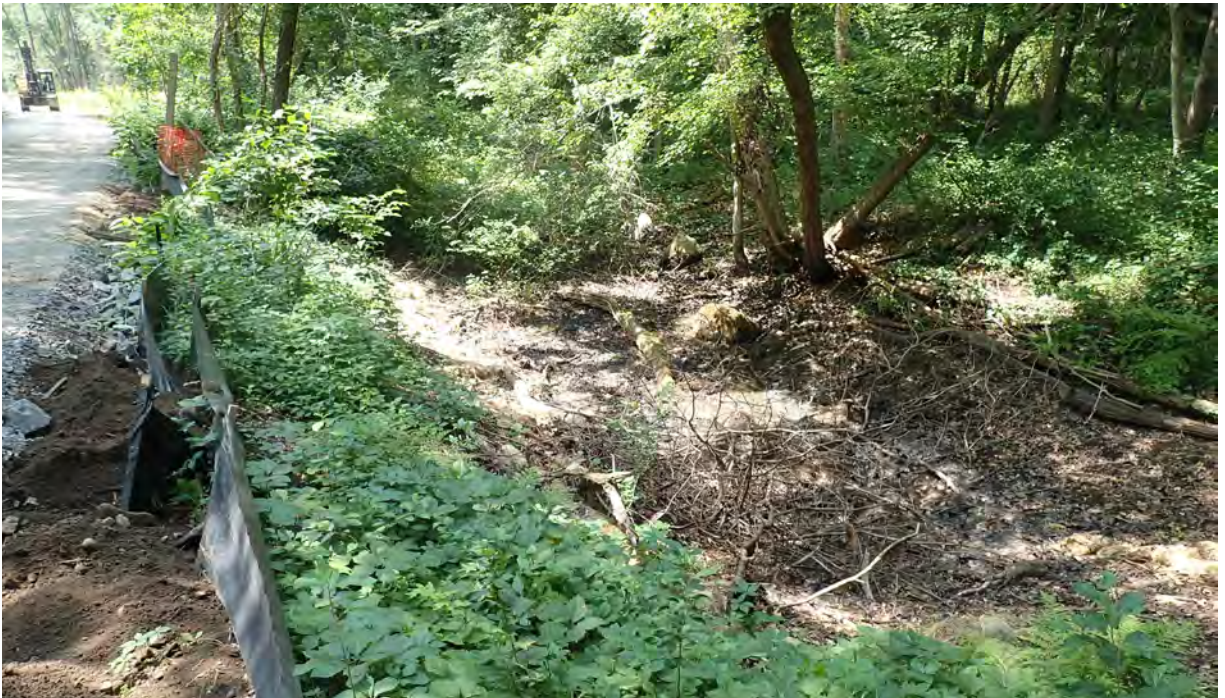
Photo #4: View of installed downed tree within vernal pool #12 in Segment 14. Silt fence has recently been repaired in this area. No sediment or debris observed within the resource area. Facing west.
