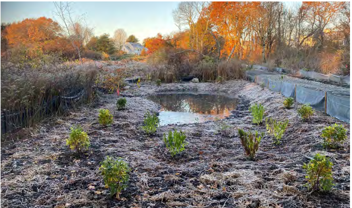
Photo #6: View of installed plantings within the wetland mitigation area. Understory was seeded with a wetland seed mix and stabilized with straw mulch. Photo taken October 27, 2023. Facing west.
