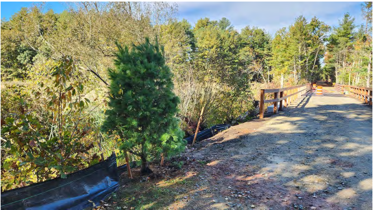
Photo 3: New plantings at Bridge 128. Photo taken on 10/15/24
