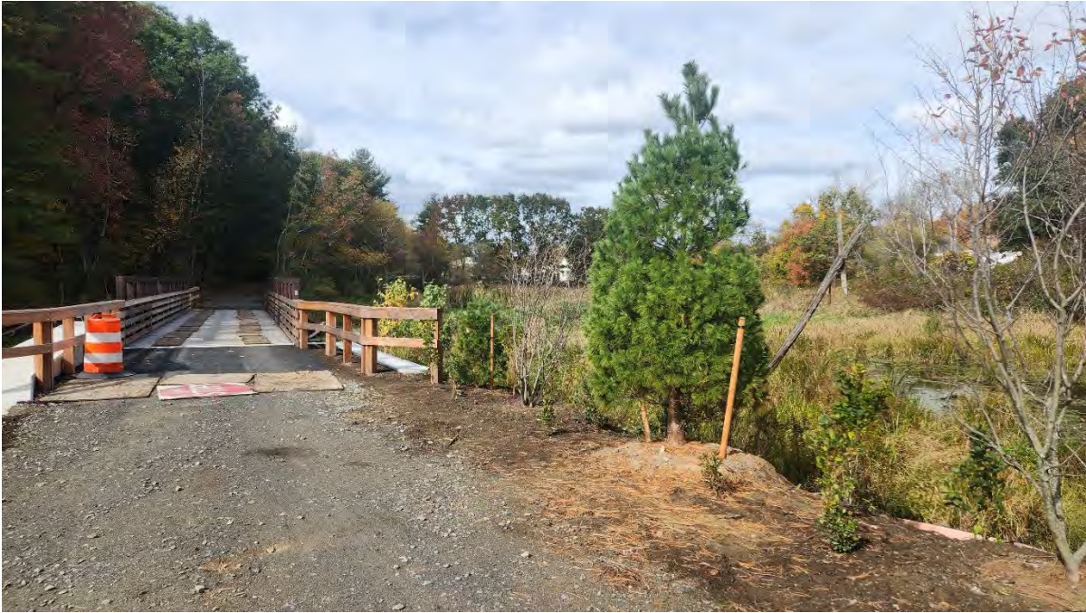
Photo 6: New plantings at Bridge 127. Photo taken on 10/15/24.
