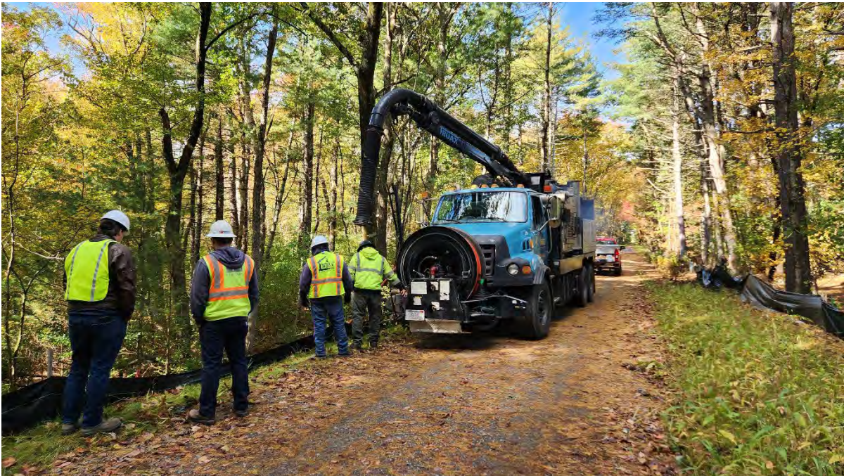
Photo 4: Vacuum truck clearing culverts along segment 9. Photo taken on 10/15/24
