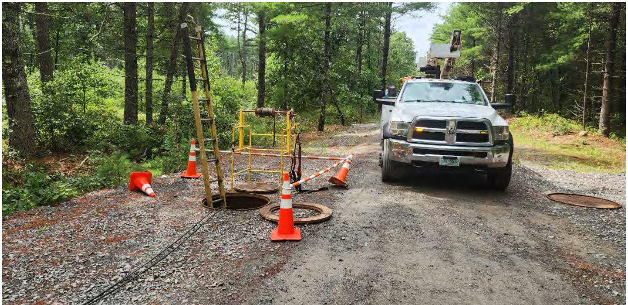
Photo 1: Cable pulling along segment 7. Photo taken on 8/09/24
