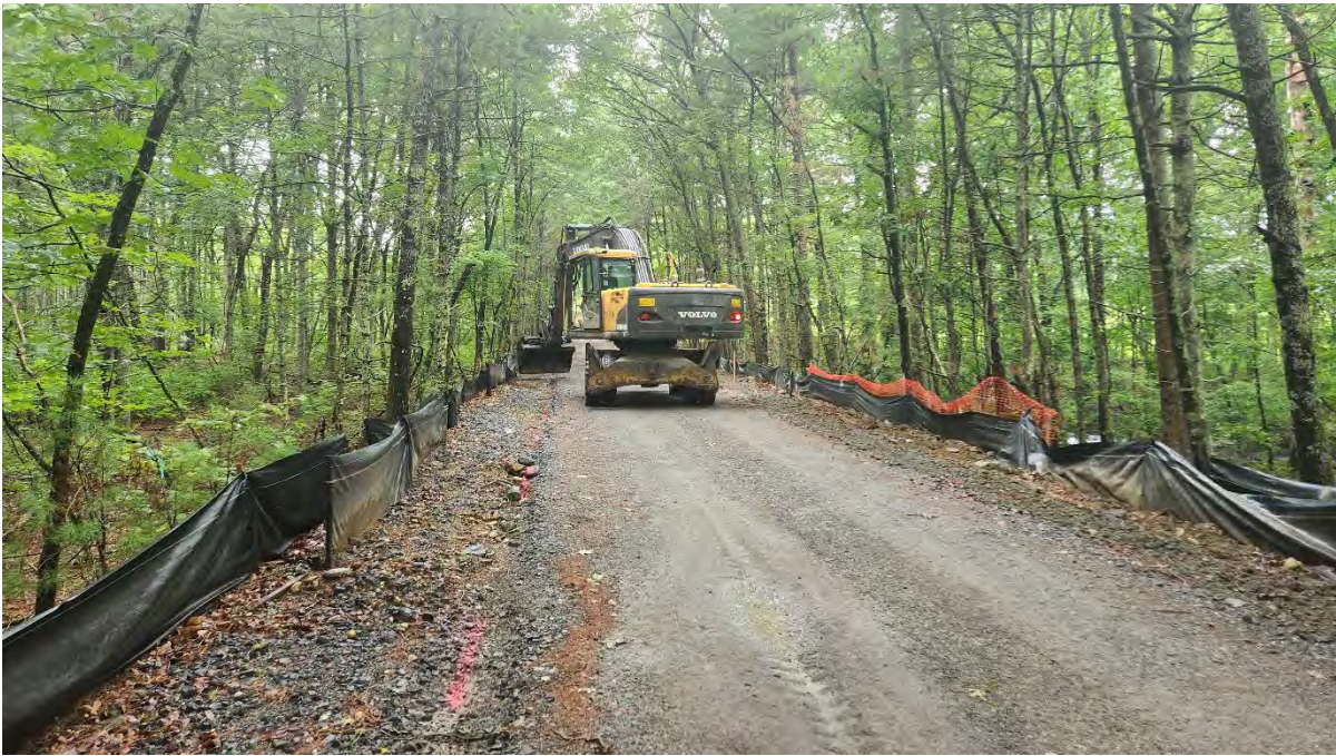
Photo 2: Grading conducted along segment 8. Photo taken on 8/09/24
