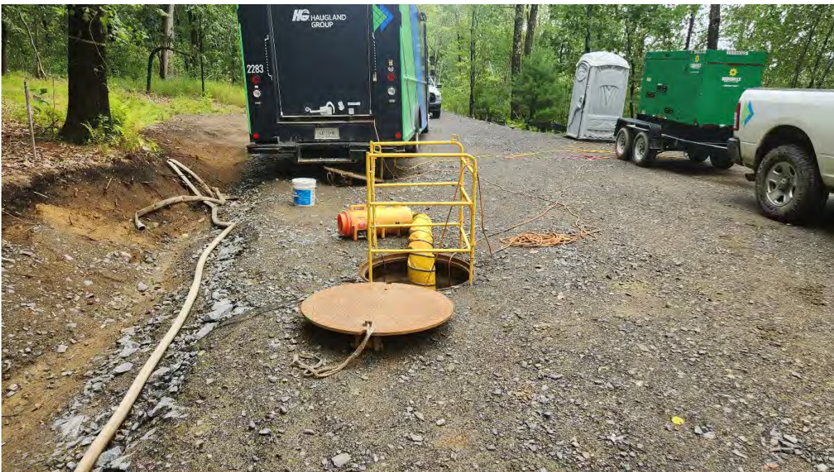
Photo 7: Cable splicing conducted along segment 14. Photo taken on 8/09/24.
