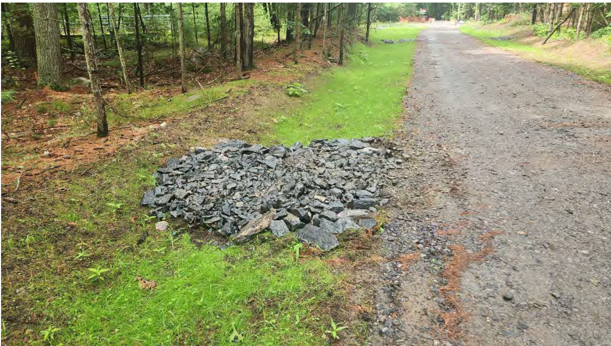
Photo 3: Gravel check dams installed along segment 9. Photo taken on 8/09/24
