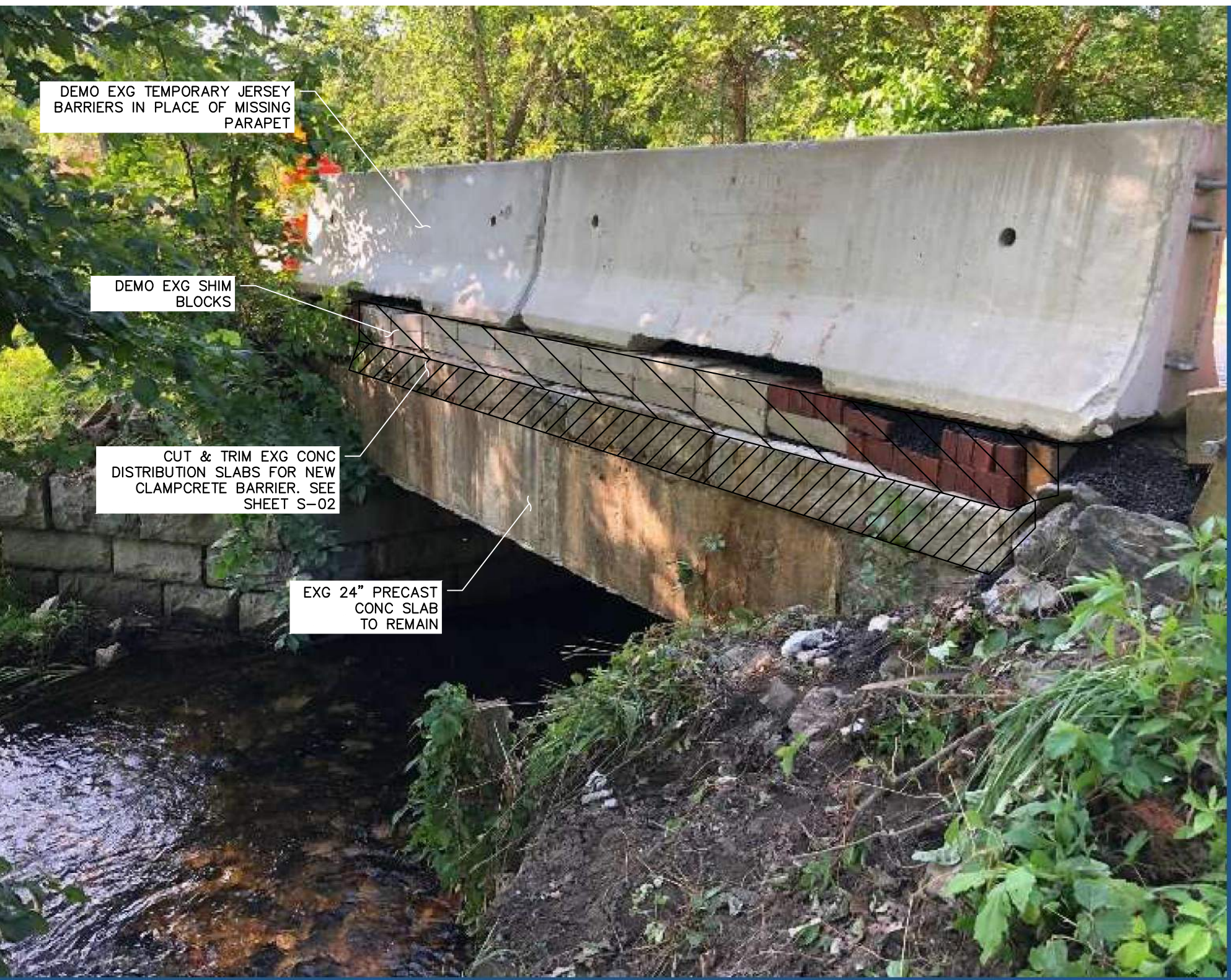
PHOTO 2: EXISTING CONDITIONS - MISSING PARAPET
