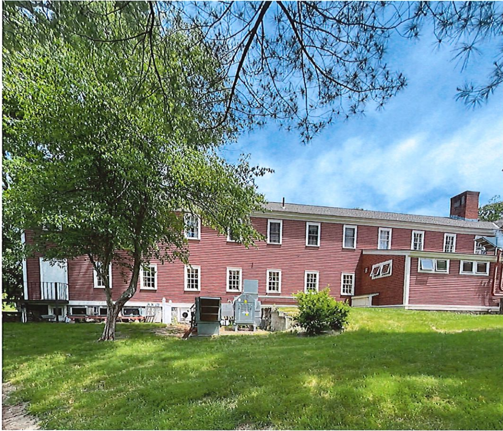
Photo 2. Looking at area of proposed work within lawn and adjacent to existing building
