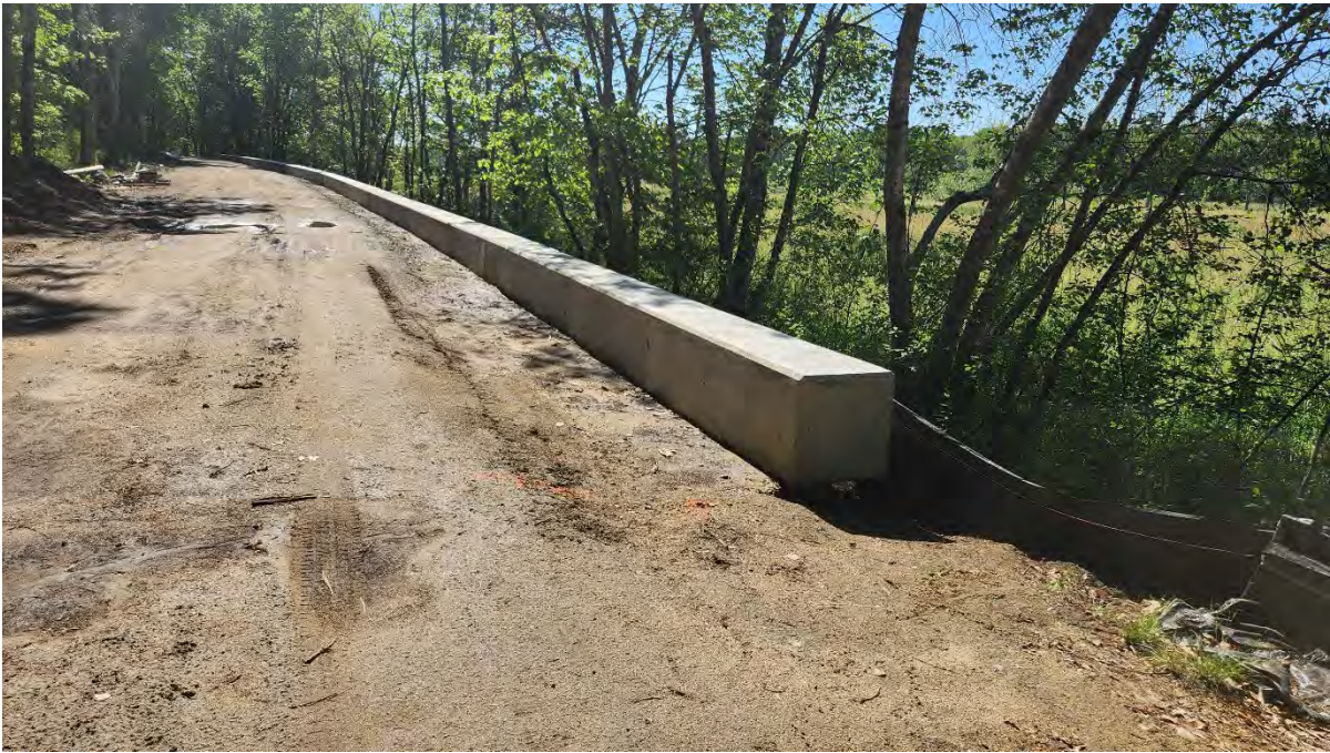
Photo 6: Concrete cap installed over sheeting wall along segment 14. Photo taken on 5/31/24.
