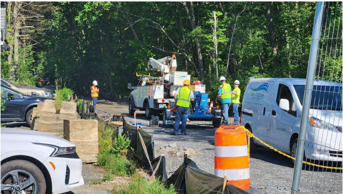
Photo 3: Cable splicing work along segment 11. Photo taken on 5/31/24
