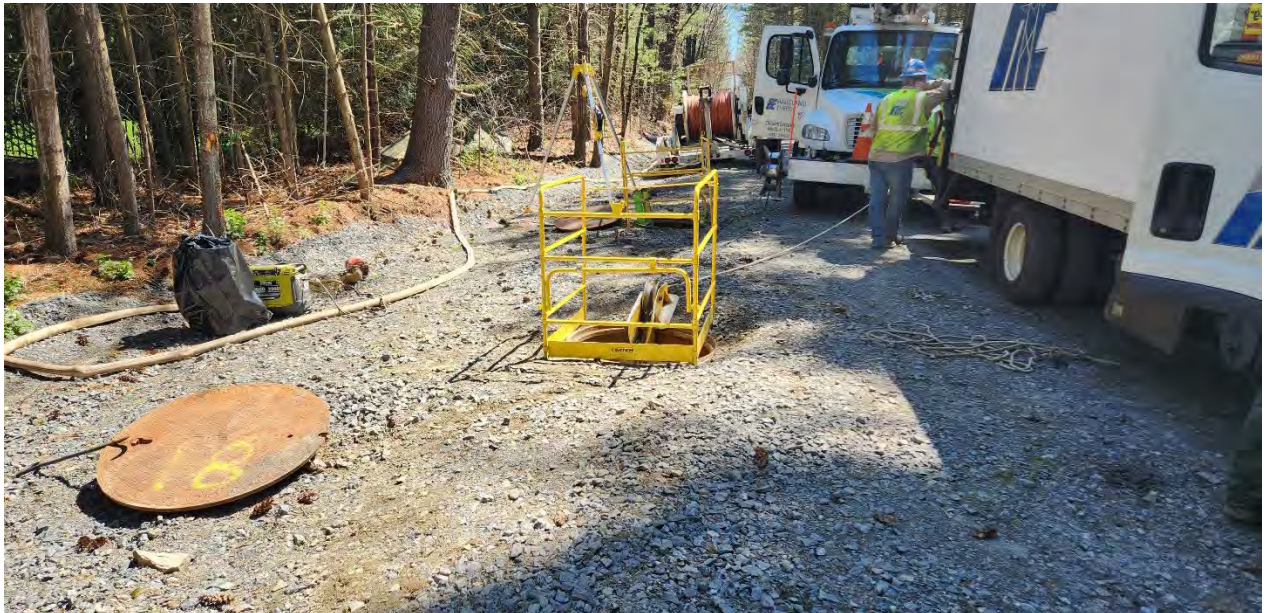
Photo 1: Cable pulling work along segment 7. Photo taken on 4/22/24
