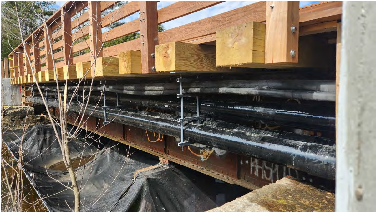
Photo 2: Conduit crossing installed underneath Bridge 128. Photo taken on 3/27/24
