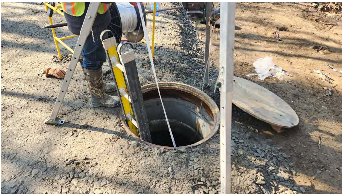
Photo 3: Mule tape blowing in progress along segment 8. Photo taken on 2/27/24
