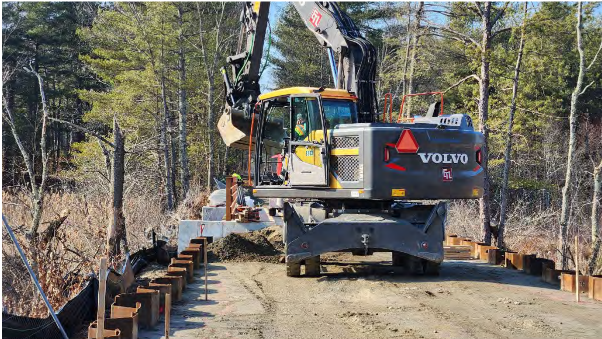
Photo 2: Wall cap installation under progress at Bridge 127. Photo taken on 2/27/24
