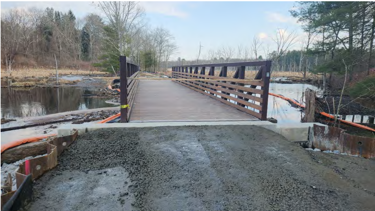
Photo 5: Bridge 127 installed. Photo taken on 2/27/24.
