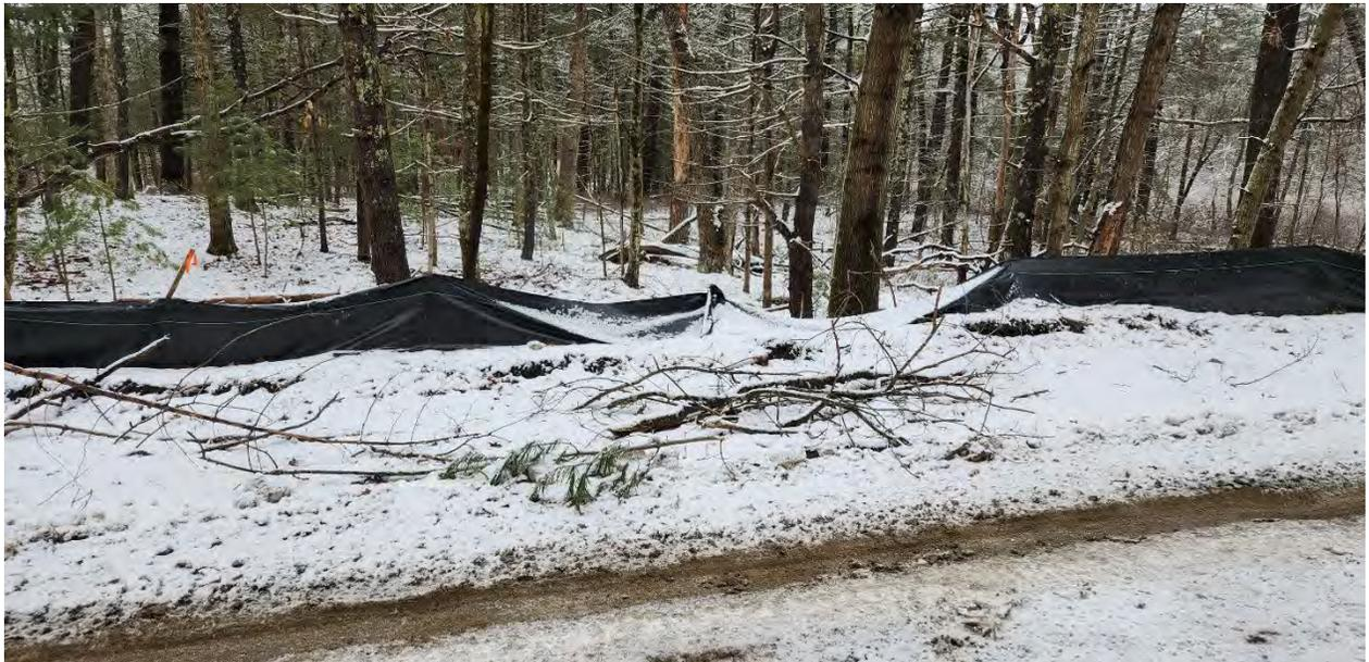
**Photo 1:** Broken stake in the silt fence along segment 8.
