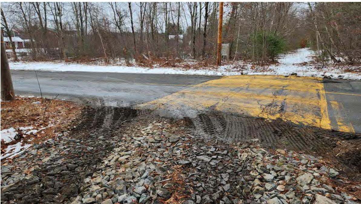
**Photo 5:** Sediment is tracked into the road at construction entrance STA 407+.
