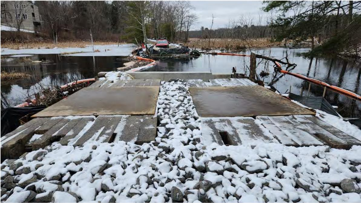
**Photo 6:** Gravel base installed at Bridge 127 along segment 13 while dewatering across Hop Brook.
