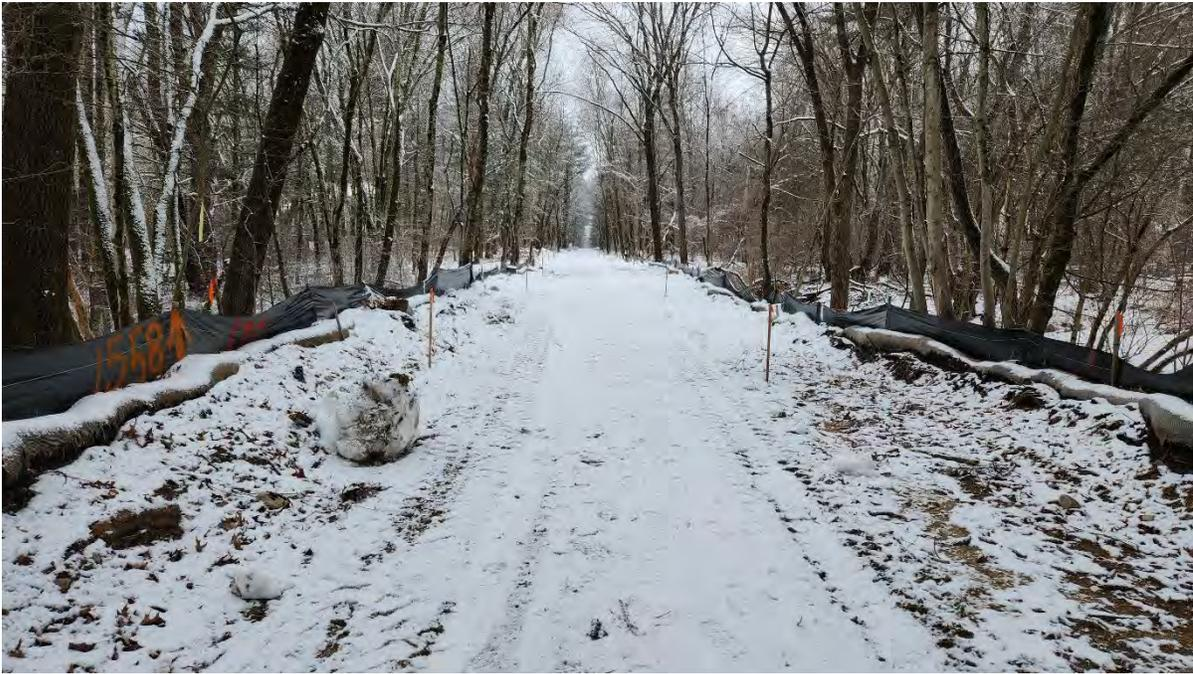
**Photo 4:** Stakes set along segment 9 at proposed path width for gravel base installation.
