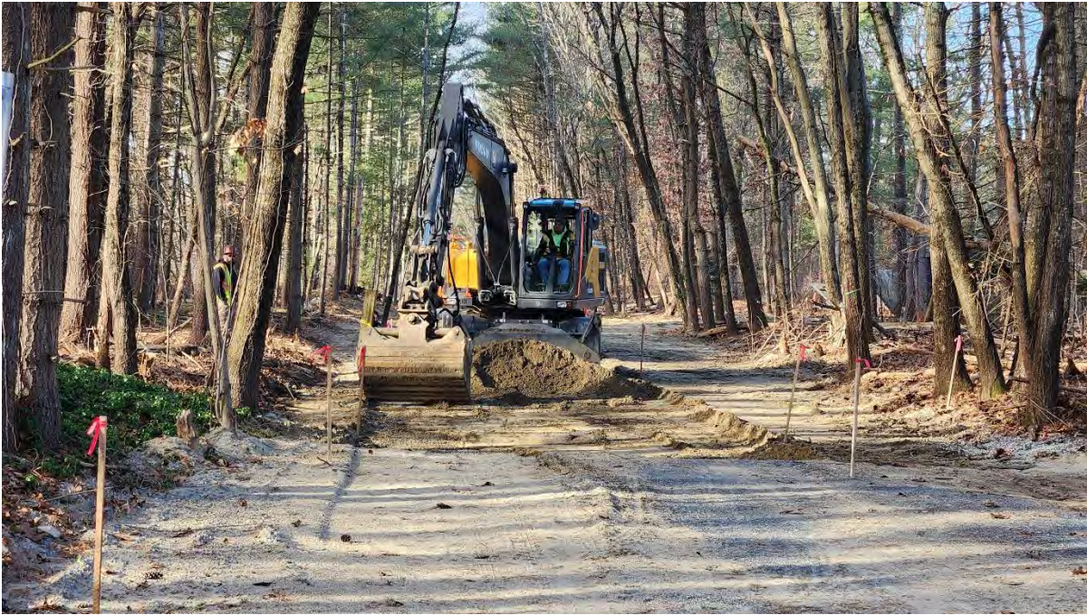
Photo 4: Excavation along segment 10. Photo taken on 12/14/23
