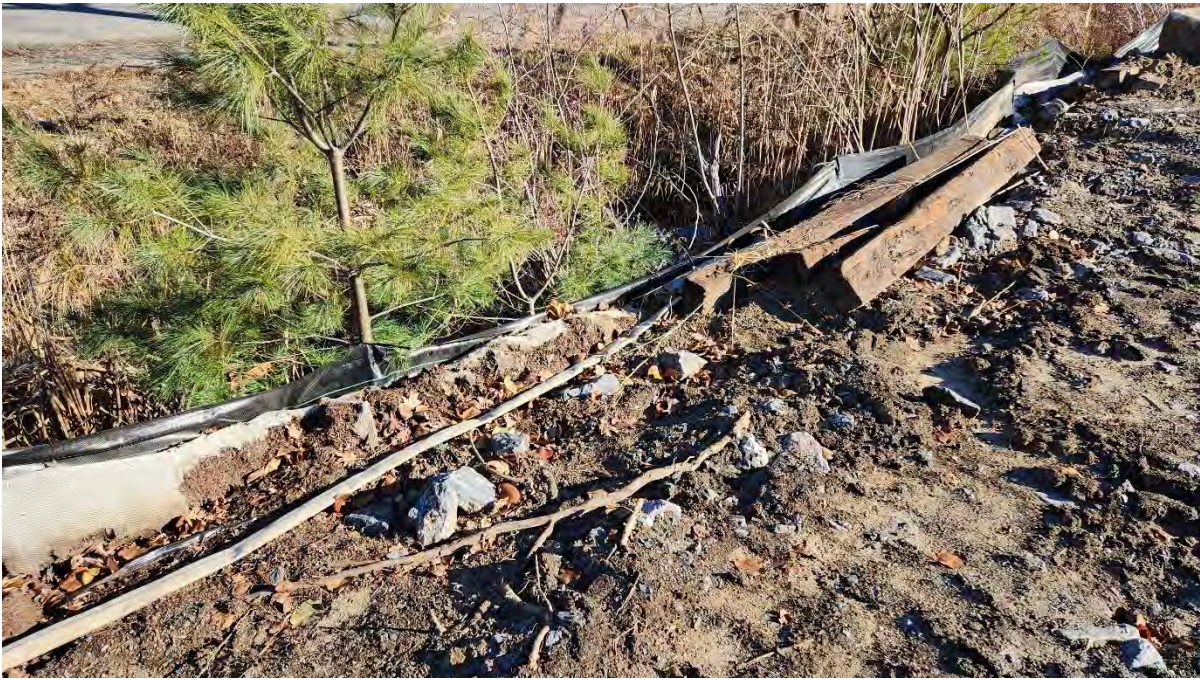
Photo 2: Filter tube ripped and silt fence sagging along segment 12. Photo taken on 12/14/23
