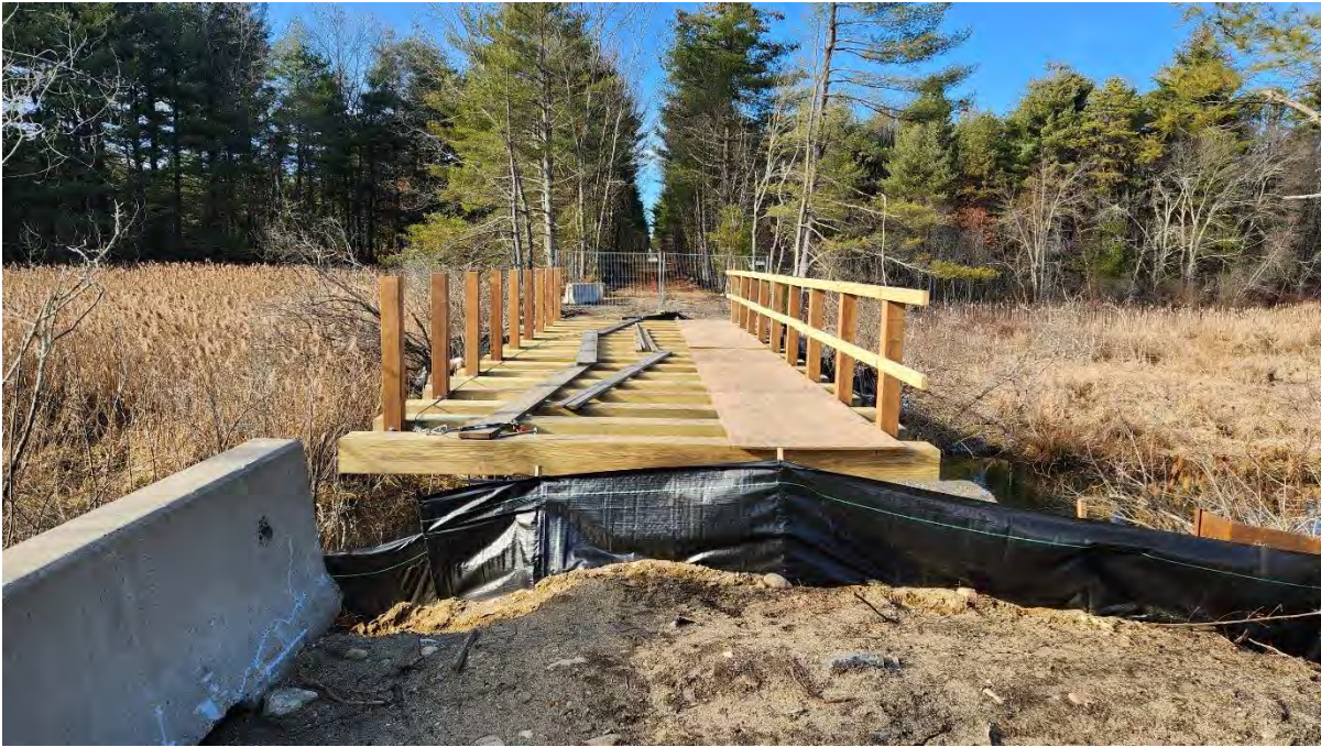
Photo 6: Bridge 127 under construction between segments 7 and 8. Photo taken on 12/14/23.
