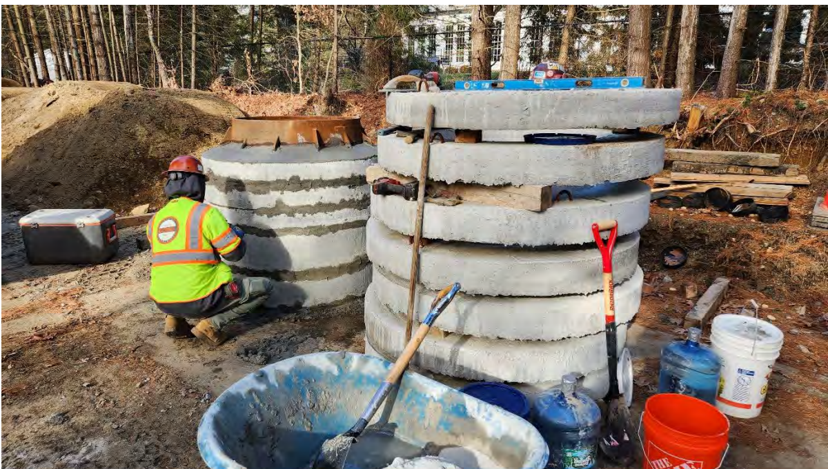
Photo 5: Hand holes being prepped for installation along segment 9. Photo taken on 12/14/23
