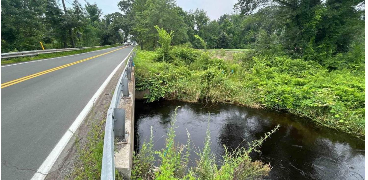
Photo #7: View of Union Ave over Hop Brook. Facing southwest.
