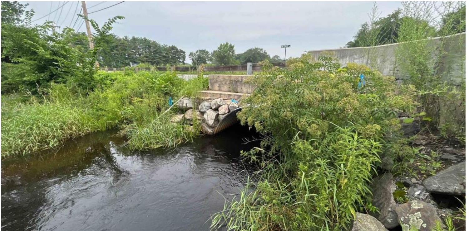
Photo #9: View of Codjer Lane culvert. Facing northwest.
