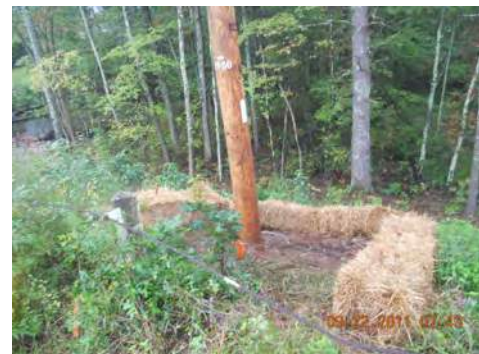
FIGURE 2: ALT. STRAW BALE APPLICATION
