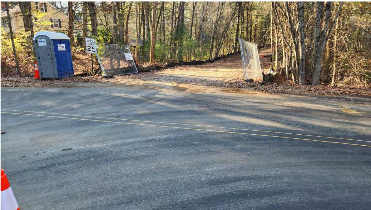
**Photo 3:** Sediment tracked into the road at gravel construction entrance STA 335+50.
