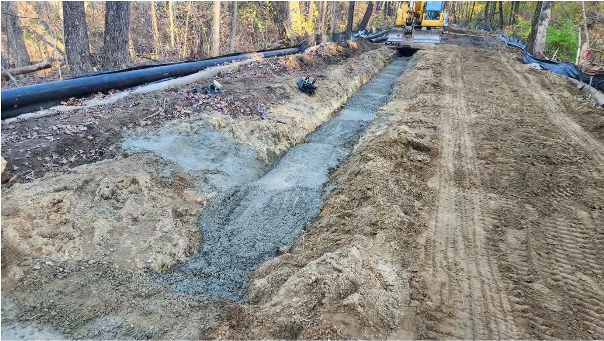
**Photo 6:** Installed conduit covered in concrete along segment 13.
