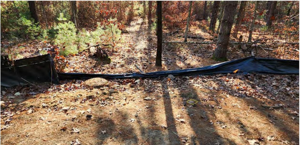
**Photo 1:** Rip in the silt fence along segment 7.
