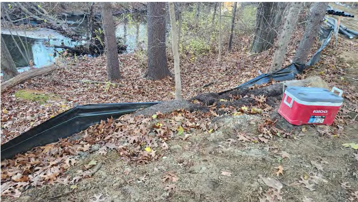
**Photo 5:** Broken stakes in the silt fence along segment 13.
