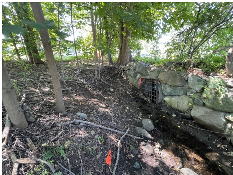
Photo 4: Northerly view of B Series BVW boundary and culvert.
