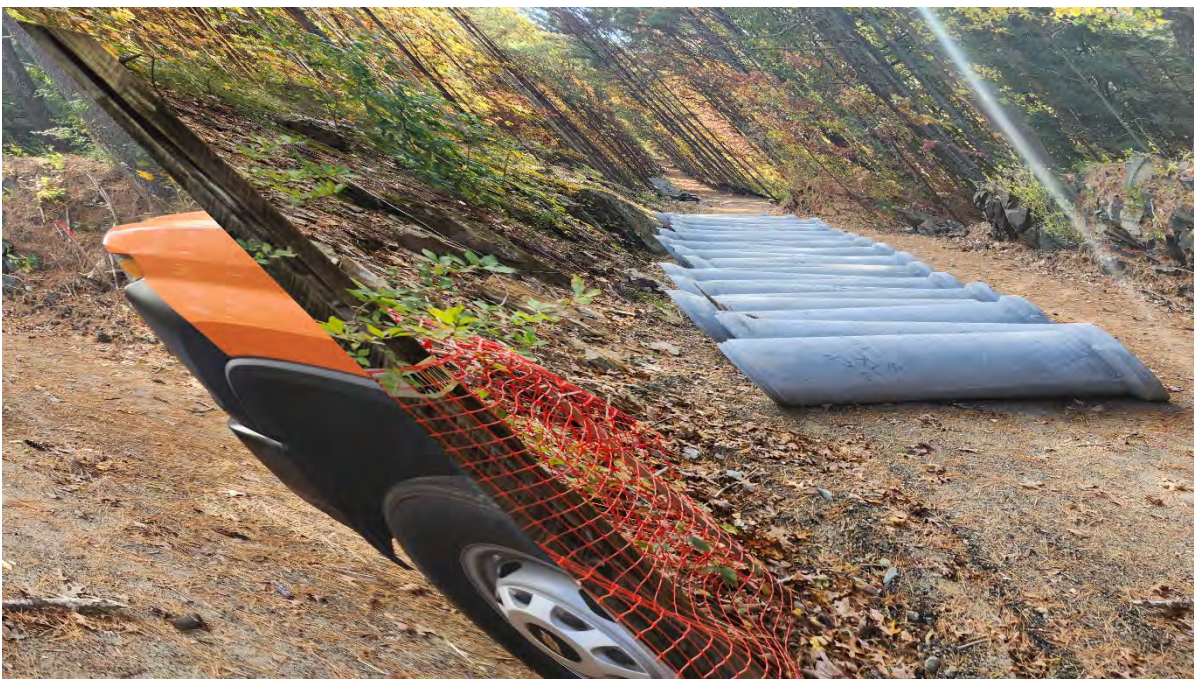
Photo 3: Drainage pipes along segment 10 waiting for structure installation. Photo taken on 10/23/23
