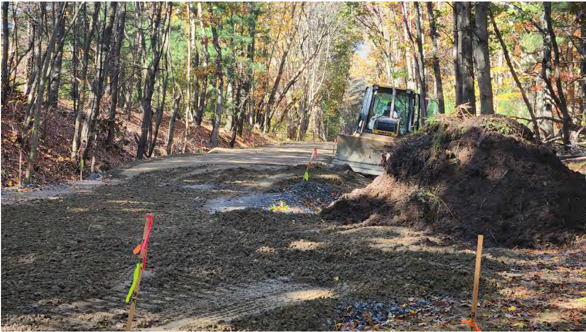
Photo 6: Earthwork activity along segment 11. Photo taken on 10/23/23
