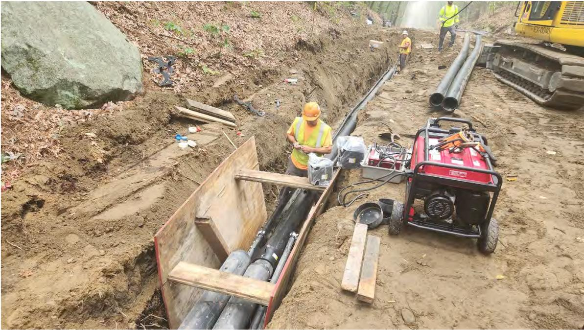
**Photo 2:** Conduit being installed along segment 9.
