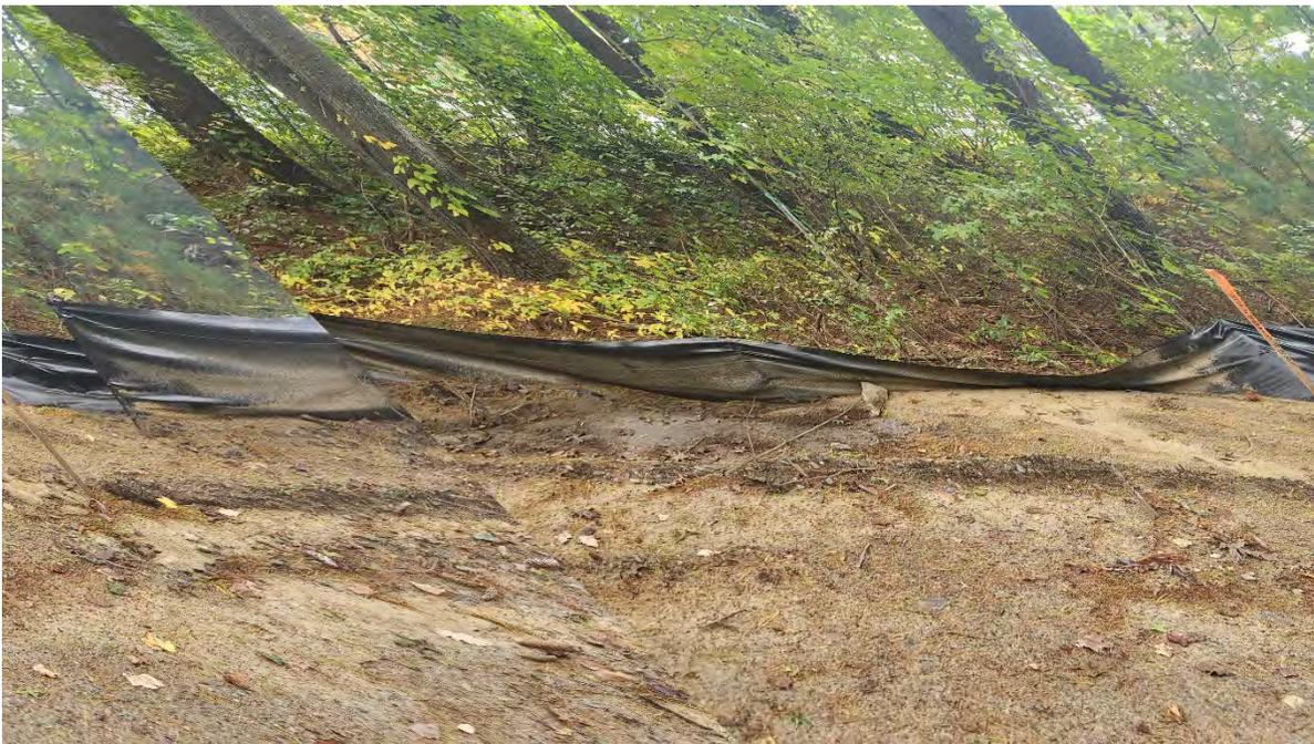
**Photo 3:** Broken stake in the silt fence along segment 11.
