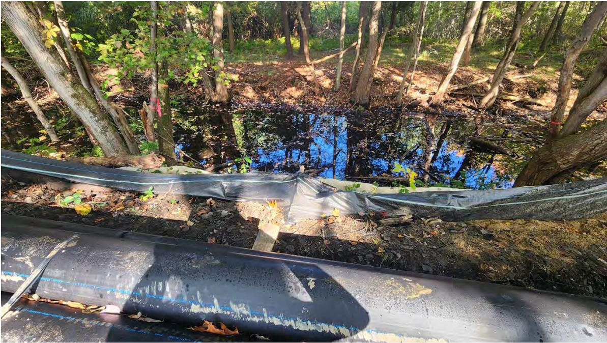
**Photo 4:** Stake in silt fence broken along segment 14.
