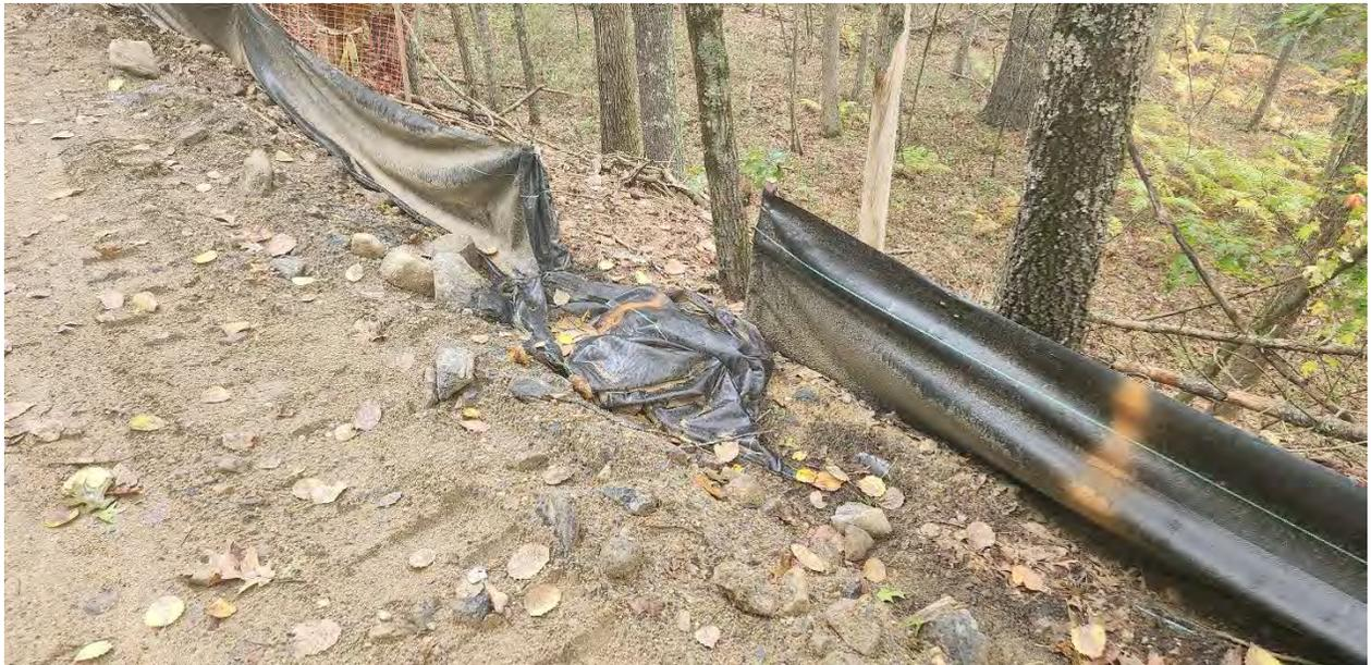
**Photo 1:** Rip in the silt fence along segment 8.
