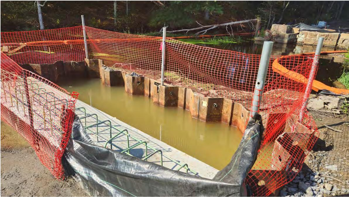
**Photo 6:** Wall stripped and backfilled at Bridge 127 along segment 14.
