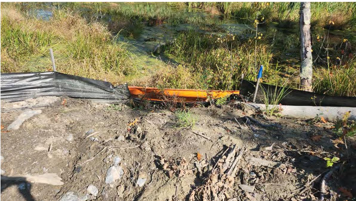
**Photo 5:** Rip in the silt fence near Bridge 127 along segment 14.
