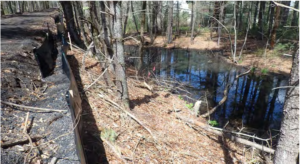
Photo #2: View of vernal pool #9 in Segment 10. No sediment or debris observed within the resource area or associated buffer zone. Silt fencing here and throughout the project area is in good condition. Pair of wood ducks and pair of mallard ducks observed in the vernal pool. Facing northwest.
