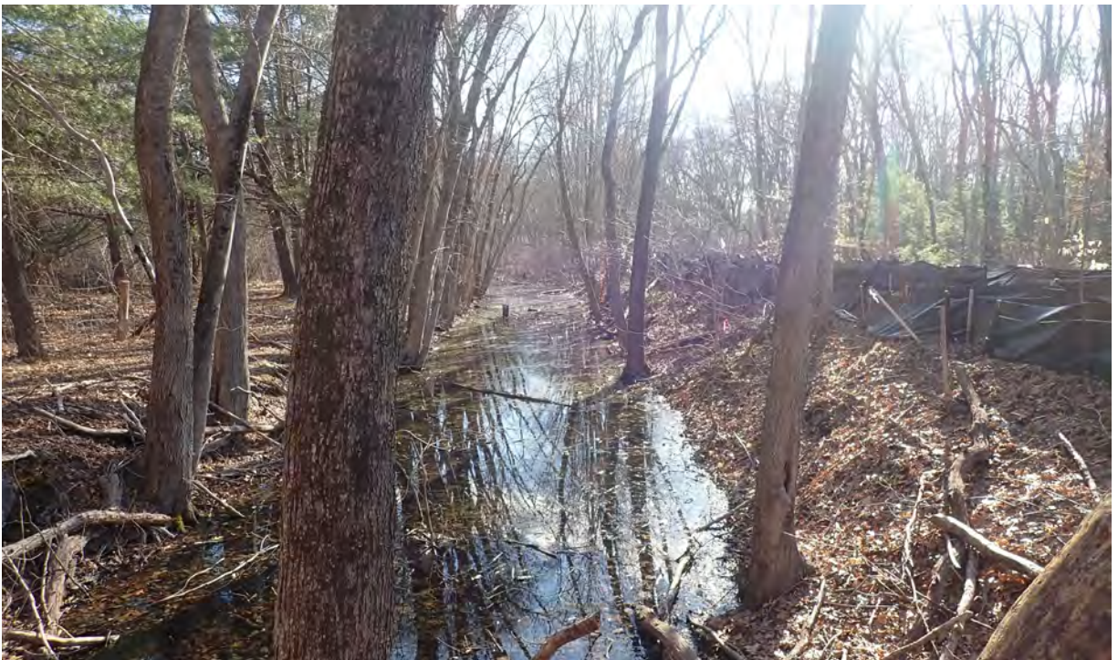
Photo #4: View of vernal pool #13 in Segment 14. Silt fence in good condition. No sediment or debris observed in the resource area or associated buffer zones. Facing east.
