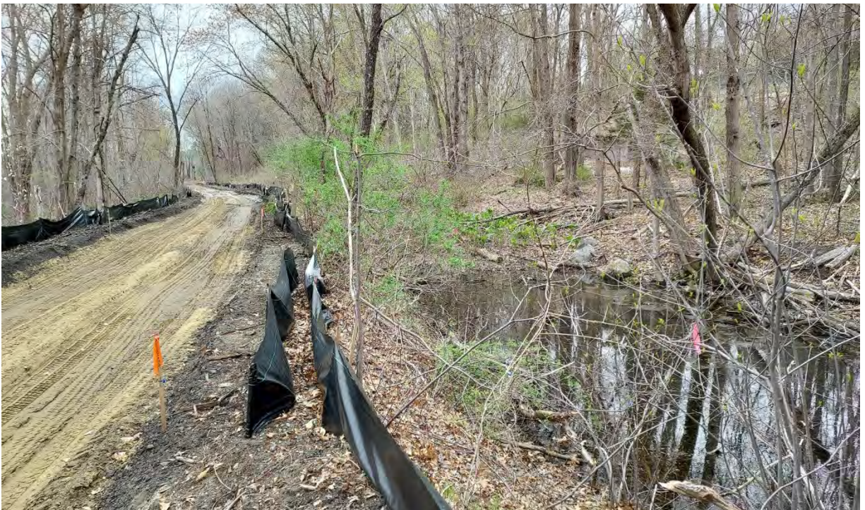
Photo #4: View of vernal pool #12 in Segment 14. Silt fence in good condition. No sediment or debris observed in the resource area or associated buffer zone. Facing west.
