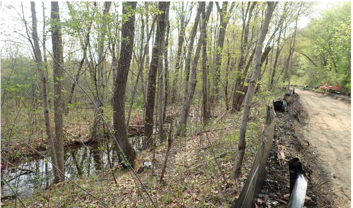
Photo #4: View of vernal pool #14 in Segment 14. Silt fence in good condition. No sediment or debris observed in the resource area or associated buffer zone. Facing west.
