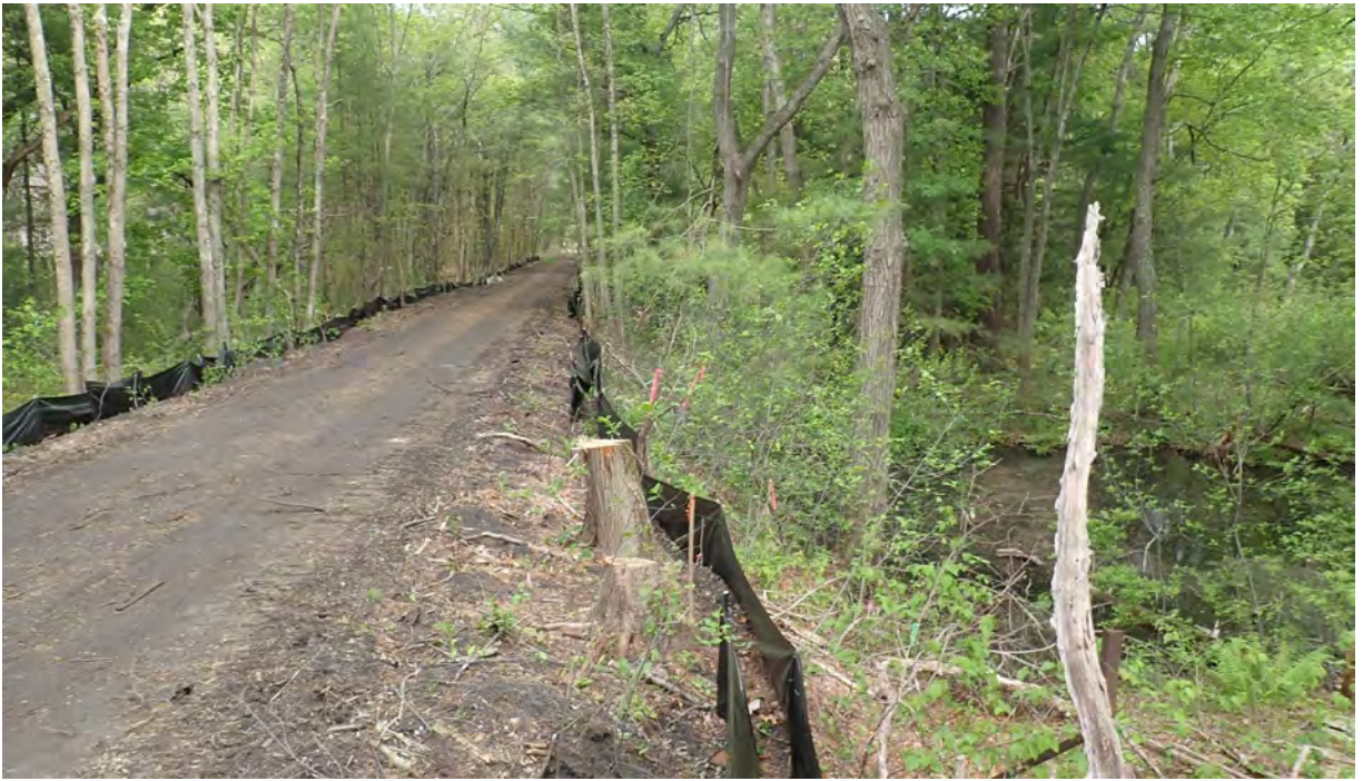
Photo #3: View of vernal pool #10 in Segment 11. Silt fence in good condition. No sediment or debris observed in the resource area or associated buffer zone. Facing northwest.
