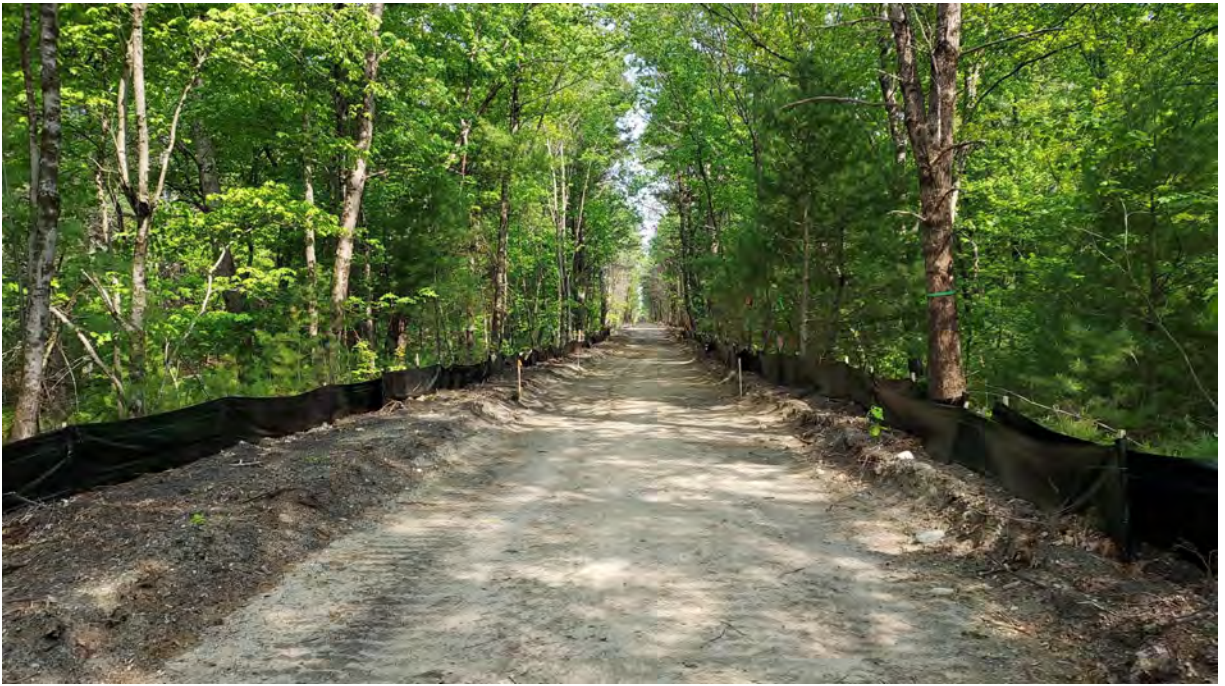
Photo #1: View of project area near vernal pools #1 in Segment 7. Silt fence is in good condition. No sediment or debris observed within the resource area, buffer zone, or project area. Facing northwest.
