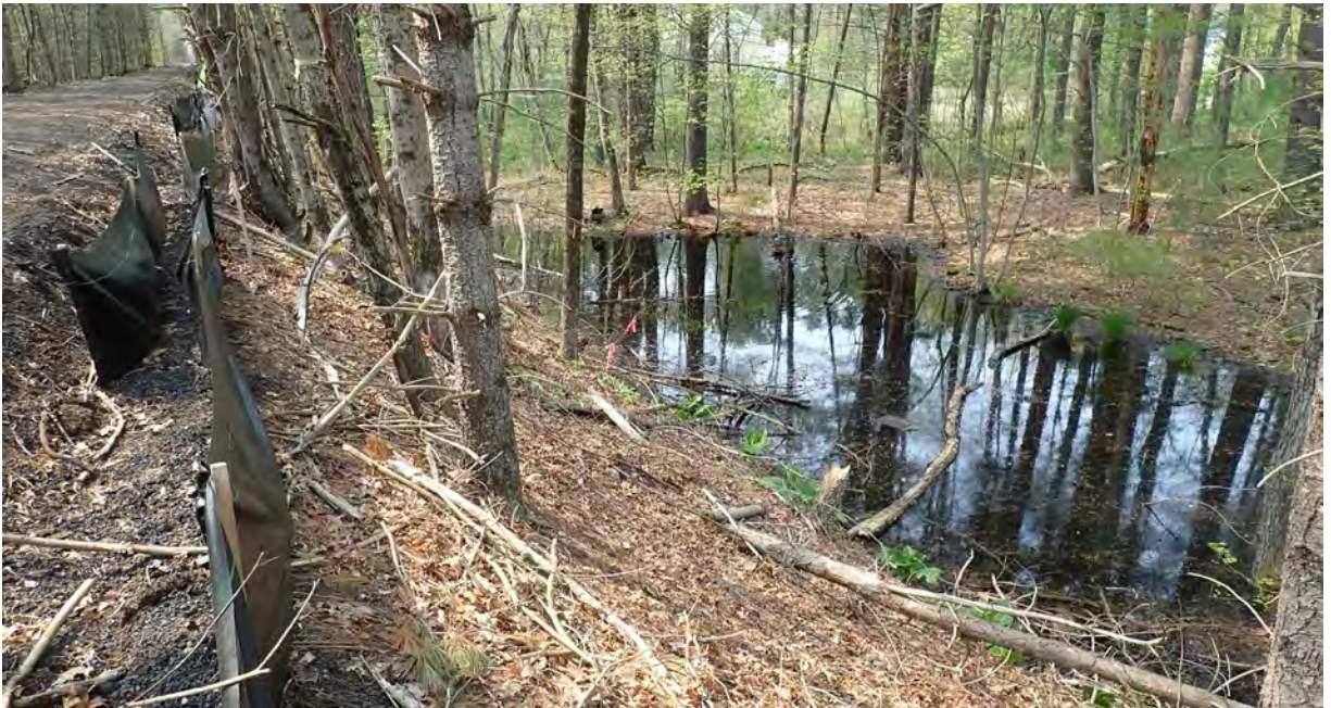
Photo #2: View of vernal pool #9 in Segment 10. No sediment or debris observed within the resource area or associated buffer zone. Silt fencing here and throughout the project area is in good condition. Pair of mallard ducks and wood ducks observed within vernal pool. Facing northwest.
