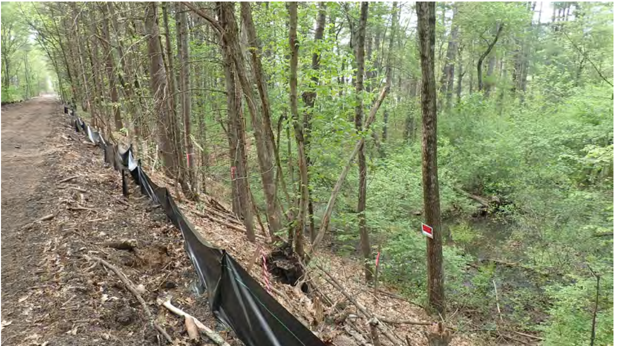
Photo #2: View of vernal pool #8 in Segment 10. No sediment or debris observed within the resource area or associated buffer zone. Silt fencing here and throughout the project area is in good condition. Facing northwest.
