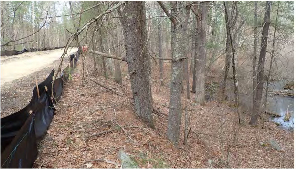
Photo #1: View of project area near vernal pool #7 and in Segment 8. Silt fence is in good condition. No sediment or debris observed within the resource area, buffer zone, or project area. Facing northwest.
