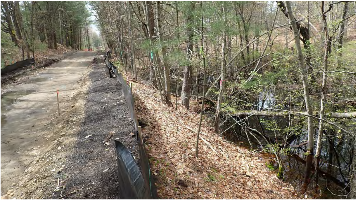
Photo #1: View of project area near vernal pool #3 and in Segment 8. Silt fence is in good condition. No sediment or debris observed within the resource area, buffer zone, or project area. Facing northwest.
