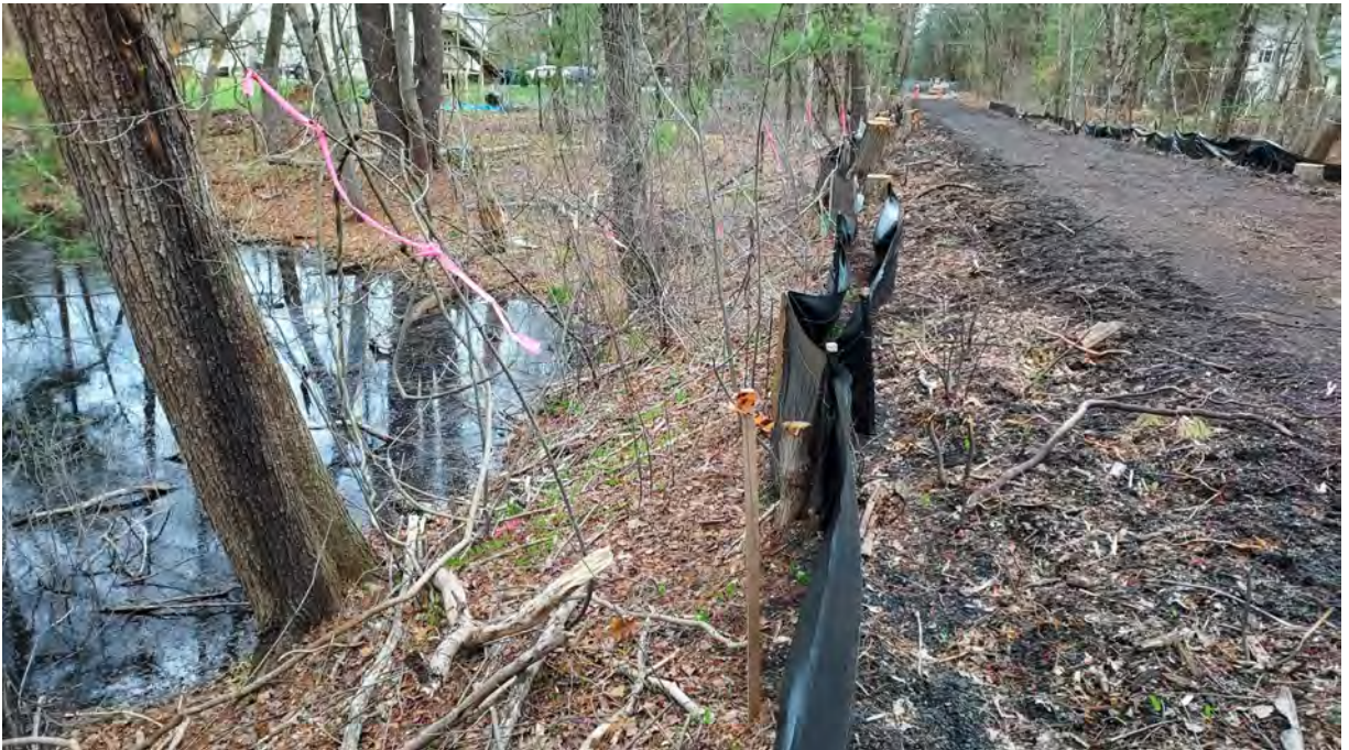
Photo #2: View of vernal pool #9 in Segment 10. No sediment or debris observed within the resource area or associated buffer zone. Silt fencing here and throughout the project area is in good condition. Pair of wood ducks observed in the vernal pool. Facing southeast.
