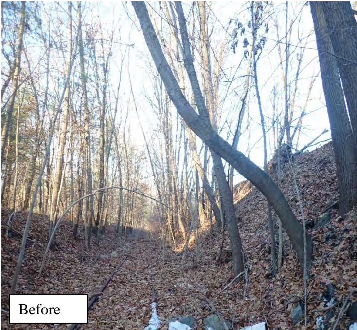
Photo #38: View of tree in Impact Area 19, at station 756+00. The base of the tree is outside the limit of work; however, the tree is leaning into the limit of work and will need to be cut. Base and root will remain in place. Facing west.
