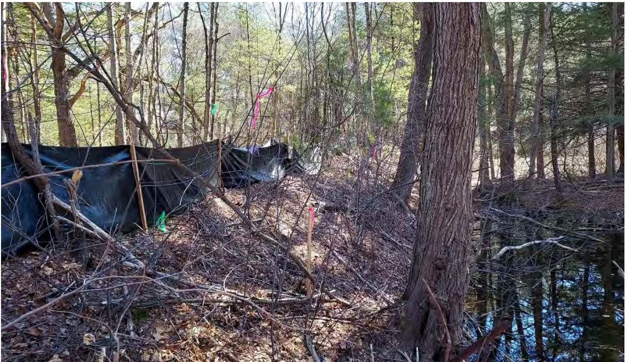
Photo #2: View of vernal pool #10 in Segment 11. No sediment or debris observed within the resource area or associated buffer zone. Silt fencing here and throughout the project area is in good condition. Facing southeast.
