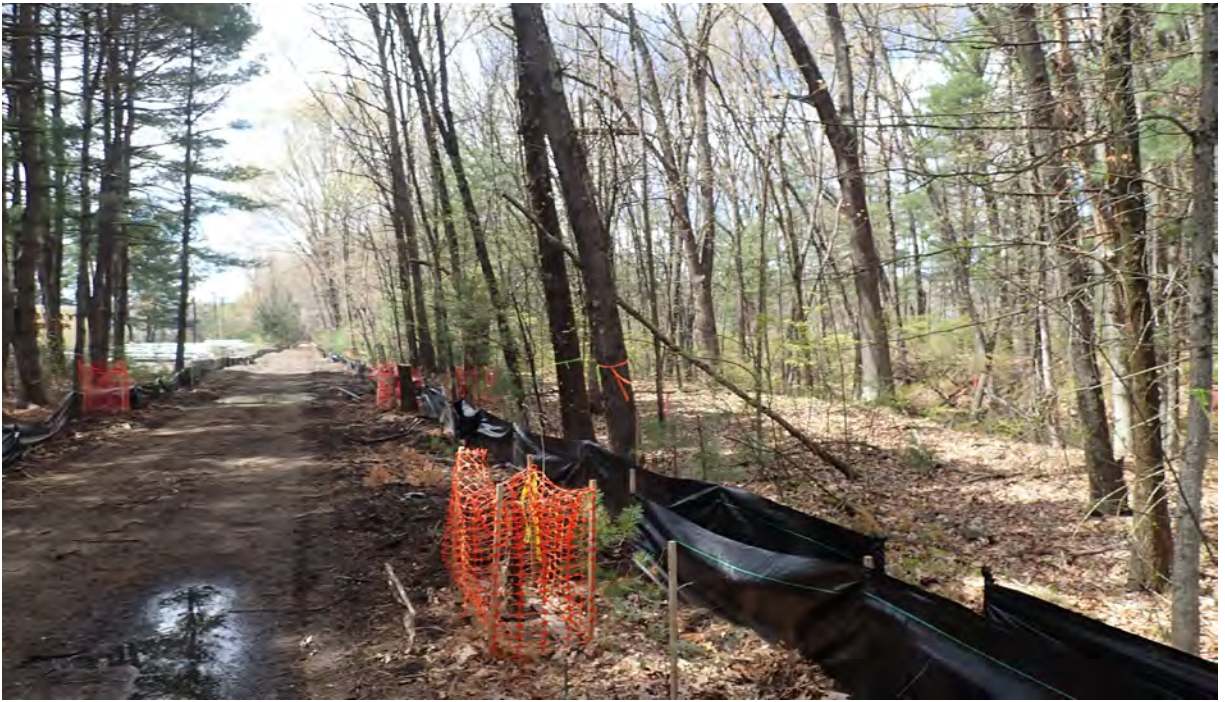
Photo #3: View of project area near vernal pool #11 in Segment 11. Silt fence in good condition. No sediment or debris observed in the resource area or associated buffer zone. Facing northwest.
