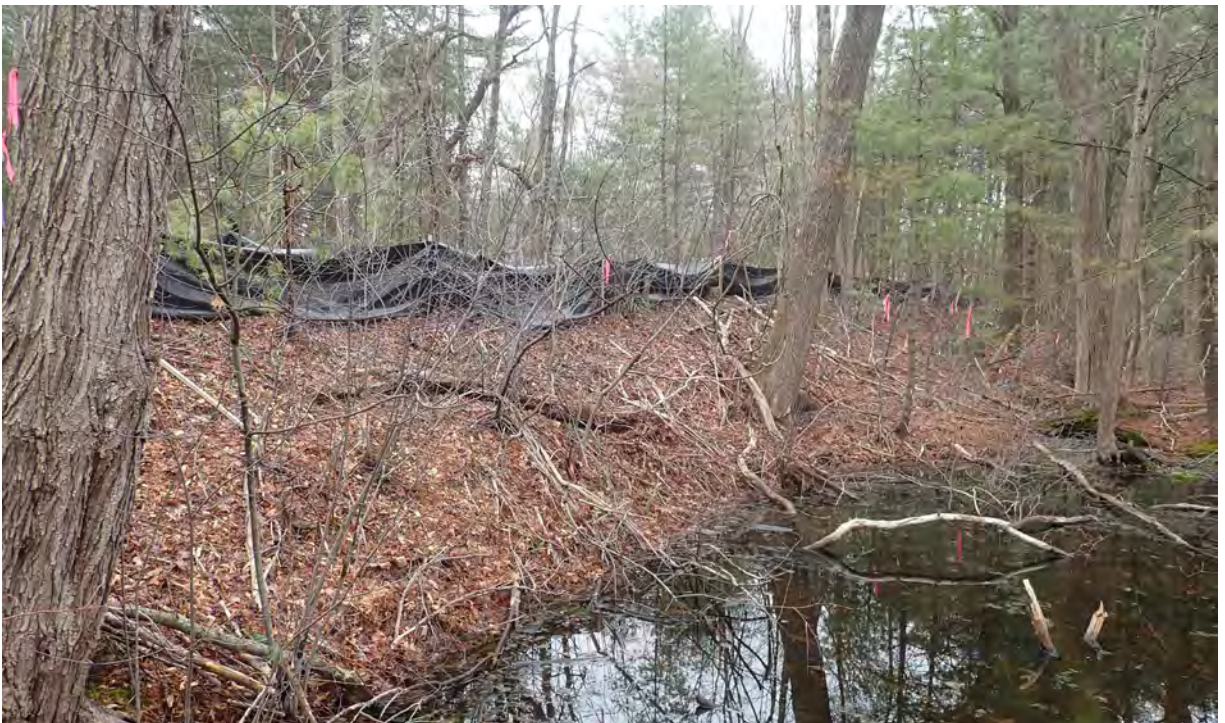
Photo #4: View of vernal pool #10 in Segment 11. Silt fence in good condition. No sediment or debris observed in the resource area or associated buffer zone. Facing southeast.
