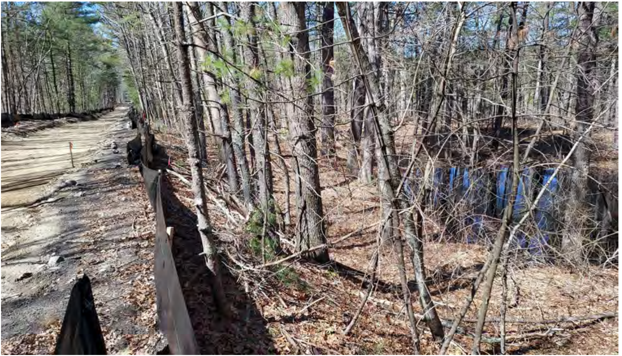
Photo #1: View of vernal pool #6 and in Segment 8. Silt fence is in good condition. No sediment or debris observed within the resource area, buffer zone, or project area. Facing northwest.
