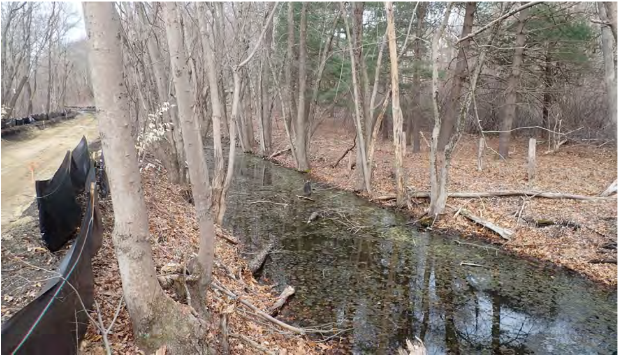
Photo #7: View of vernal pool #13 in Segment 14. Silt fence in good condition. No sediment or debris observed in the resource area or associated buffer zones. Facing west.
