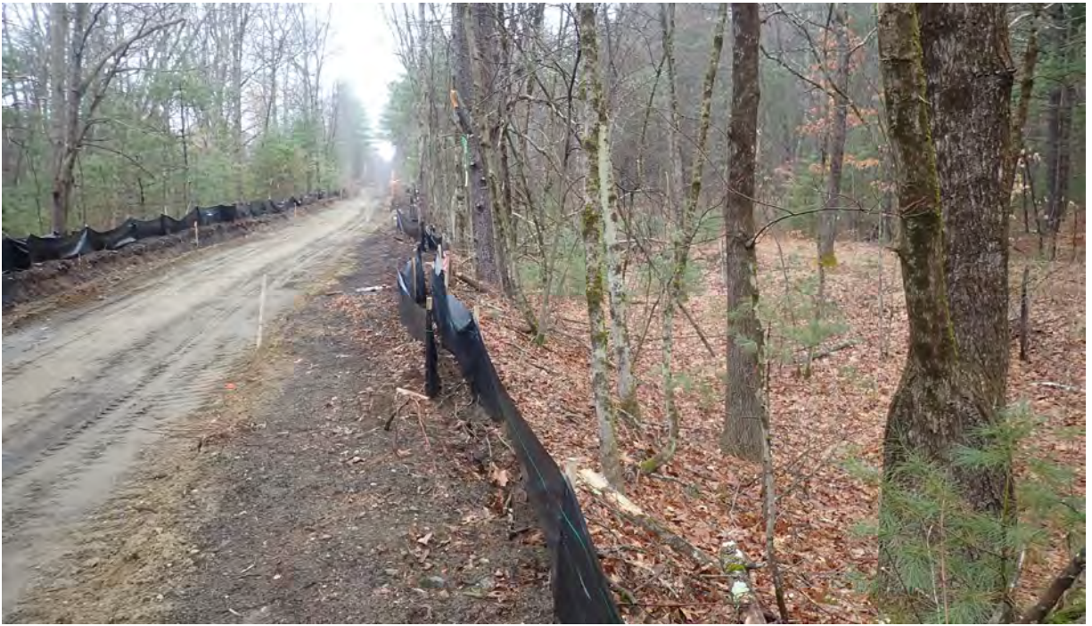
Photo #1: View of project area near vernal pool #1 and in Segment 7. Silt fence is in good condition. No sediment or debris observed within the resource area, buffer zone, or project area. Facing northwest.
