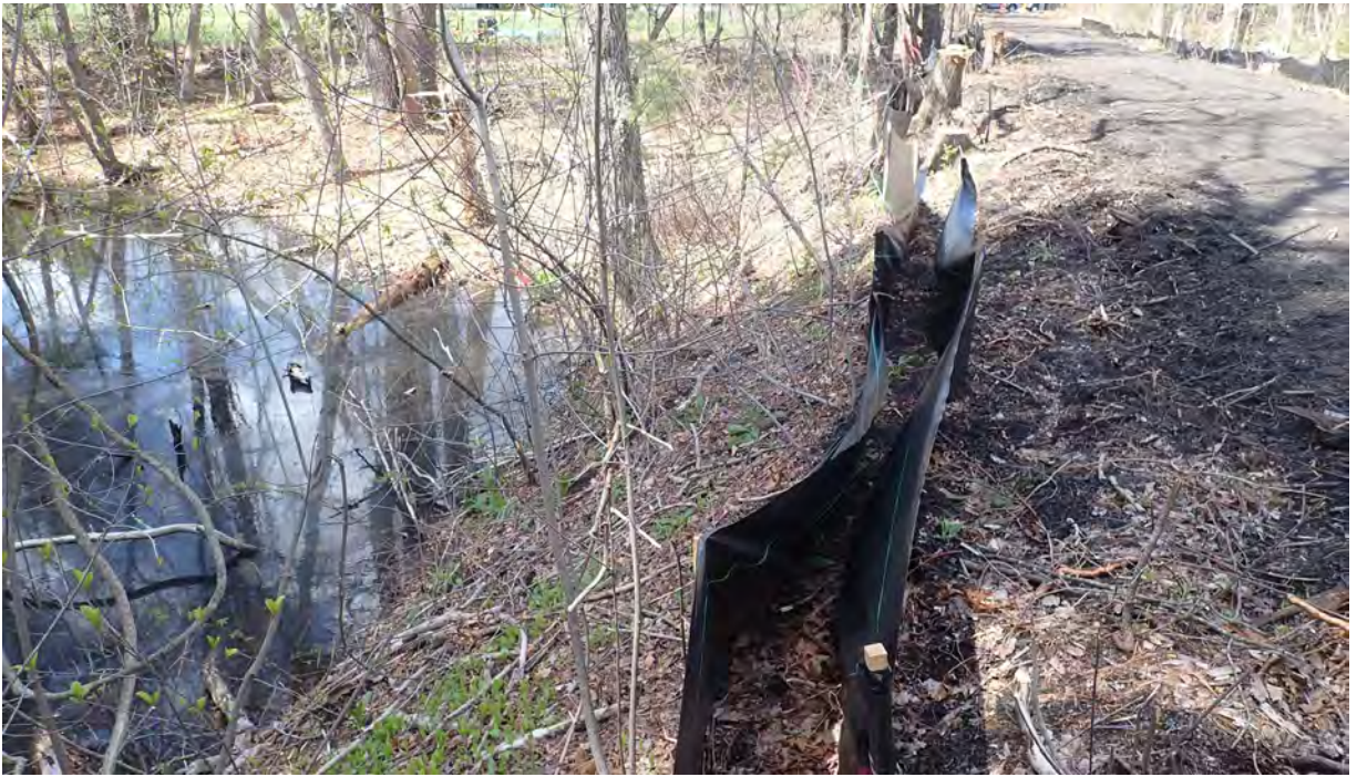
Photo #3: View of vernal pool #10 in Segment 11. Silt fence in good condition. No sediment or debris observed in the resource area or associated buffer zone. Facing southeast.
