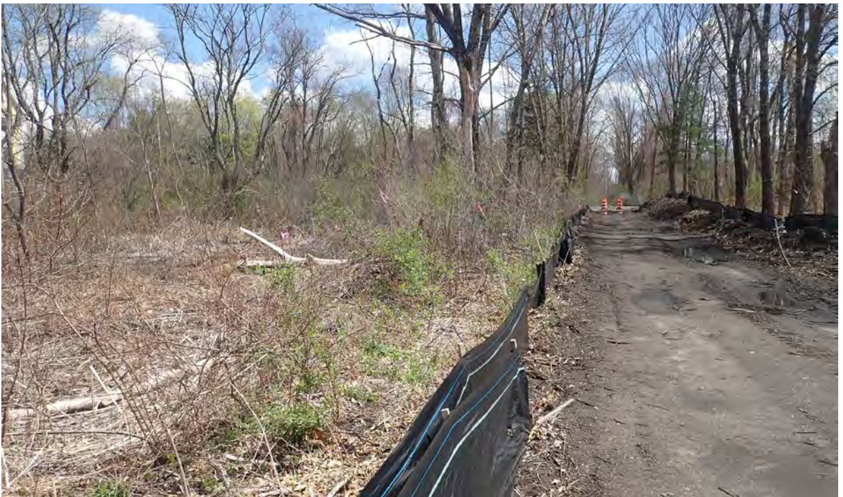
Photo #4: View of vernal pool #15 in Segment 14. Silt fence in good condition. No sediment or debris observed in the resource area or associated buffer zone. Facing east.
