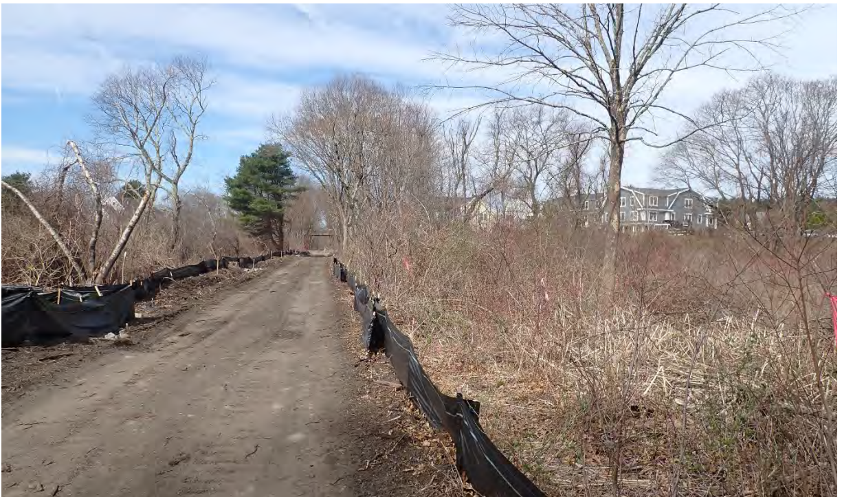
Photo #4: View of vernal pool #15 in Segment 14. Silt fence in good condition. No sediment or debris observed in the resource area or associated buffer zone. Facing east.
