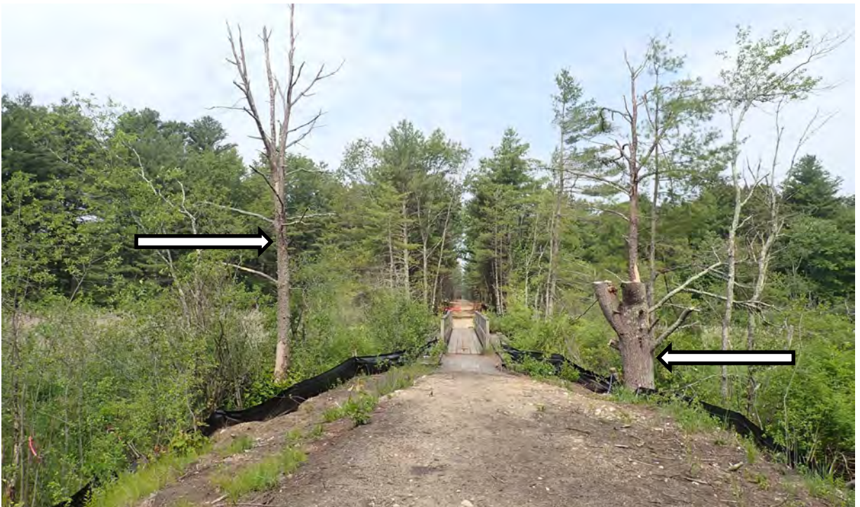
Photo #8: View of one snag that was left in place (left) in Impact Area 5, near the bridge crossing. Large pine (right) required removal to allow for bridge repairs. The stump of the pine was left in place. Facing west.
