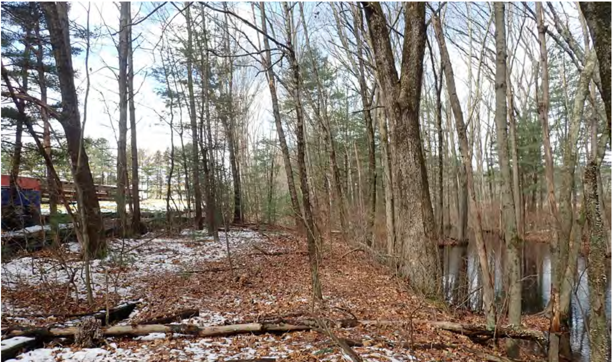
Photo #2: View of vernal pool #11 in Segment 11. No sediment or construction debris observed within the resource area or beyond the silt fencing. Silt fence is in good condition. Facing northwest.
