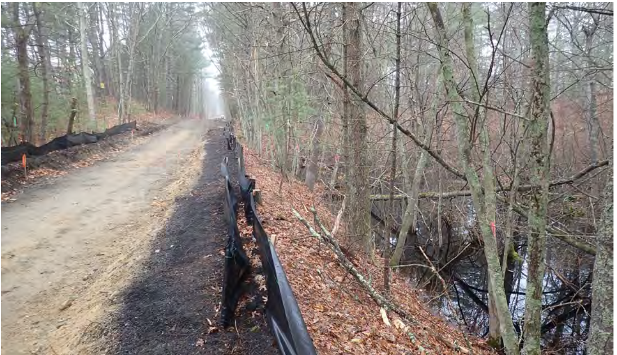
Photo #2: View of vernal pool #3 in Segment 8. No sediment or debris observed within the resource area or associated buffer zone. Silt fencing here and throughout the project area is in good condition. Facing northwest.
