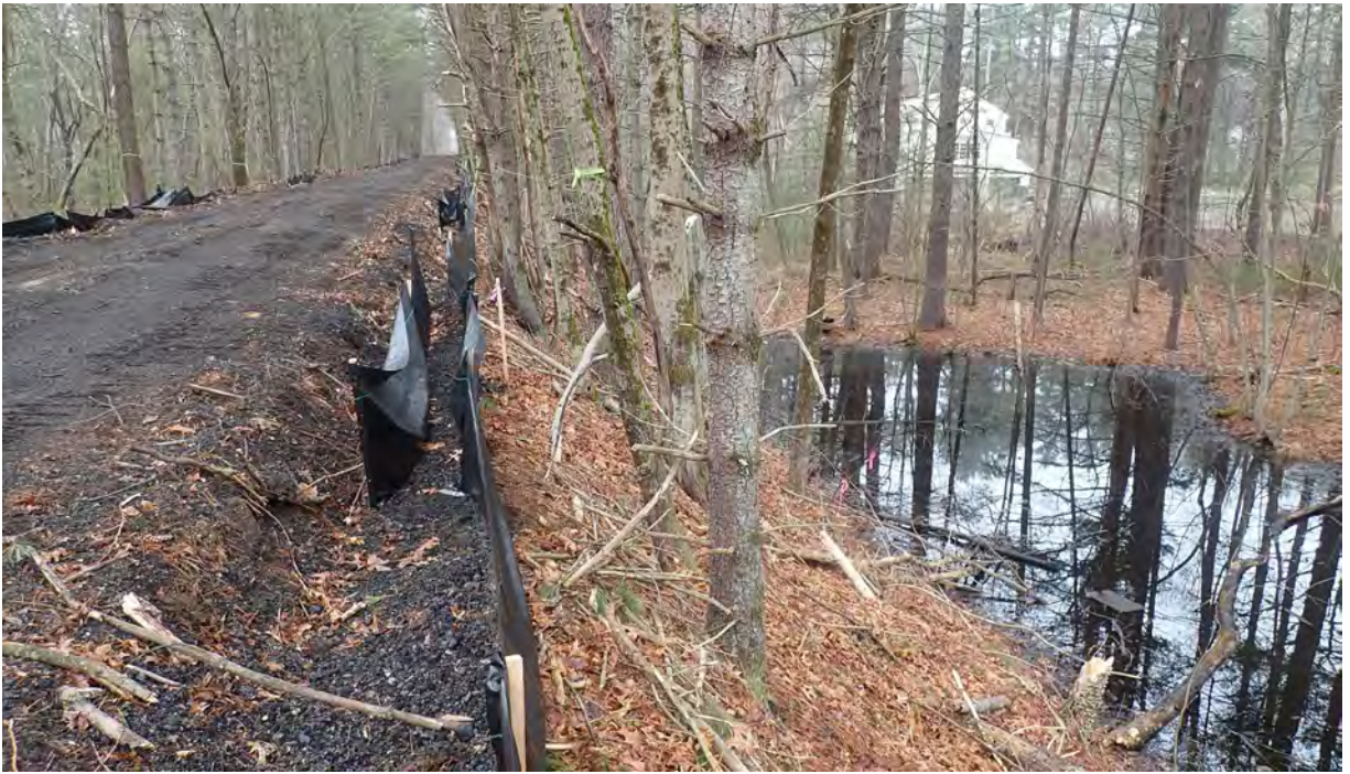
Photo #3: View of vernal pool #9 in Segment 10. Silt fence in good condition. No sediment or debris observed in the resource area or associated buffer zone. Facing northwest.
