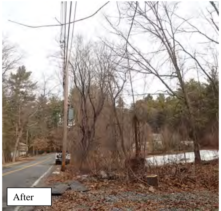
Photo #13: View of tree in Impact Area 9 on the eastern side of Peakham Road. Tree was located just beyond the limit of work and in poor condition. Tree branches and thick vines connected the tree extended into the limit of work and onto the power lines. For safety concerns the entire tree was removed and stump left in place. Facing northeast.
