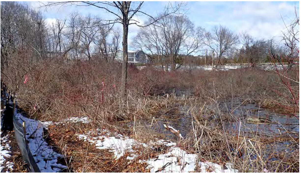
Photo #1: View of vernal pool #15 in Segment 14. Silt fence is in good condition here and throughout the project area. No sediment or debris observed within the resource area. Facing northwest.
