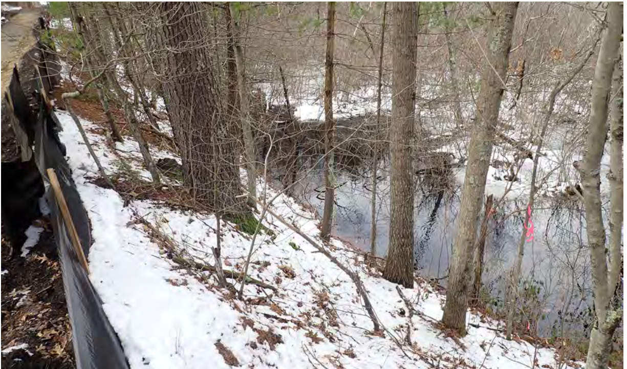
Photo #4: View of vernal pool #4 in Segment 8. Silt fence in good condition. No sediment or debris observed in the resource area or associated buffer zones. Facing northwest.
