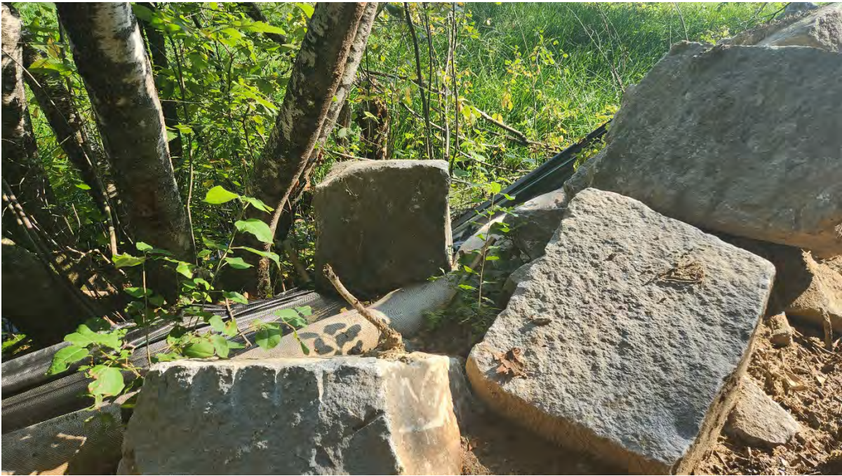
Photo 4: Boulder on the silt fence along segment 13. Photo taken on 9/06/23
