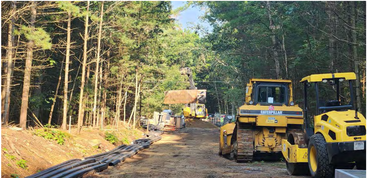
Photo 1: Manhole installation between segment 8 and segment 9. Photo taken on 9/06/23
