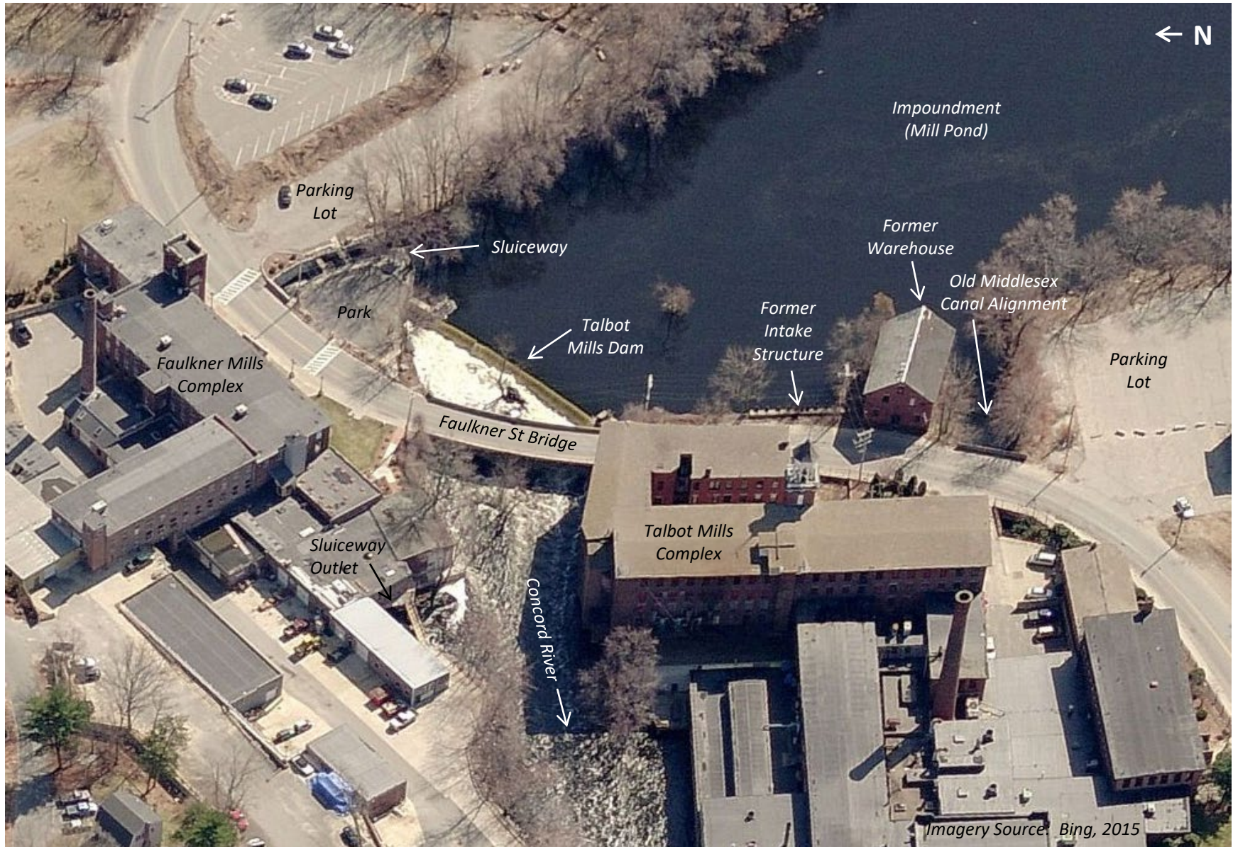
Figure 3-3: Aerial View of Talbot Mills Dam
