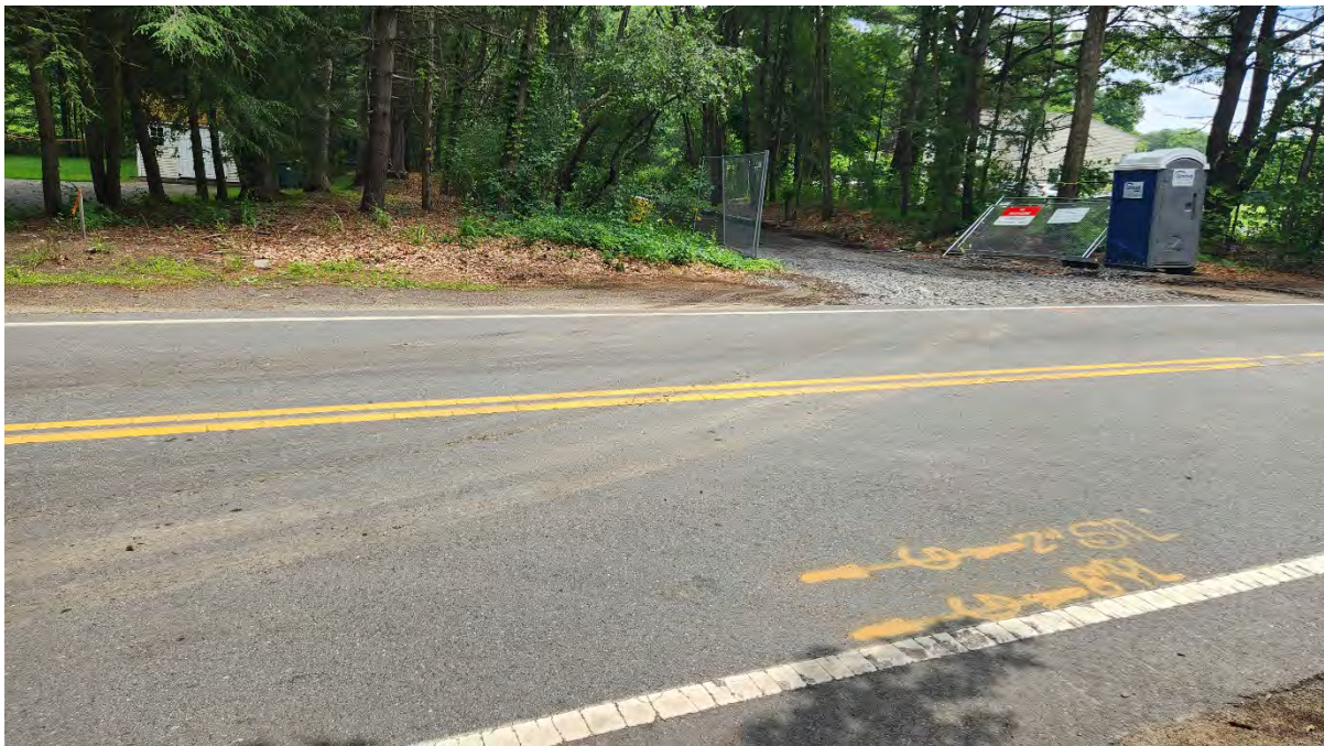
Photo 1: Sediment in road from construction entrance STA 361+00. Photo taken on 6/26/23
