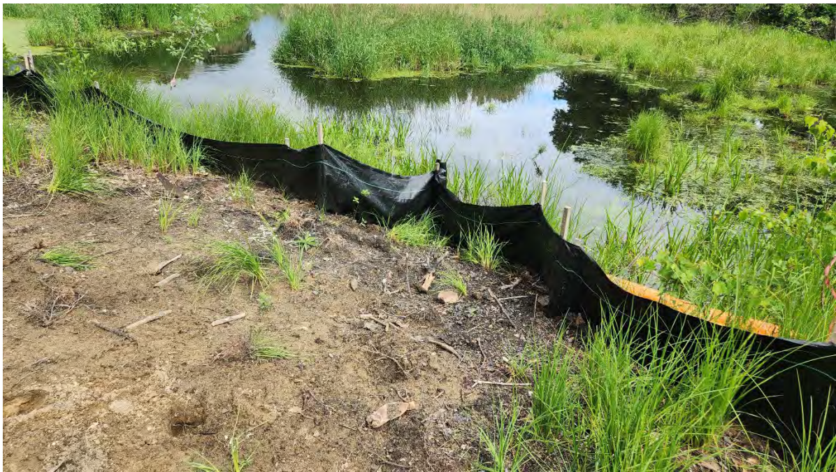
Photo 1: Silt fence and filter tube functioning properly along segment 14 near Hop Brook Bridge. Photo taken on 6/15/23
