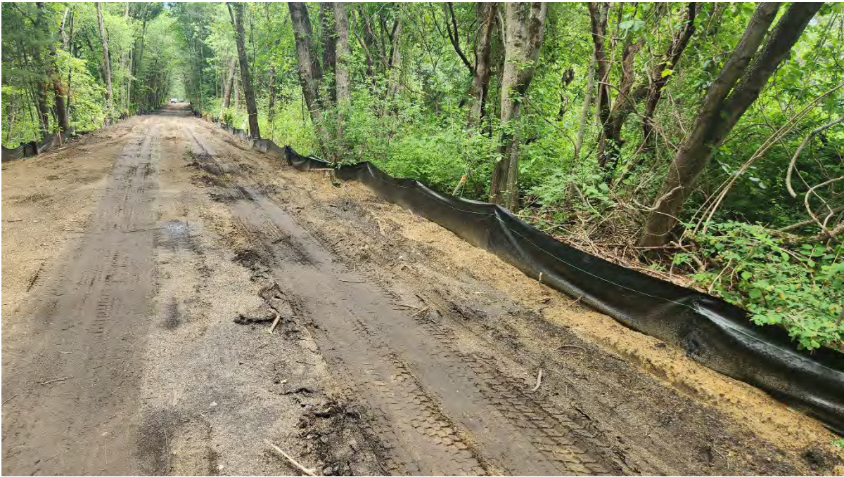
Photo 6: Silt fence functioning properly along segment 11. Photo taken on 6/15/23
