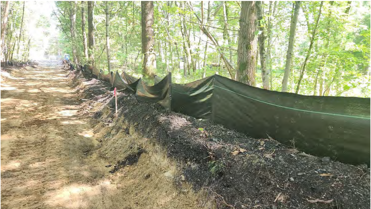
Photo 8: Silt fence functioning properly along segment 9. Photo taken on 6/15/23
