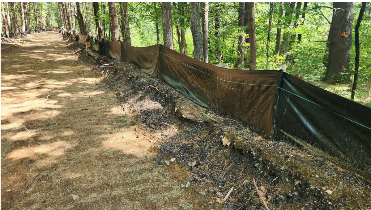
Photo 7: Silt fence functioning properly along segment 10. Photo taken on 6/15/23
