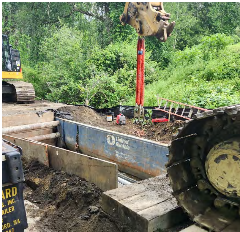
Photo 3: Manhole being installed along segment 14. Photo taken on 6/15/23
