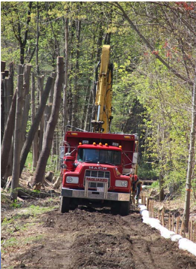
BFRT at Hudson Road After Railroad Tie Removal
