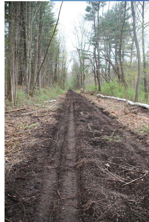
BFRT at Hudson Road After Railroad Tie Removal
