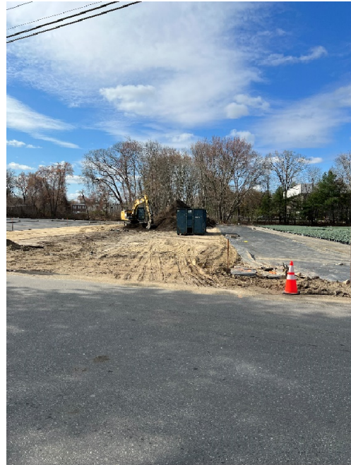
Photo 2: Sta. 116+00 looking south, standing at Codjer Lane.
