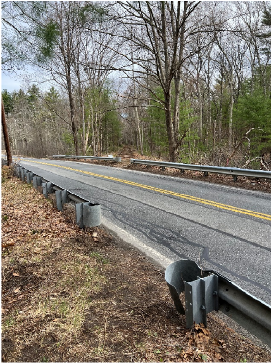
Photo 13: Sta 284+00 looking north towards Pantry Road
