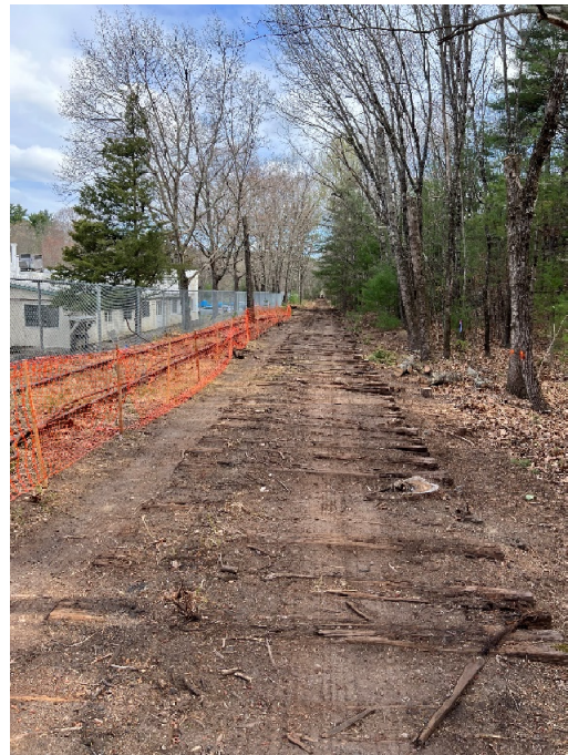
Photo 12: Sta. 176+00 looking north, standing near Hudson Road
