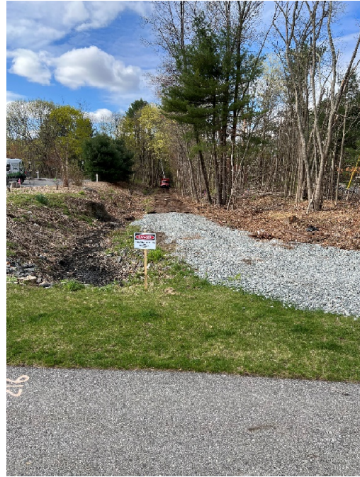
Photo 6: Sta. 175+00 looking south, standing at Hudson Road
