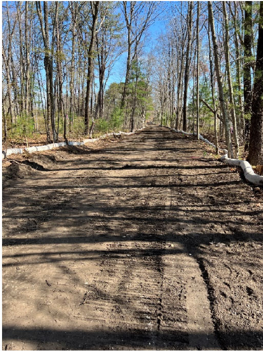
Photo 1: Sta. 101+00 looking north
