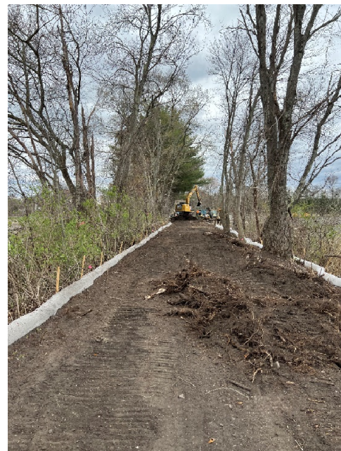
Photo 4: Sta. 118+00 looking south towards Codjer Lane
