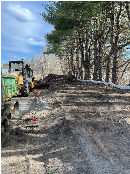
Photo 11: Sta. 116+00 looking north, standing at Codjer Lane
