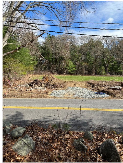
Photo 8: Sta. 215+00 looking north, standing at Morse Road
