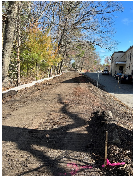
Photo 10: Sta. 106+50 looking north towards the 71 Union Avenue driveway
