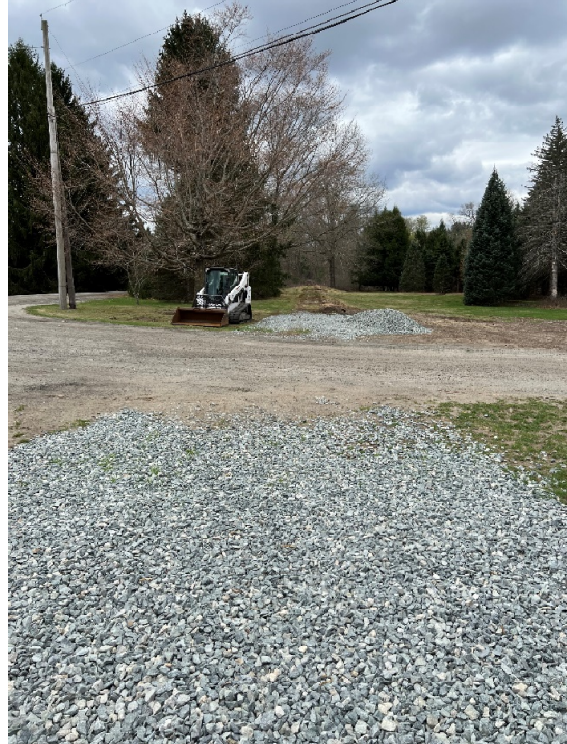
Photo 14: Sta. 321+00 looking south towards Fairview Farms driveway
