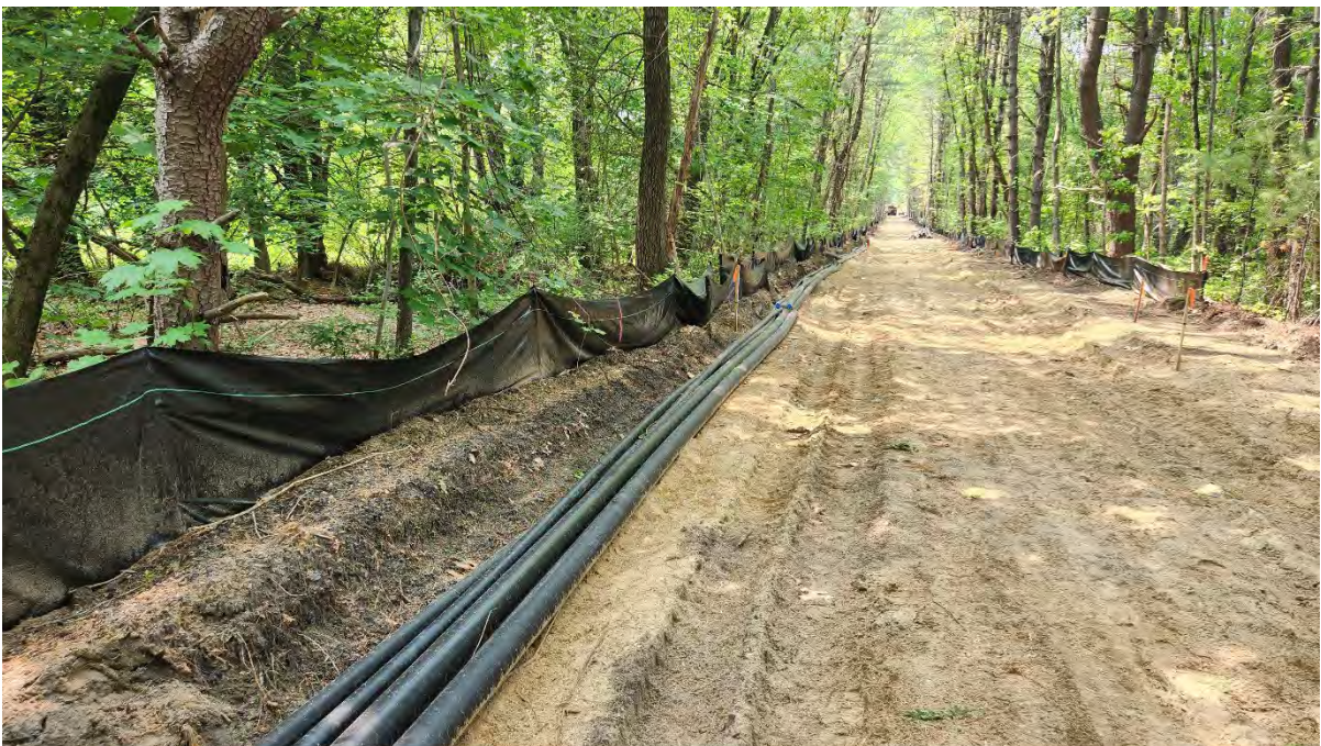
Photo 5: Silt fence functioning properly along segment 11. Photo taken on 5/24/23
