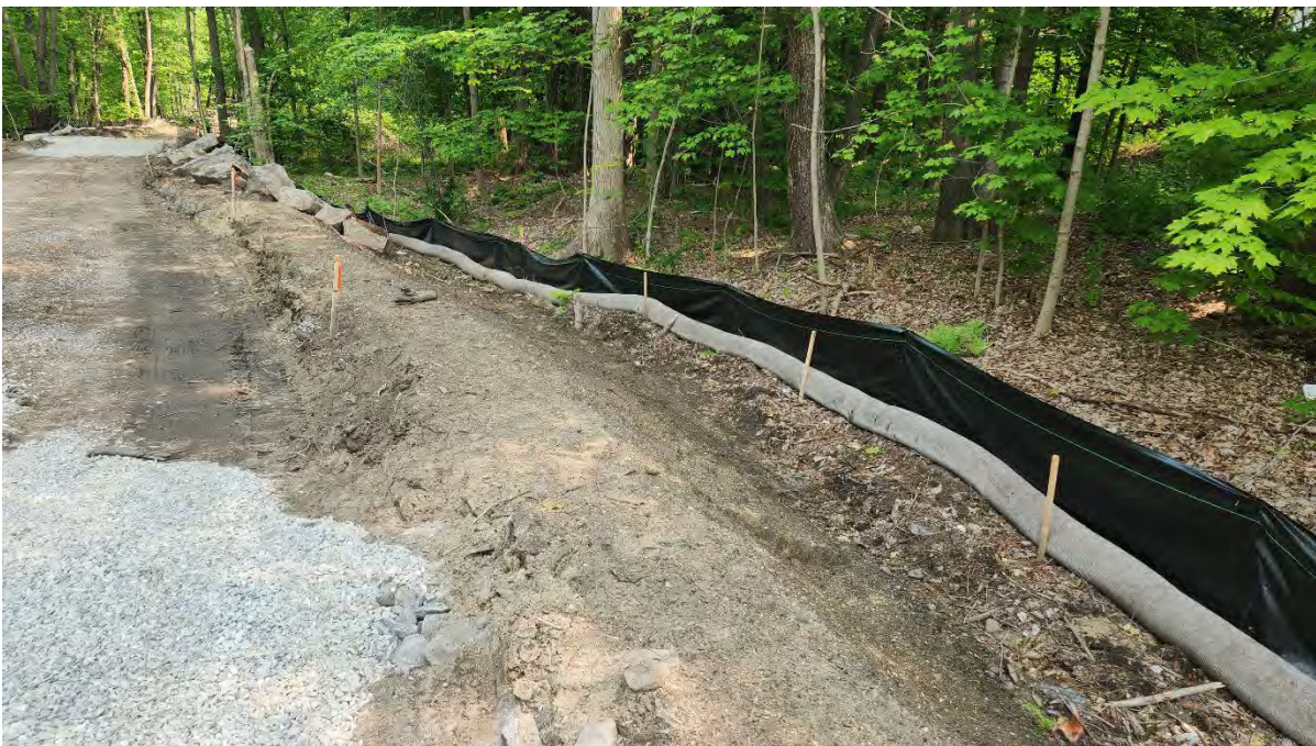
Photo 9: Silt fence functioning properly along segment 8. Photo taken on 5/24/23
