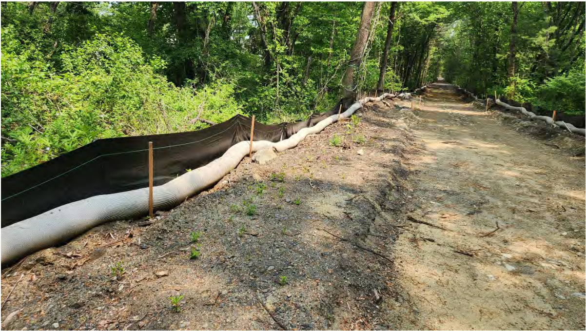
Photo 4: Silt fence functioning properly along segment 12. Photo taken on 5/24/23
