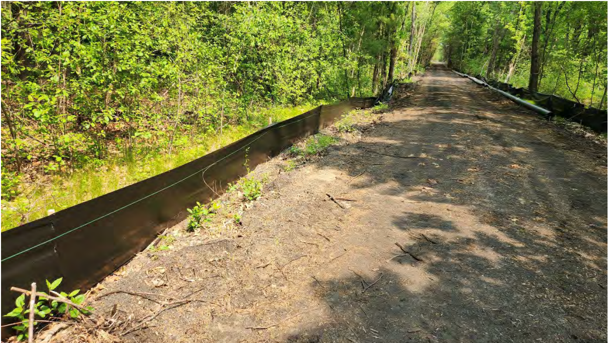
Photo 6: Silt fence functioning properly along segment 10. Photo taken on 5/24/23
