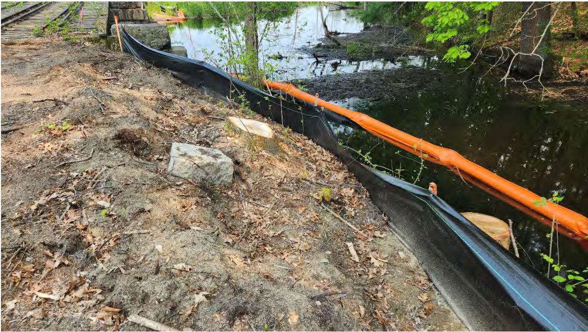
Photo 10: Silt fence functioning properly along segment 7. Photo taken on 5/24/23
