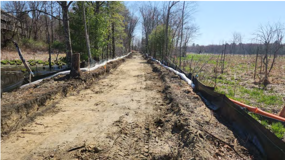
Photo 1: Silt fence and filter tube functioning properly along segment 14. Photo taken on 4/20/23
