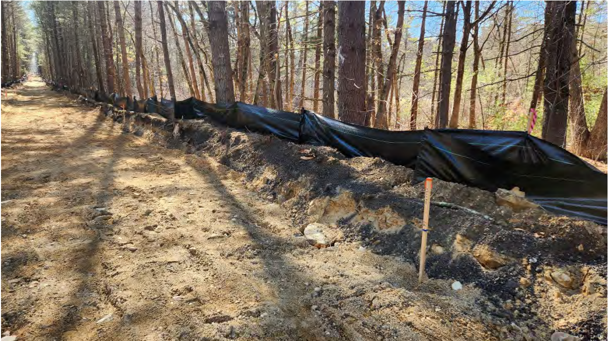
Photo 6: Silt fence functioning properly along segment 10. Photo taken on 3/30/23
