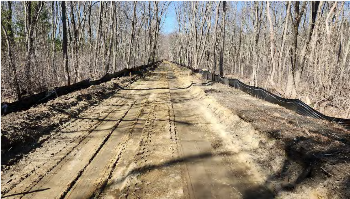
Photo 1: Silt fence functioning properly along segment 14. Photo taken on 3/30/23
