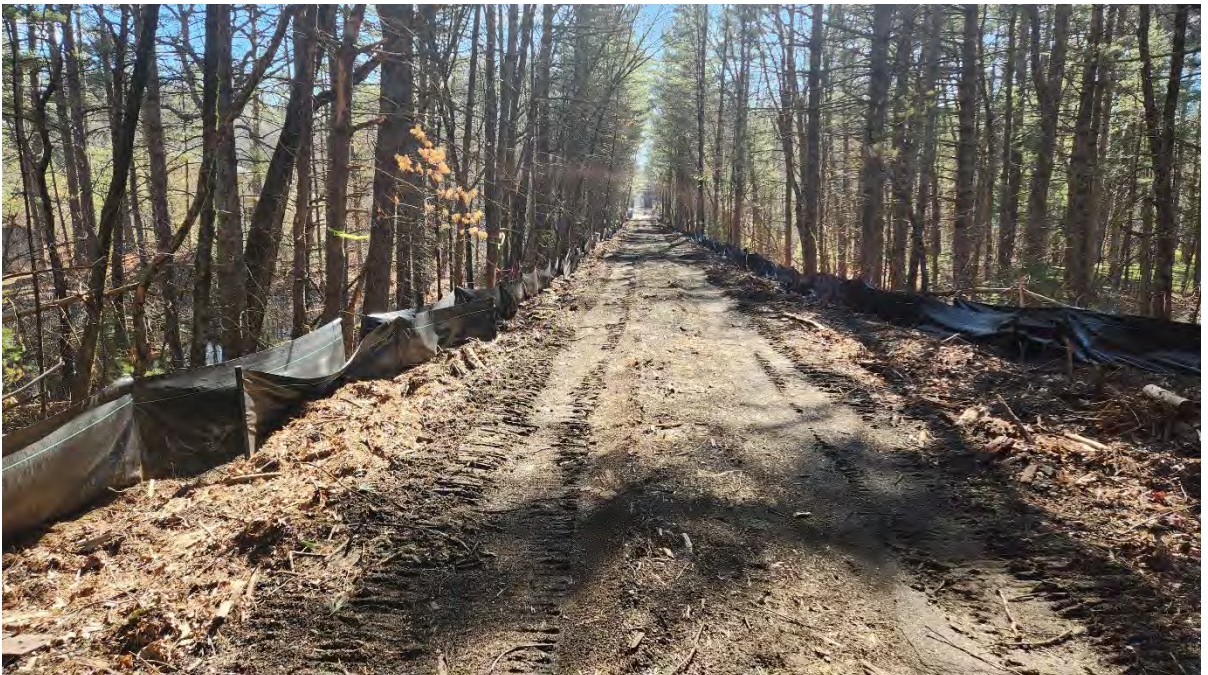
Photo 7: Silt fence functioning properly along segment 9. Photo taken on 3/30/23
