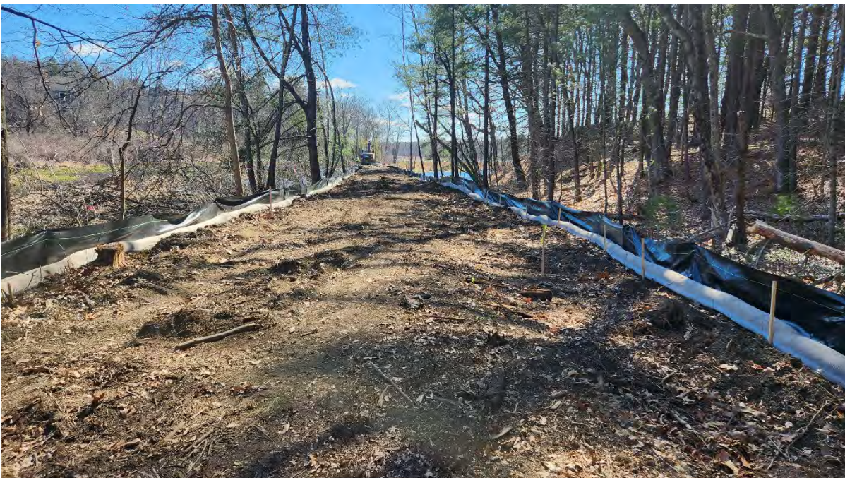
Photo 3: Silt fence and filter tubes functioning properly along segment 13.
