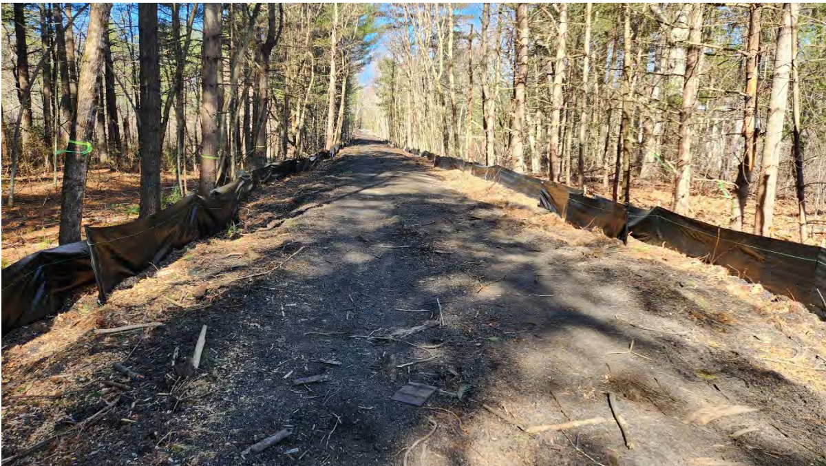
Photo 5: Silt fence functioning properly along segment 11. Photo taken on 3/30/23
