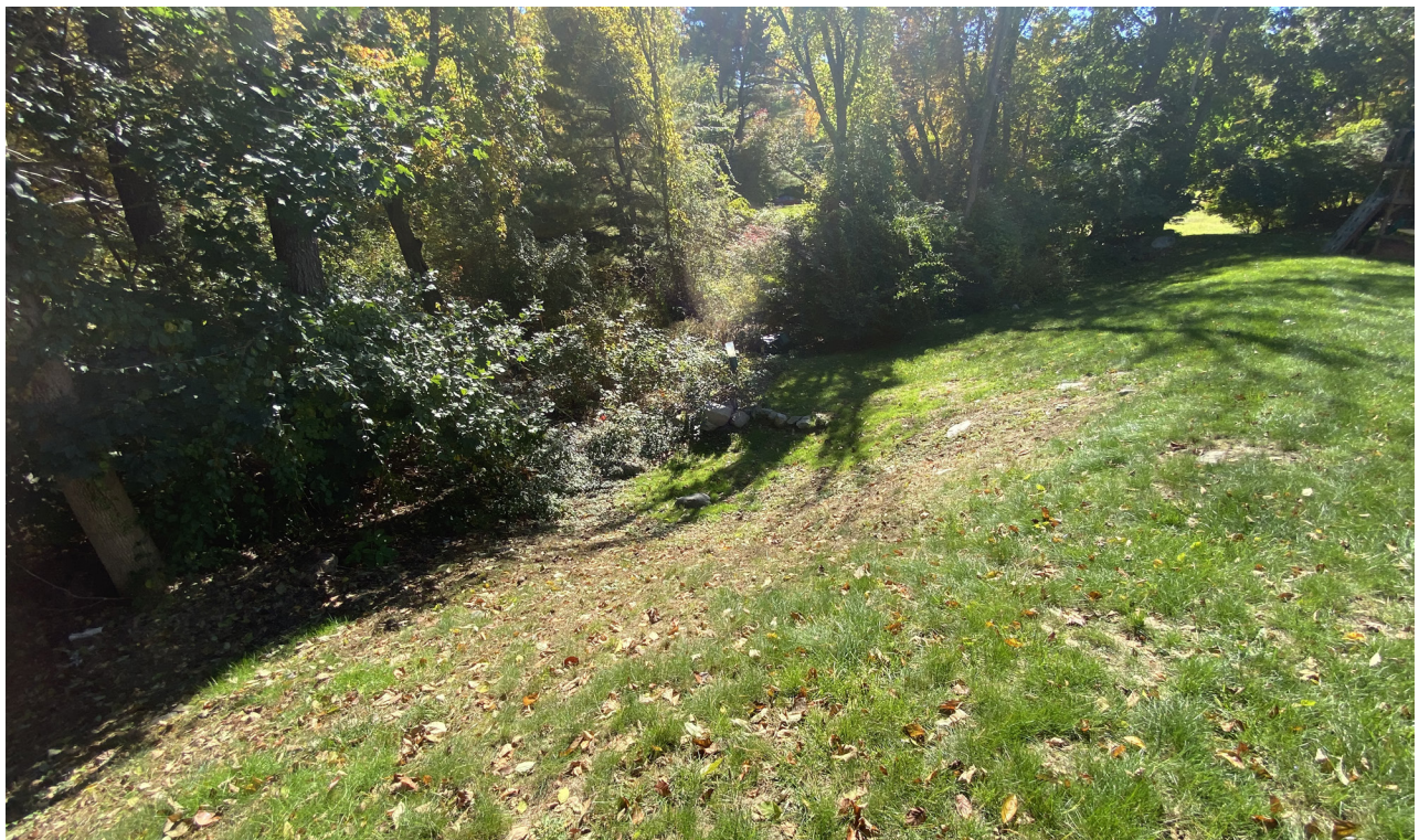
REAR SLOPE, WATER RETENTION AREA, AND WELAND (SOUTH) - FALL 2022
