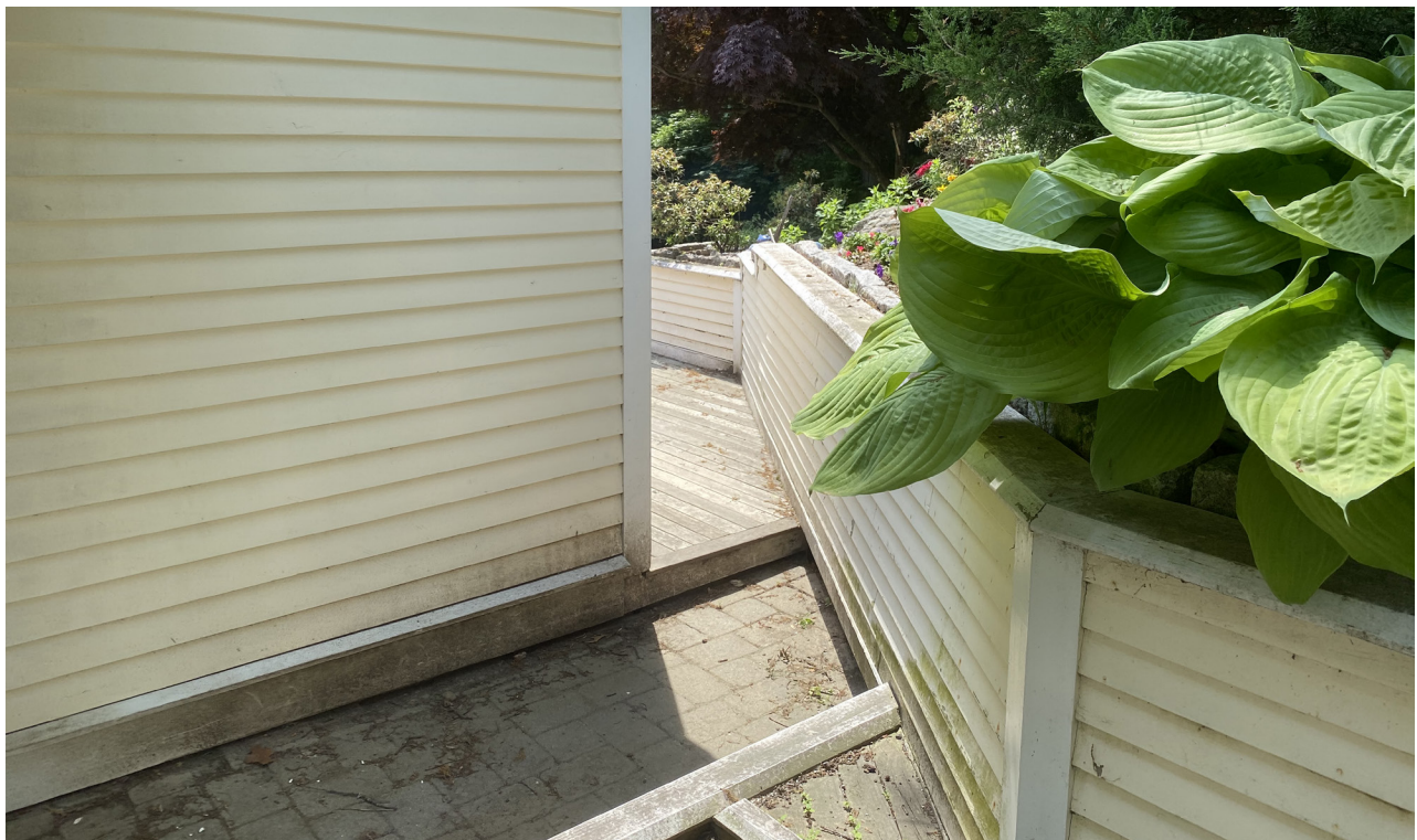
TIMBER RETAINING WALL AT HOUSE CORNER (WEST) - SPRING 2022
