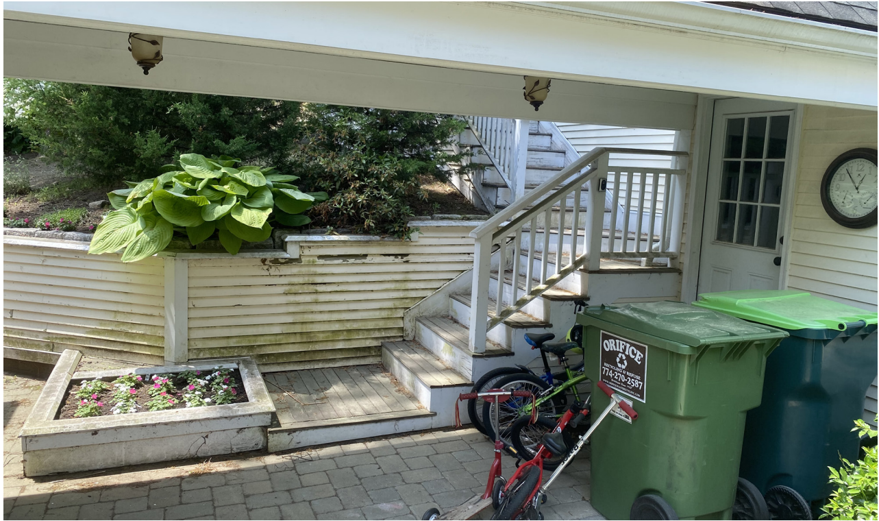
HOUSE/GARAGE CONNECTOR & STAIRS TO GARAGE DECK (WEST) - SPRING 2022
