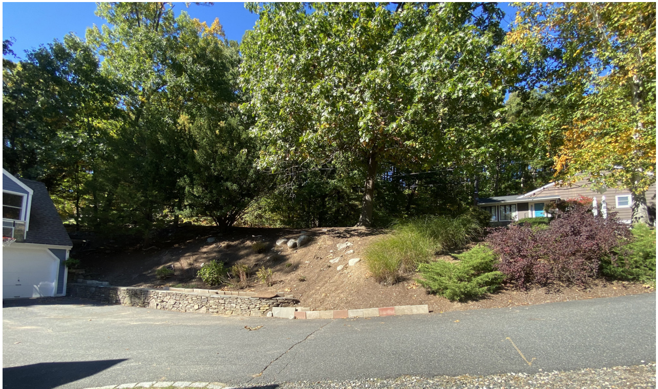
FRONT SLOPE (NORTH) - FALL 2022
