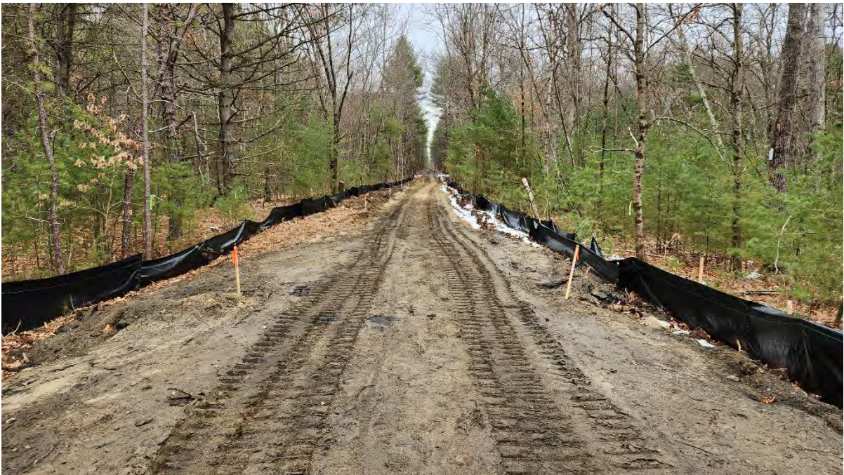
Photo 9: Silt fence operating properly along segment 7. Photo taken on 3/14/23
