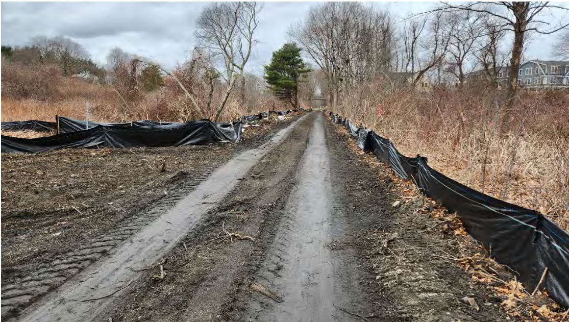
Photo 1: Silt fence operating properly along segment 14.
