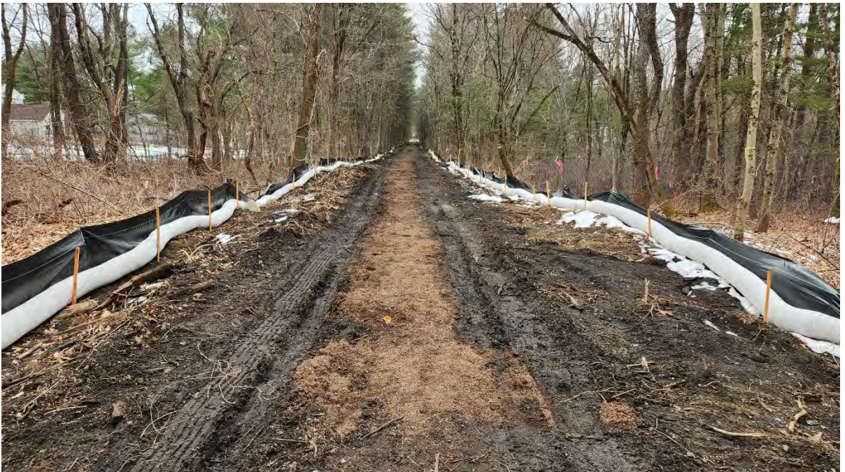
Photo 7: Silt fence and filter tube installed and operating properly along segment 9.
