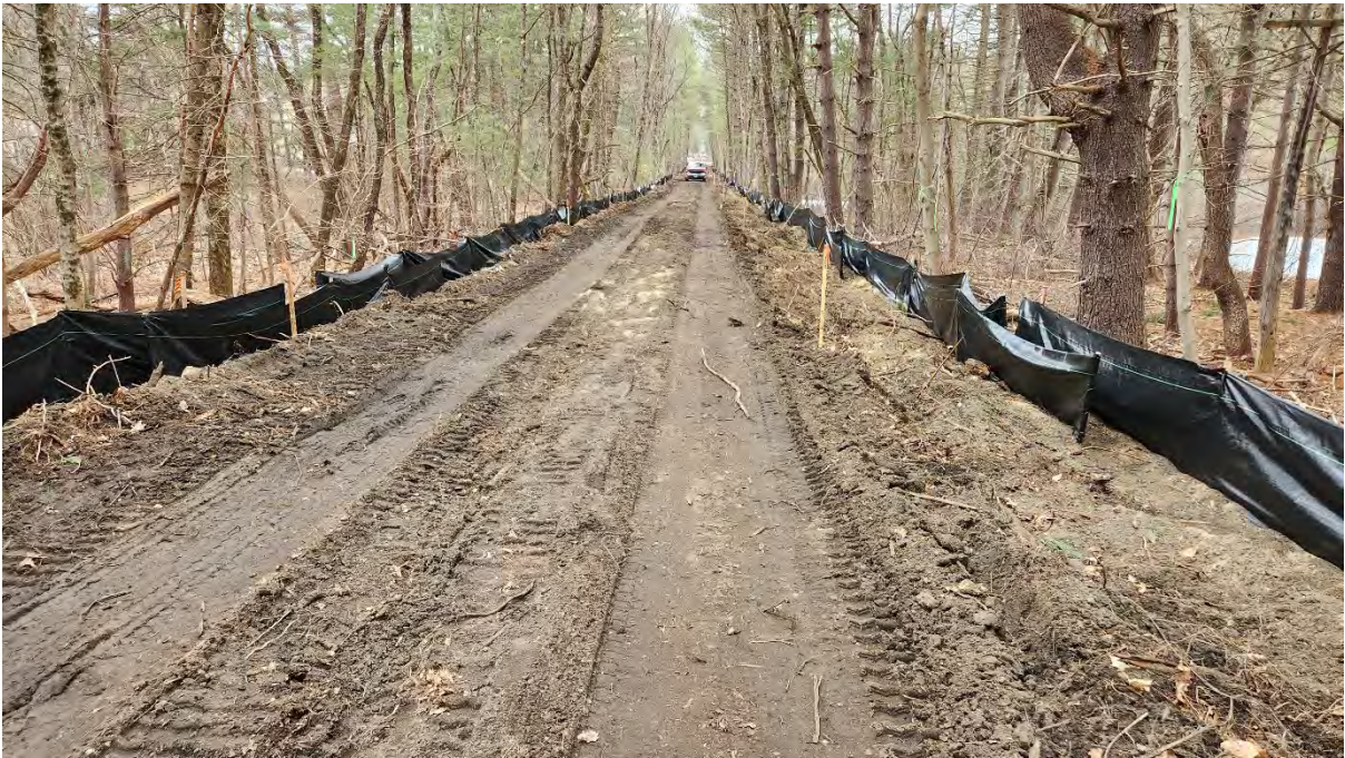
Photo 6: Silt fence operating properly along segment 10.
