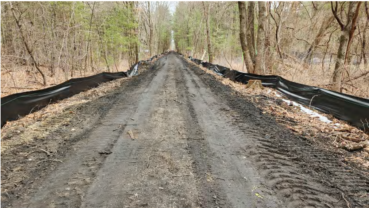
Photo 5: Silt fence operating properly along segment 11. Photo taken on 3/14/23
