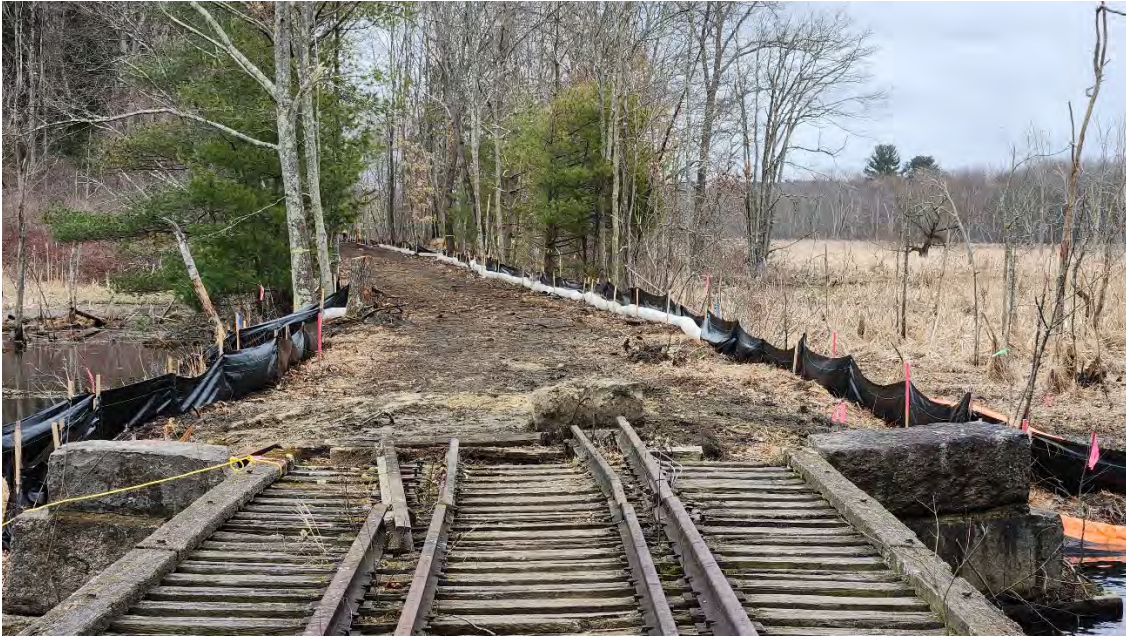
Photo 2: Turbidity curtain, filter tubes, and silt fence installed and operating properly at bridge 127.
