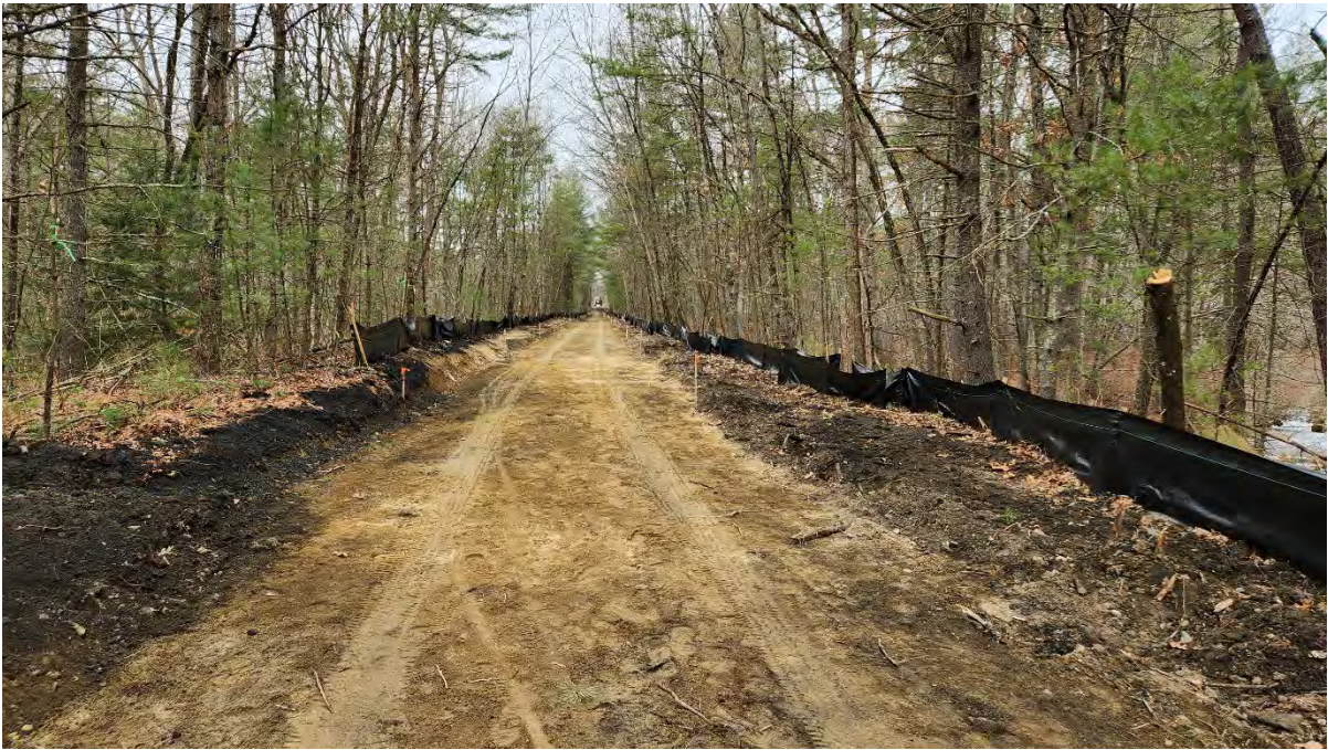
Photo 8: Silt fence operating properly along segment 8. Photo taken on 3/14/23
