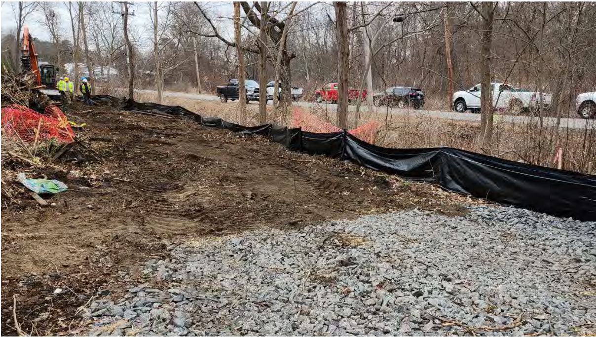
Photo 4: Silt fence operating properly along segment 12 while construction occurs. Photo taken on 3/14/23
