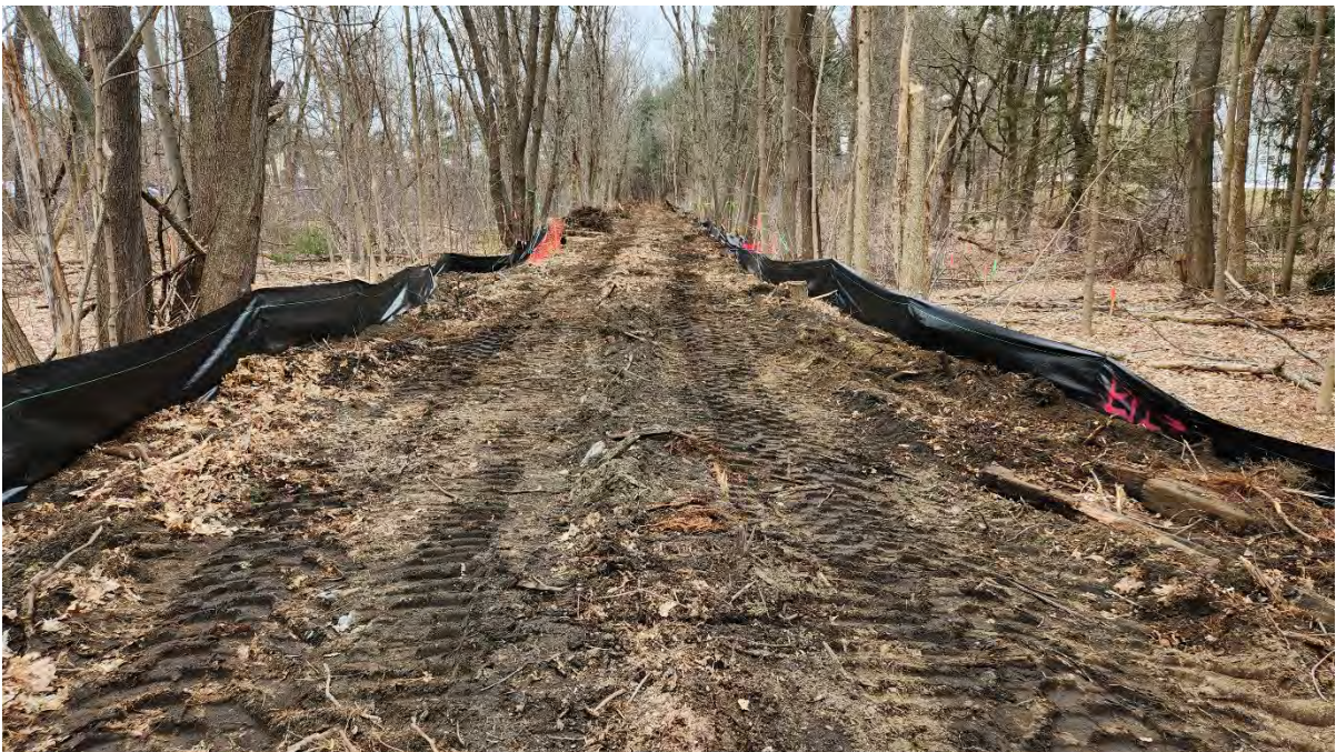
Photo 3: Silt fence operating properly along segment 13.
